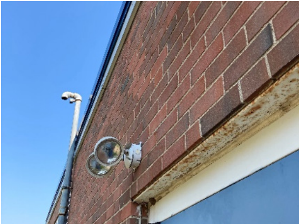
Exterior Door Remote Heads
