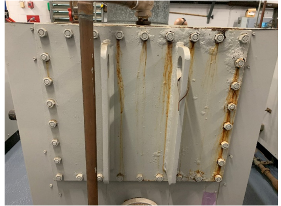
Boiler Condition (Typ 3)
