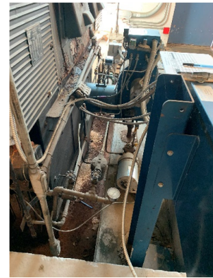
Boiler Installed in Pit
