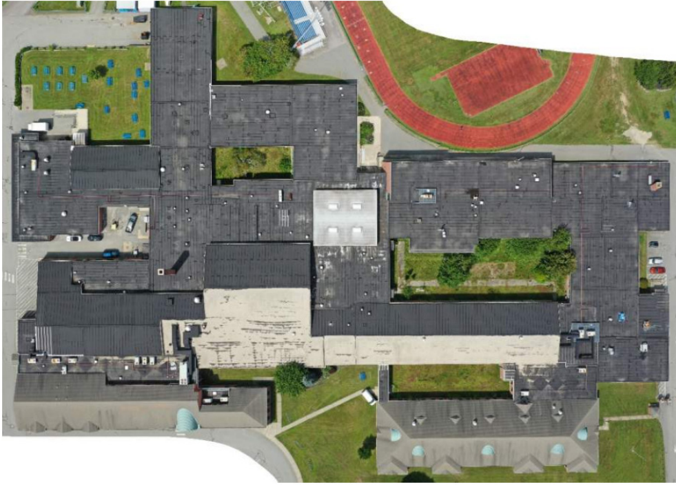
Overall aerial photo of Barrington High School at 220 Lincoln Avenue taken by Odeh Engineers with a drone. North is oriented upwards on the page
