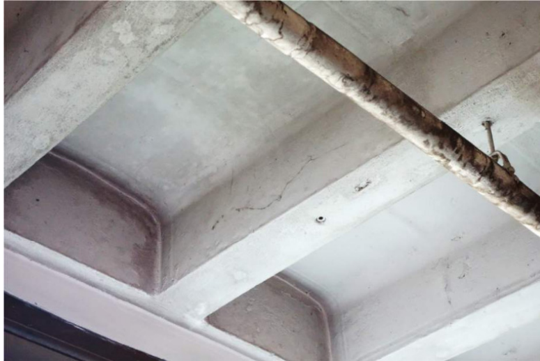
Photo of concrete double tee floor framing in boiler room.
