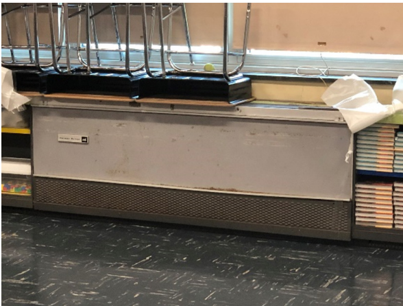
Typical Unit Ventilator
