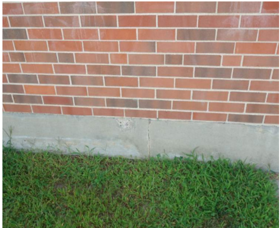
Photo of typical cast-in-place concrete foundation wall
