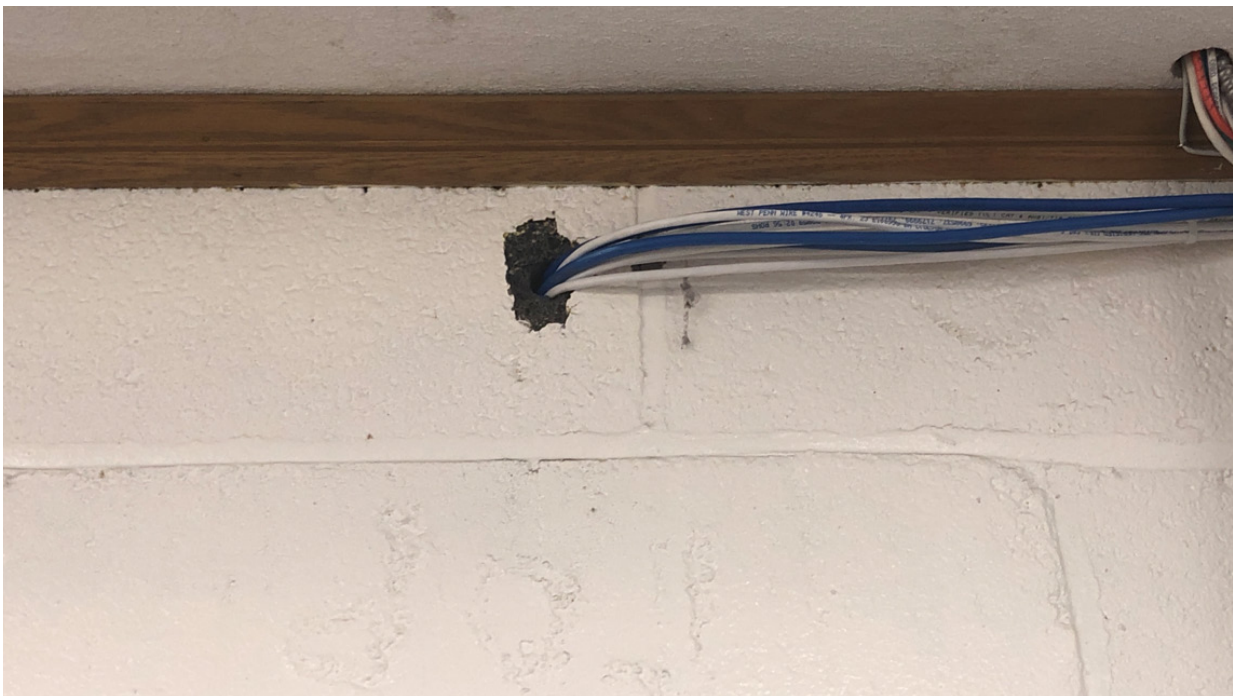
Photo of non-firestopped sleeve in MDF
