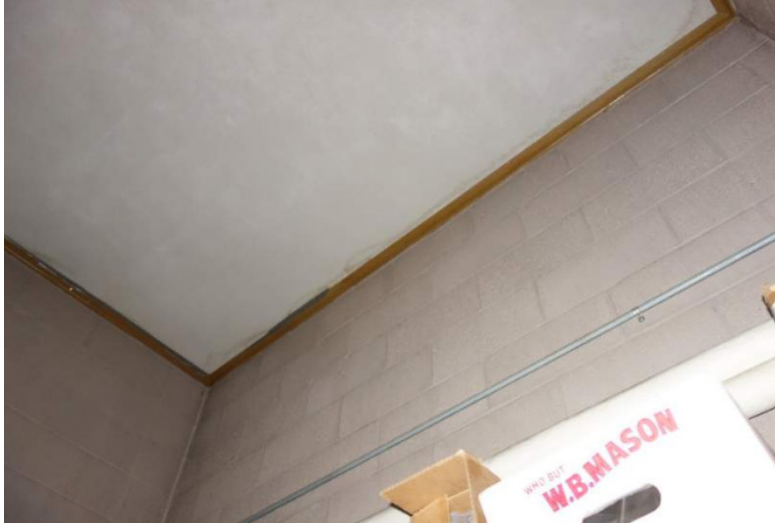
Photo showing typical interior cmu wall.
