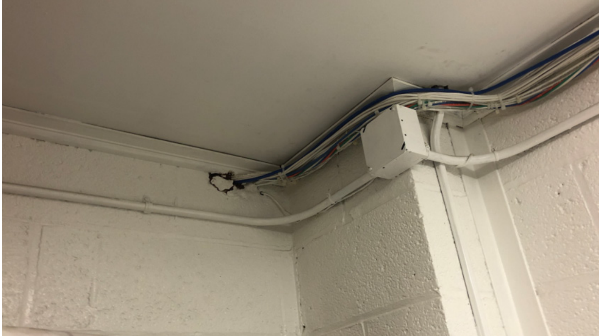
Photo of non-firestopped sleeve in MDF
