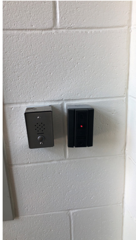
Picture of communication device and card reader
