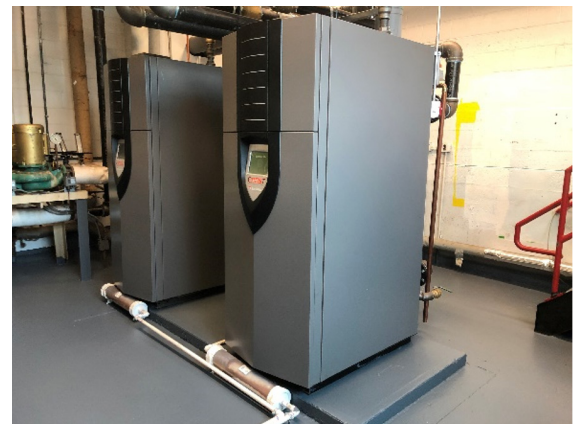
Condensing Boiler
