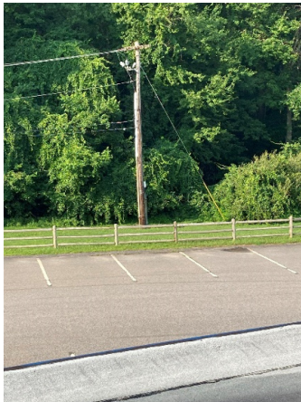
Service Riser Pole
