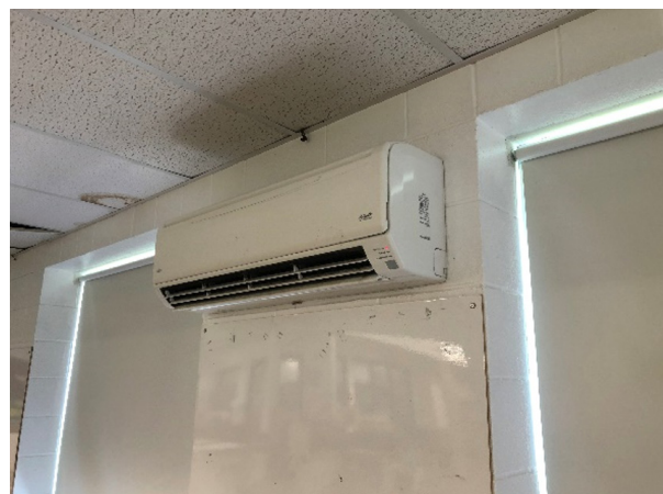
Ductless Cooling Units
