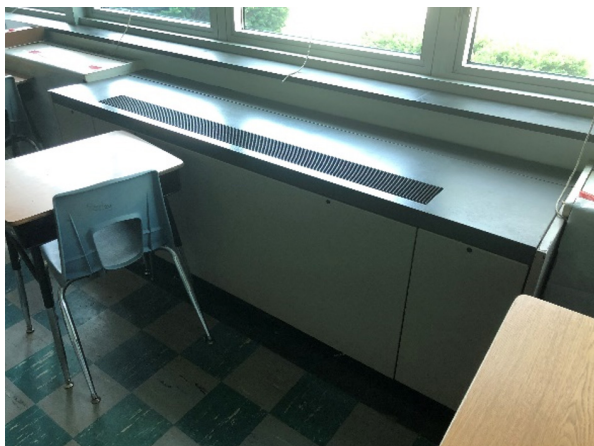
Typical Unit Ventilator
