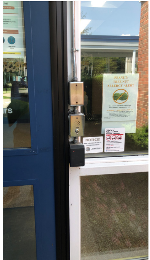
Photo of communication device and card reader
