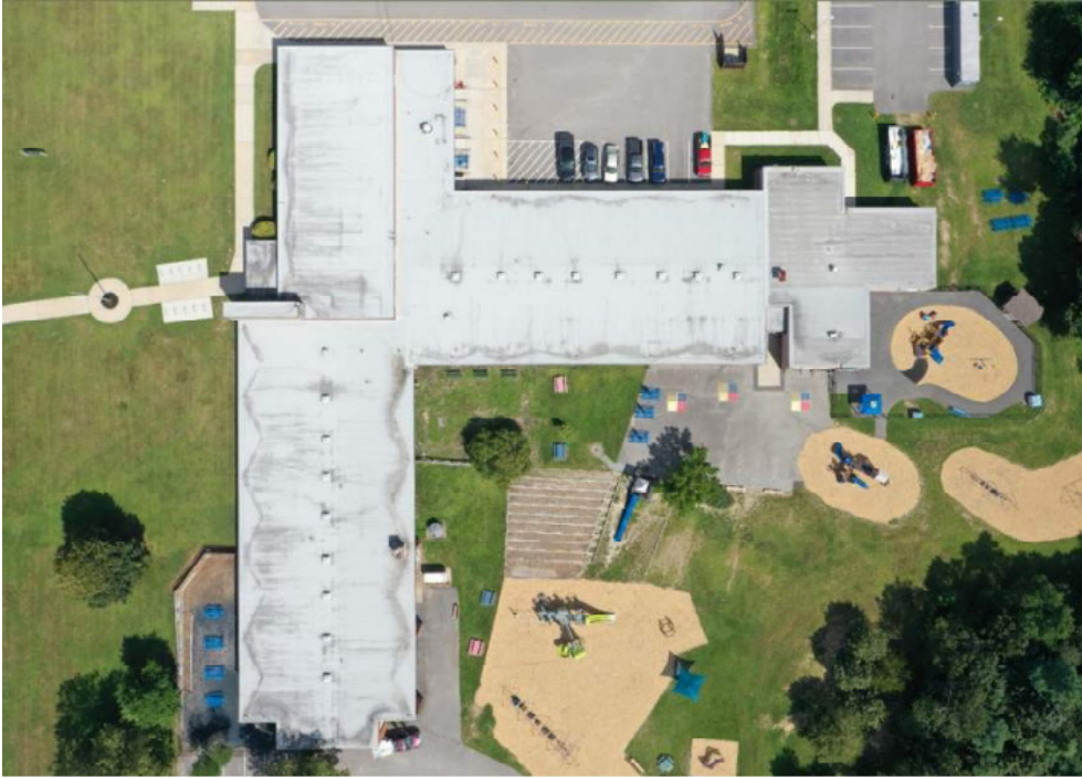
Overall aerial photo of the Primrose Hill Elementary School at 60 Middle Highway taken by Odeh Engineers with a drone. North is oriented upward on the page.
