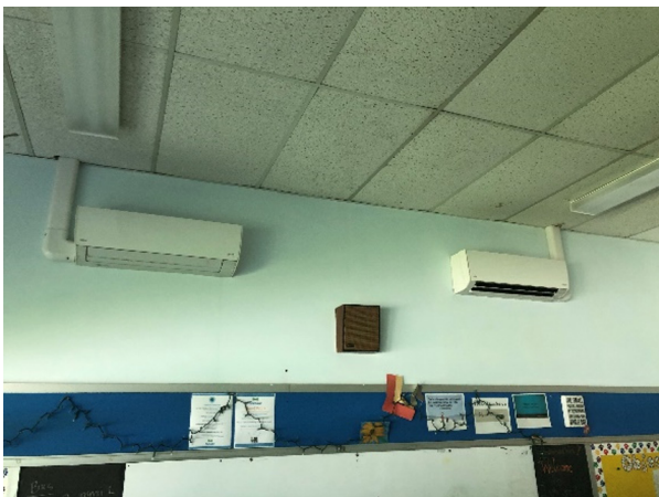
Ductless Cooling Units
