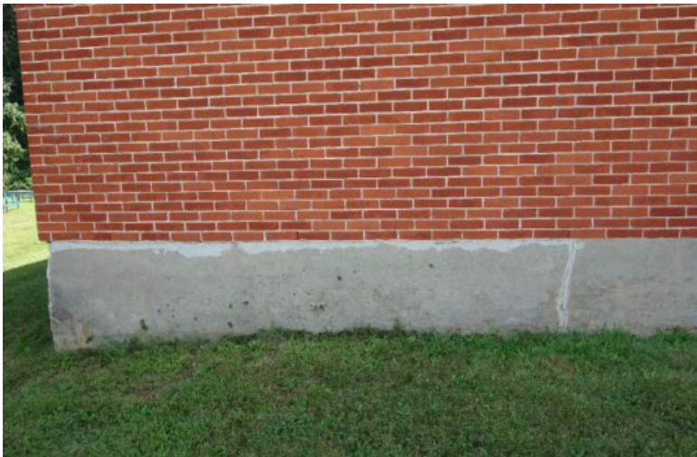
Photo showing the typical exterior brick veneer.
