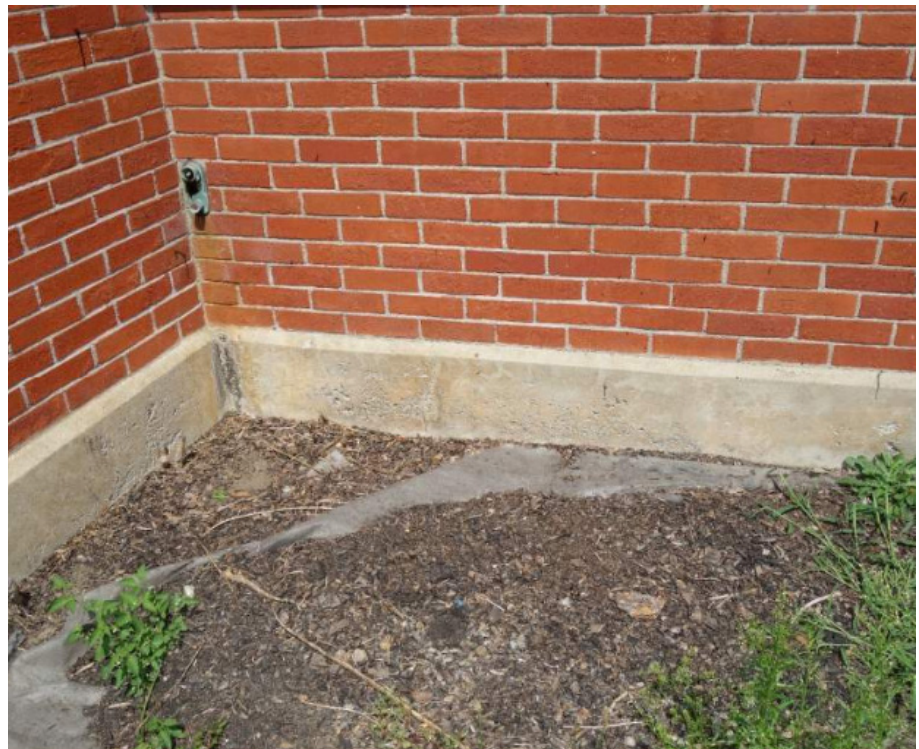
Photo of typical cast-in-place concrete foundation wall
