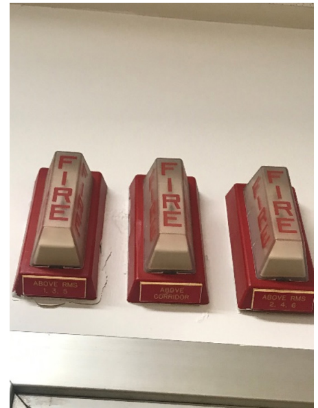
Above Ceiling Heat Detector Indicators
