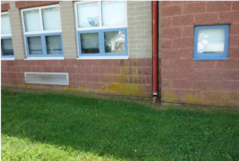
Photo showing typical exterior cmu.
