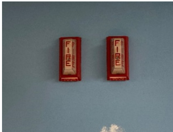
Above Ceiling Heat Detector Indicators
