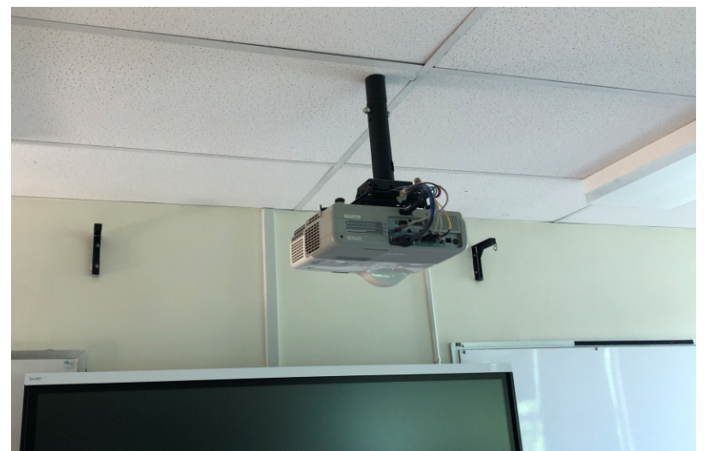
Photo of ceiling mounted projector.
