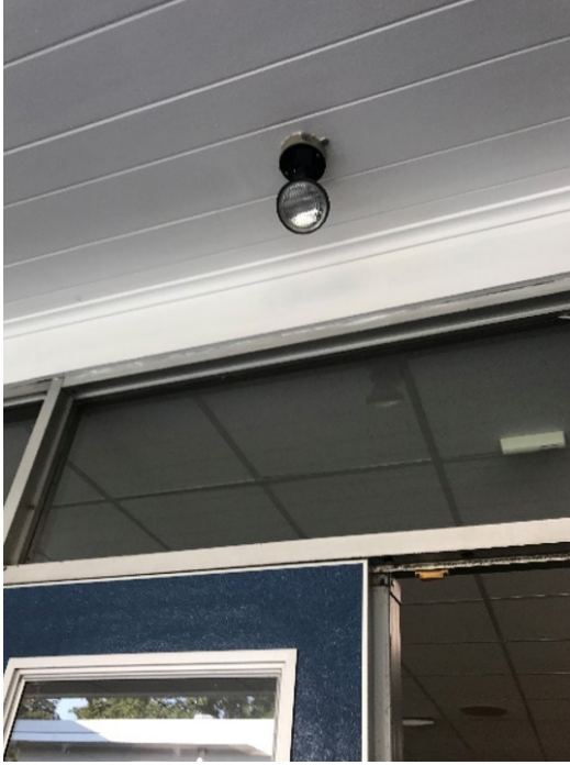
Exterior Door Remote Head
