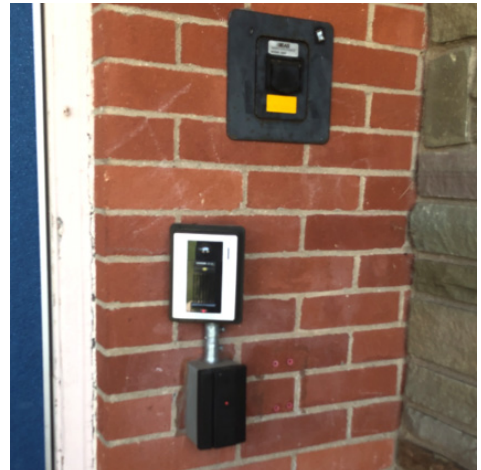
Picture of communication device and card reader
