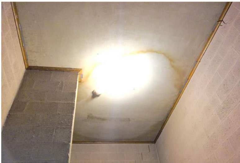
Photo of the typical hard ceiling at Nayatt Elementary School.
