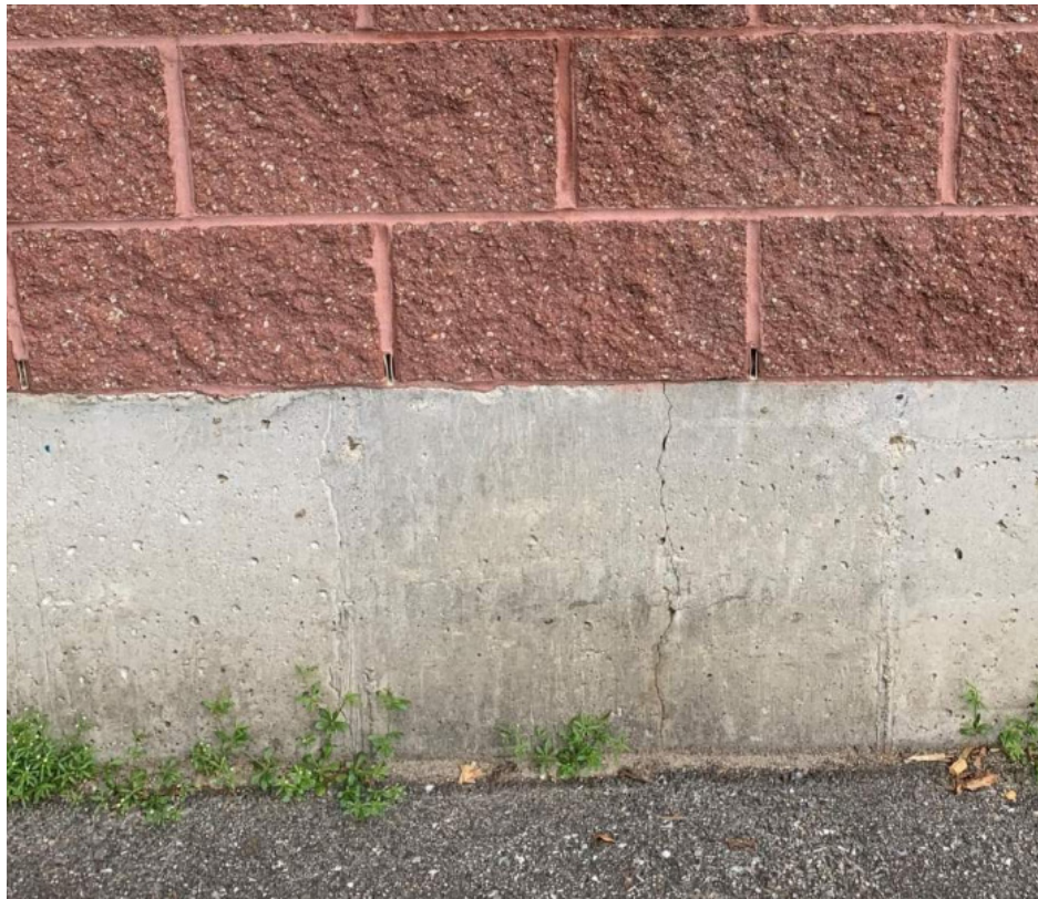
Photo of typical cast-in-place concrete foundation wall
