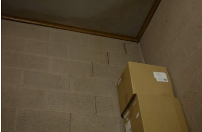
Photo showing the typical interior cmu wall
