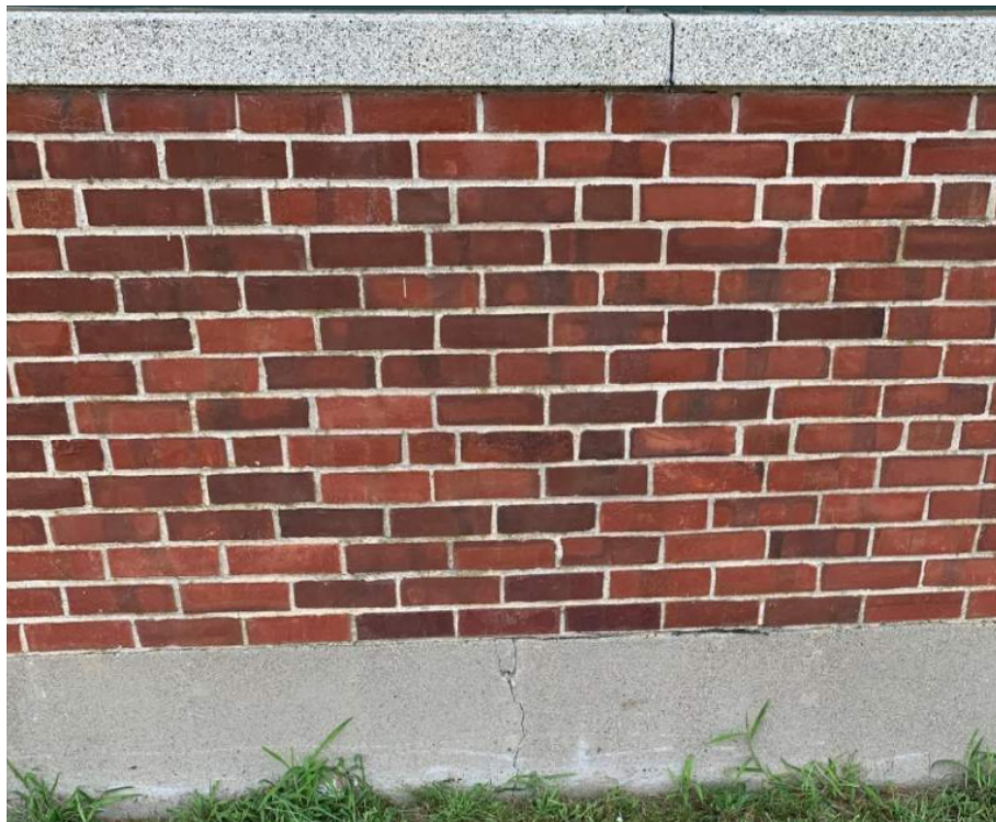
Photo of typical cast-in-place concrete foundation wall
