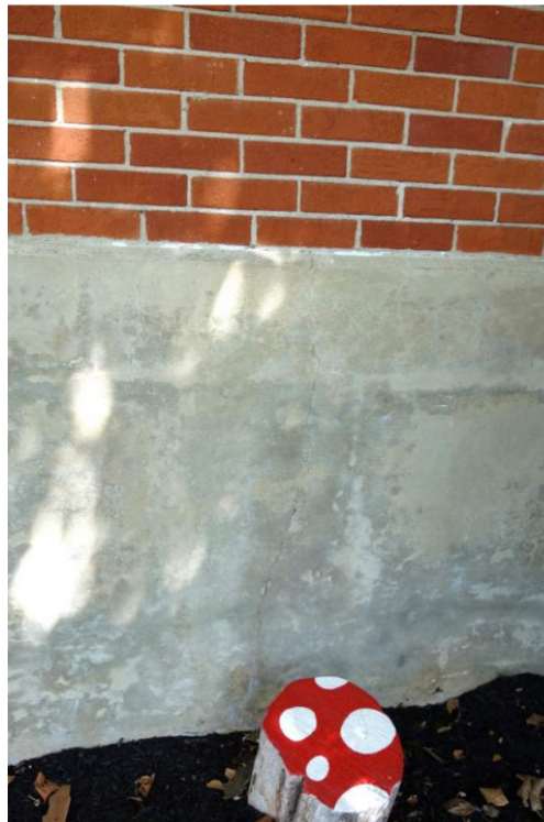
Photo of typical cast-in-place concrete foundation wall
