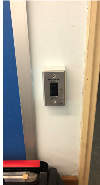
Photo of typical call switch below
