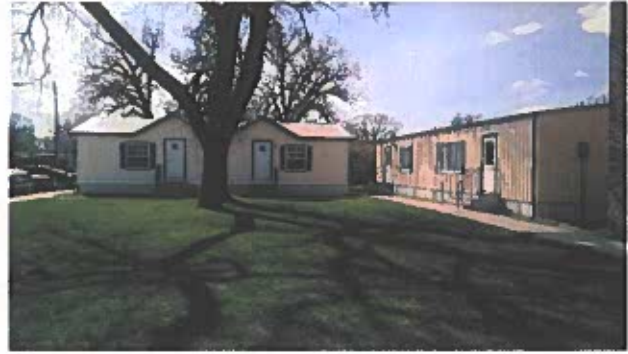
Stair access only to both portable buildings
