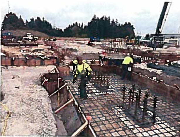
Incredibly large footings
