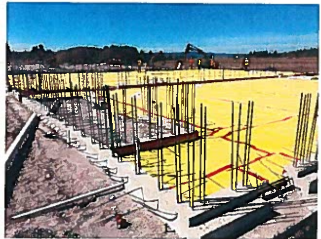
Vapor barrier under the wrestling / MP room
