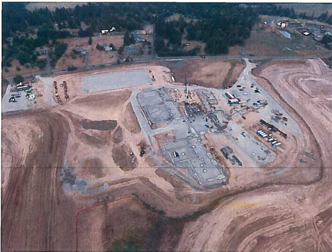
9-8: Drone photo of site looking east.
