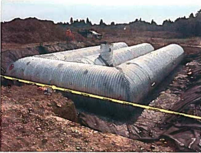
Massive underground storm water control under north parking lot
