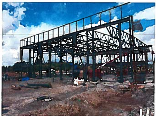
9-19: Steel after 10 work days
