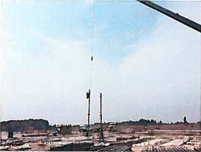
9-7: First steel in the air
