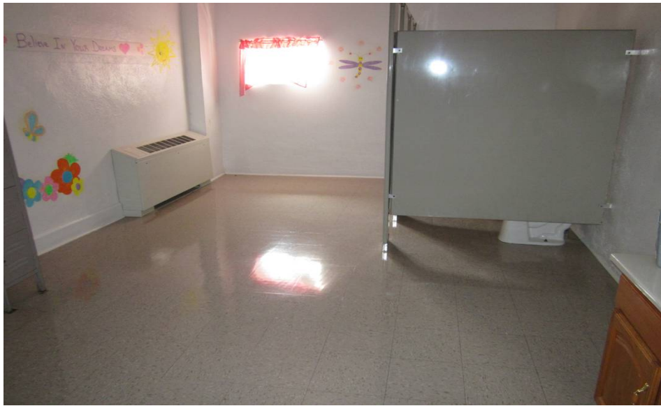
Photo 44 Location: Inside High School Date: 08/06/2013 Looking inside one of the restrooms
