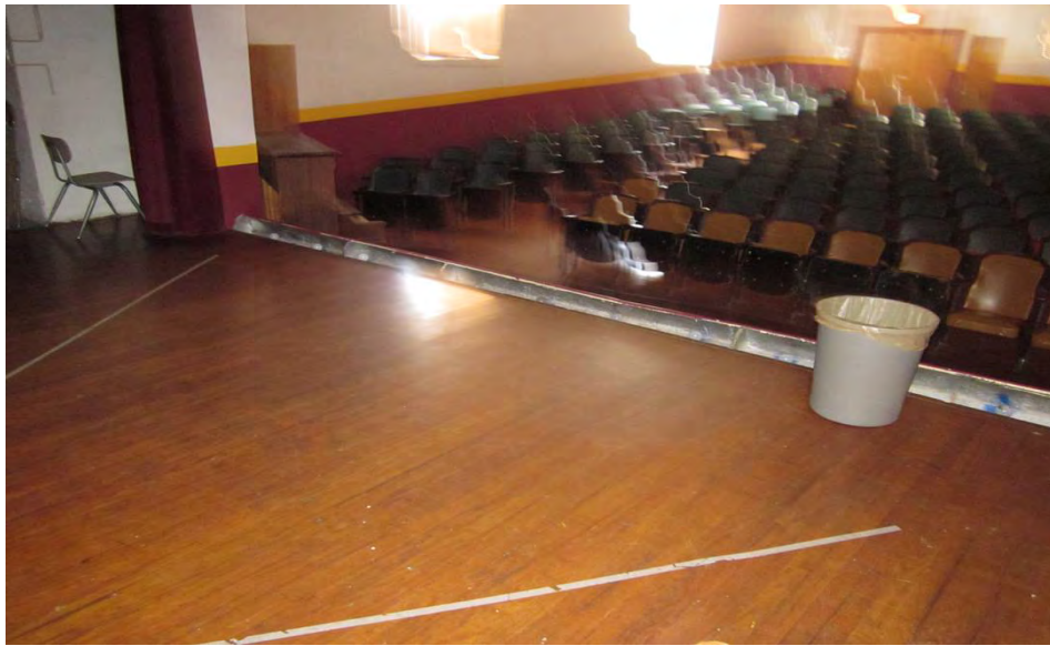
Photo 4 Location: Inside Elementary School Date: 08/06/2013 Looking inside of the auditorium
