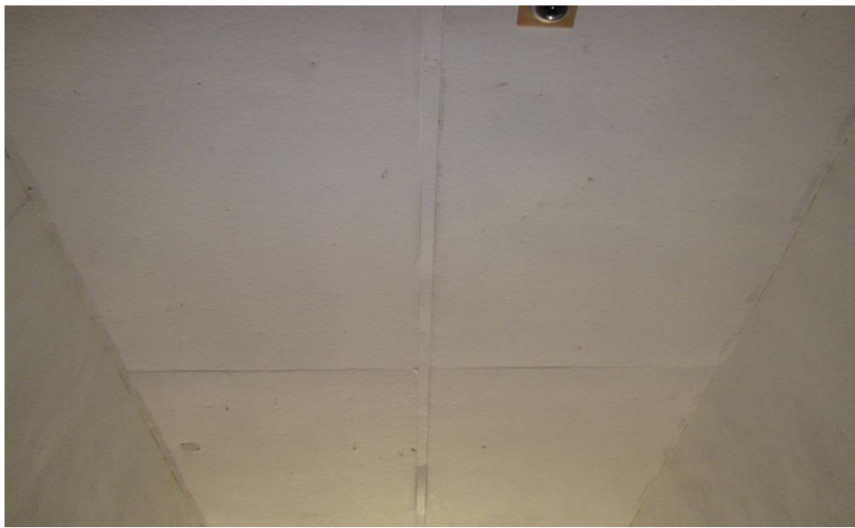
Photo 2 Location: Inside Elementary School Date: 08/06/2013 Looking at large ceiling tiles
