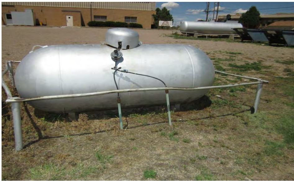
Photo 22 Location: West Side of School Date: 08/06/2013 Looking at smaller propane AST
