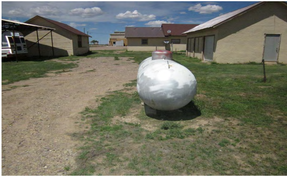
Photo 24 Location: West Side of School Date: 08/06/2013 Looking at propane AST
