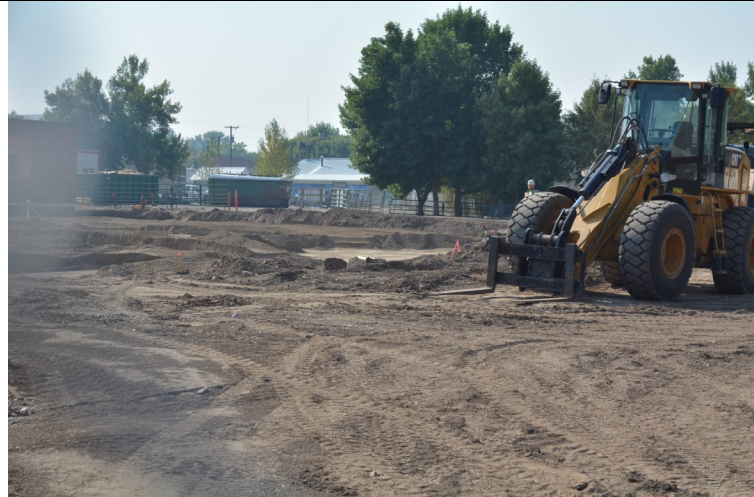
Construction visible from behind the shop. Taken 8/28/17
