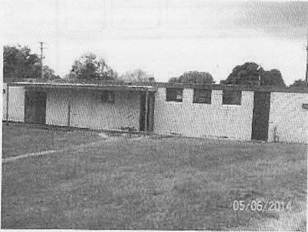
2015-066 Luling ISD - Weight Room Building
