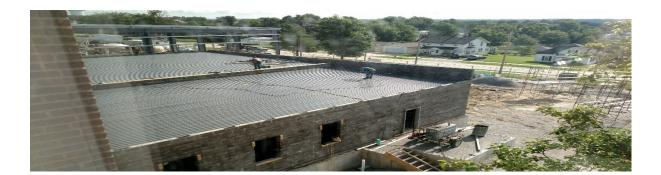
This is a NORTHEAST facing picture of the roof over the KITCHEN and Cafeteria-Commons Area. The area at the bottom of the picture is the NEW loading dock for the FOOD SERVICE deliveries. At completion, the roof will be an EPDM type; but currently the ironworkers are connecting/fastening the ceiling joists with the under roof. It's taking shape!
