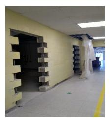
These are former door ways that are being replaced with BRICK/MASONRY to provide classrooms
