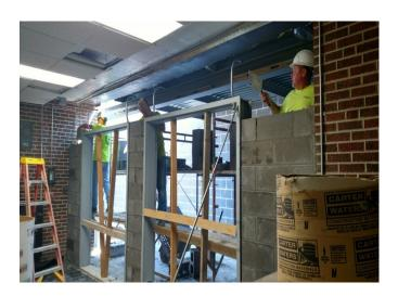
The former main GYM entry will be removed and new frames are being installed, with a block connection. This area will serve as the main connection area between the CURRENT gym and NEW gym
