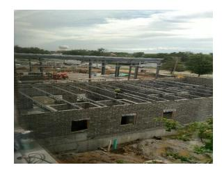
This is an 'above' perspective of the Kitchen – the three (3) windows are on the south side of the kitchen. The Bar Joists for the roof/ceiling are also installed.
