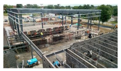
This is an extended view of the Cafeteria-Commons Area. The masonry blocks are being installed to the gym wall.
