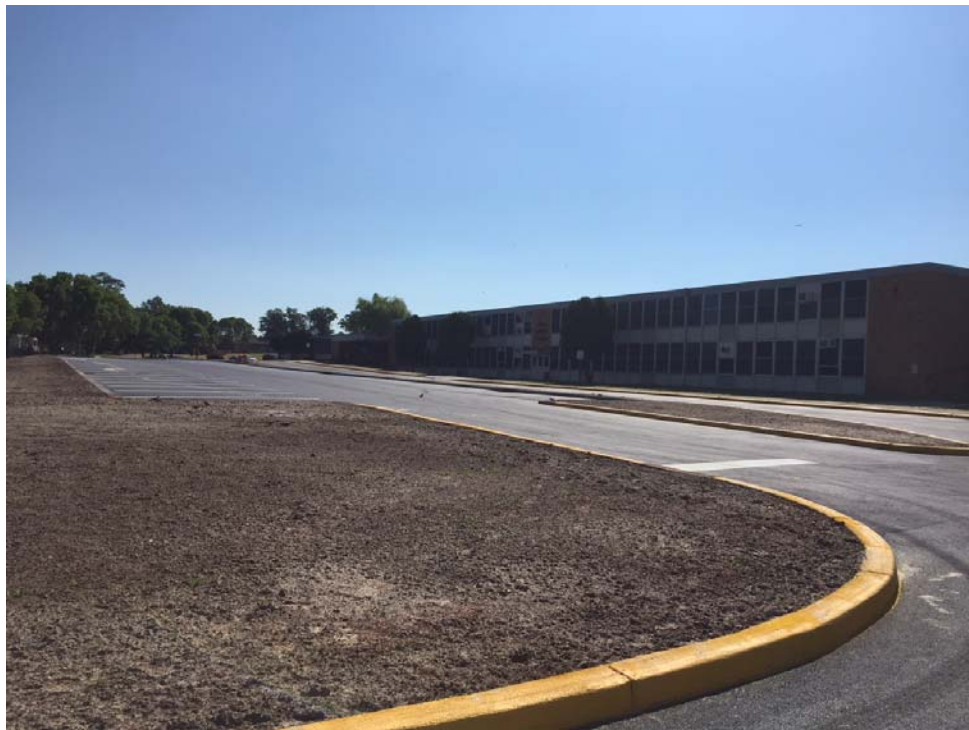
New parking lot at Avenel MS
