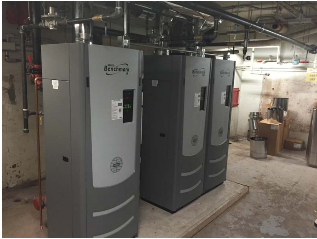
New boilers installed at our schools
