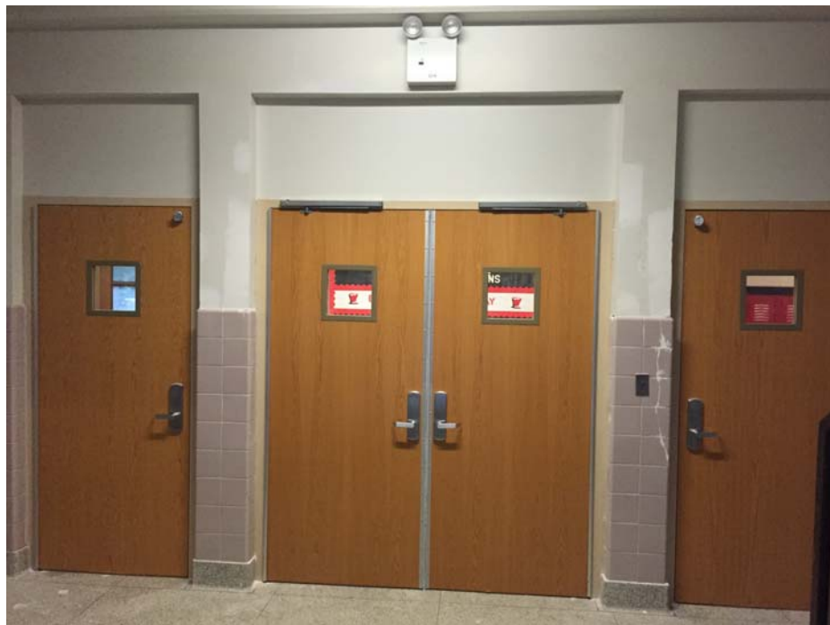
New fire doors at Woodbridge HS
