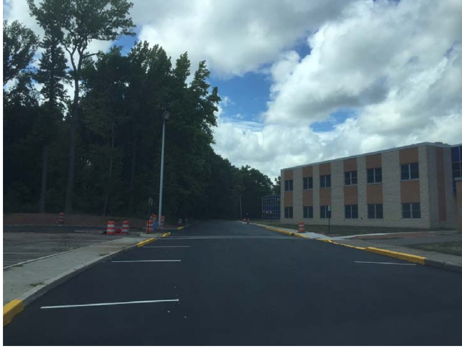
New paving at Colonia HS
