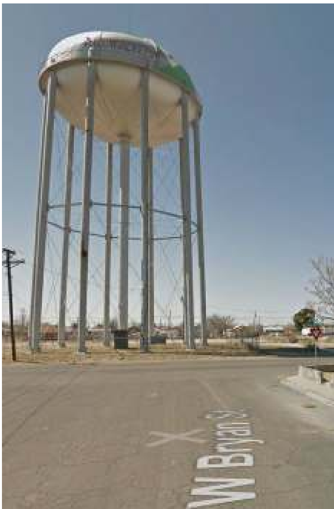
City of Kermit Water Tower
