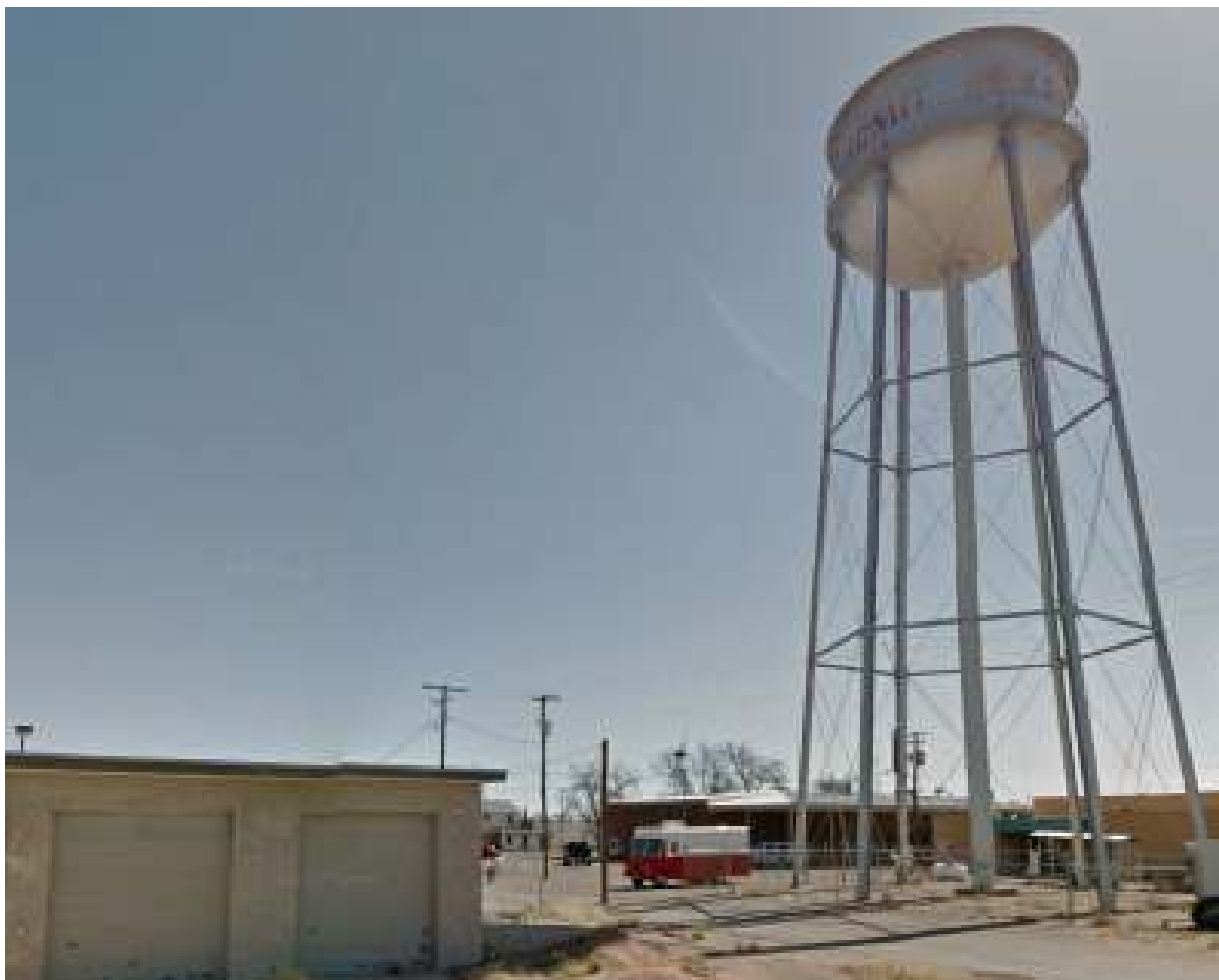
City of Kermit Water Tower
