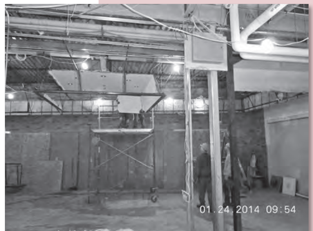
Above are pictures of the band and choral room renovation.
