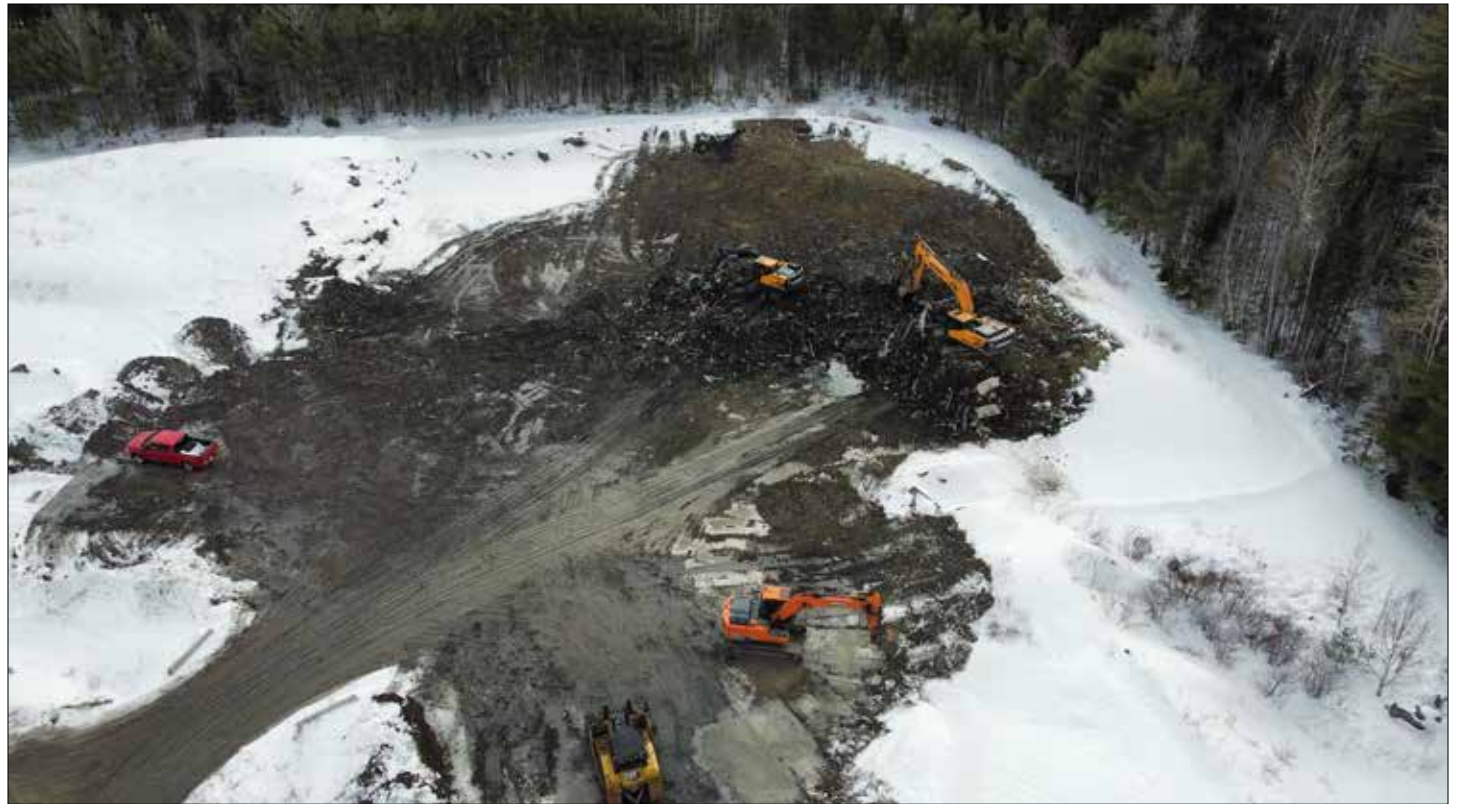
Crews excavate city's Construction and Demolition Debris Landfill.
