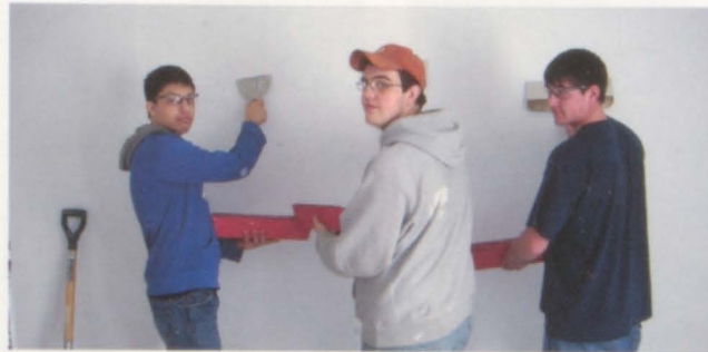
Senior Jalen Diede, junior Logen Lechner and sophomore Tyler Roe mud the newly drywalled room at VOED.
