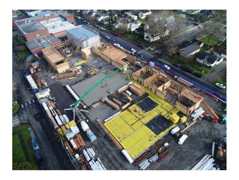
Lexington Elementary - Just a little behind Wallace Elementary due to permits (and weather has been very wet) Underground prep is well under way, electrical/mechanical/plumbing. They are pouring area 'C' this week, area 'A' in 2 weeks and area 'B' in 4 weeks, then they will start building "vertically". Photos show great progress in just 3 months!
