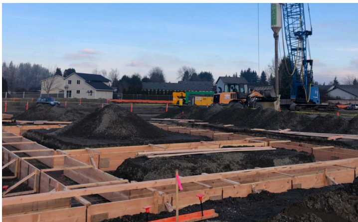
Gym & Commons Area Footing Forms
