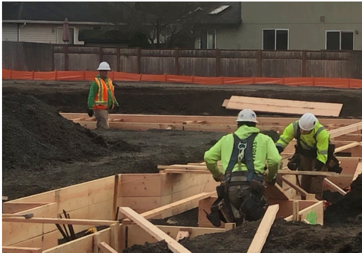
Forming up Footings
