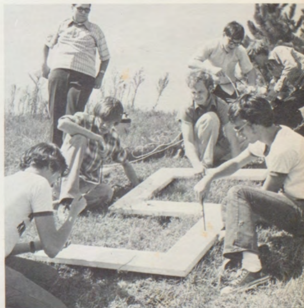
BLOCKHEADS Randy Smith, Ken Moyer, Rick Garner, Darrell Smith, Steve Williams, Stephen Rea and Mike Marshall prepare to block out in cement the traditional '75 on Cherry Hill.
