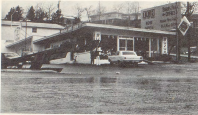
CLOSED DOWN after tornadoes struck in February, many North Little Rock businesses suffered hundreds of dollars in sales losses. Despite this fact, North Little Rock was not considered a disaster relief area.
