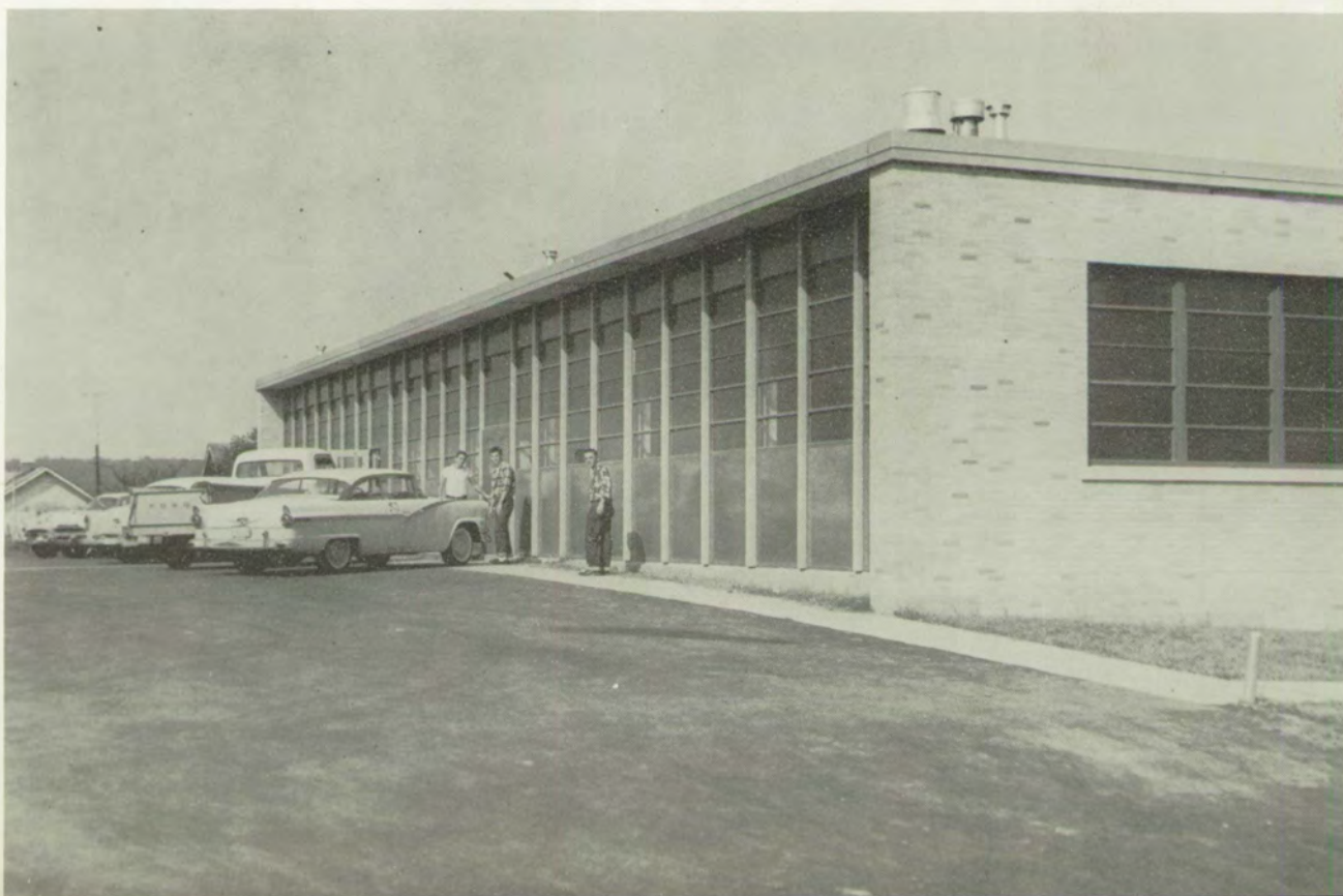
ALL GLASS south wall of the Vocational Arts Building.
