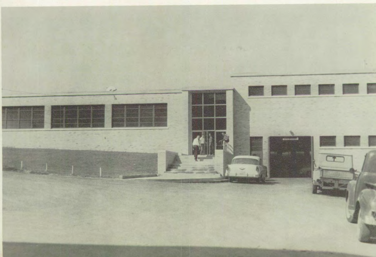
FRONT ENTRANCE to the Vocational Arts Building faces the east.
