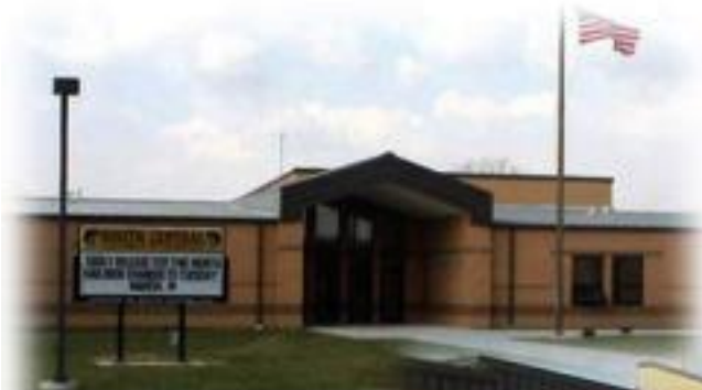
South Central Elementary & Middle School
