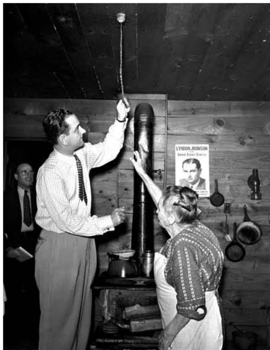
HILCO was among the first co-ops in Texas to bring electricity to rural areas.
