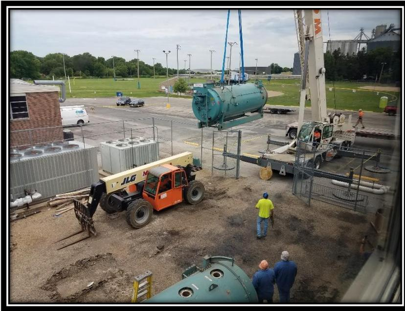
**Removal of old boilers from BRHS, as part of the energy efficiency project.**
