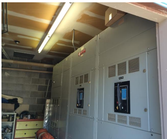
Figure 22: Main Metered Service Switchboard at Electrical Room
