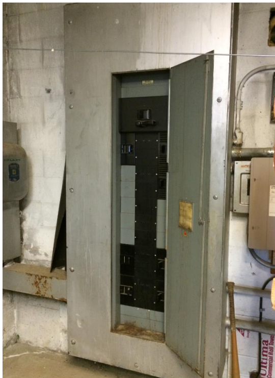
Figure 5: Service #1 120/240V Switchboard at Electrical/Storage Room
