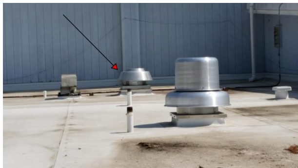
Figure 3: New Kitchen Exhaust Fans
