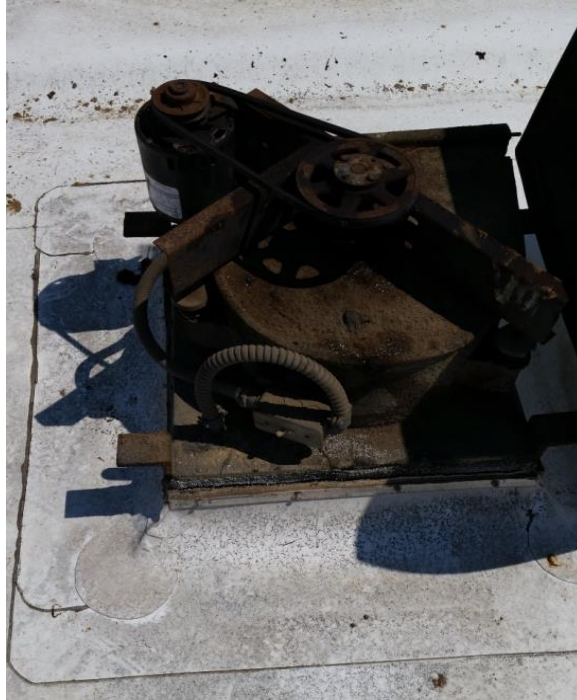
Figure 17: Exhaust Fan with Cover Lifted Off, Exposing Rusted Components
