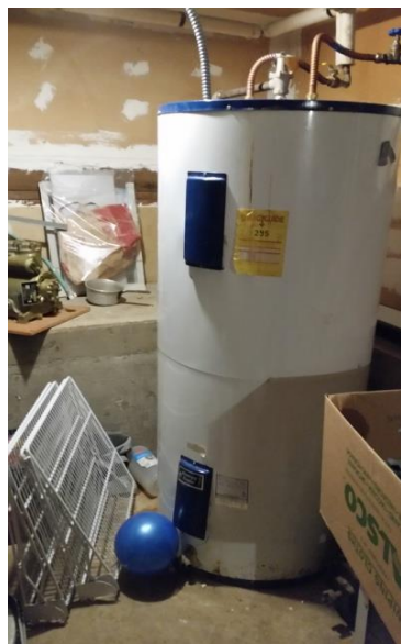
Figure 4: Water Heater below Kitchen without Seismic Bracing
