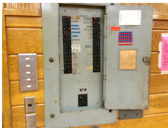
Figure 6: Service #2 277/480V Equipment at Building Exterior
