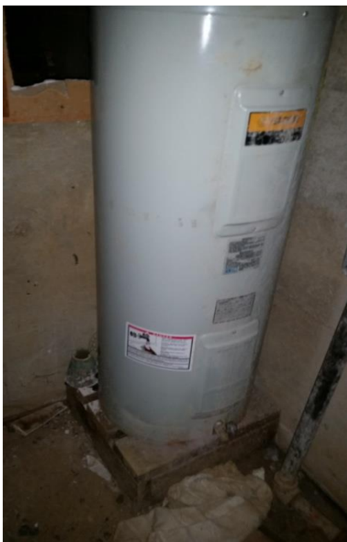
Figure 18: Water Heater in Stage Pit without Seismic Bracing
