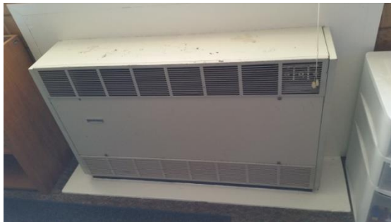
Figure 1: Unit Ventilator Console
