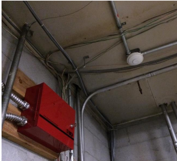
Figure 10: Existing Fire Alarm Control Panel in Electrical/Storage Room
