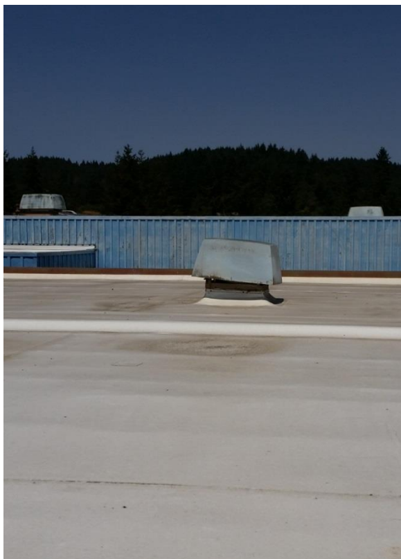
Figure 16: Several Roof Exhaust Fans. The near unit with a broken cover support.
