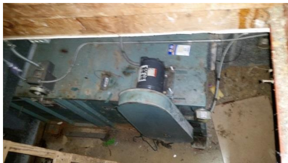
Figure 15: Stage Pit Forced Air Fan Unit
