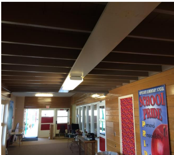
Figure 8: Surface Wrap in Corridor
