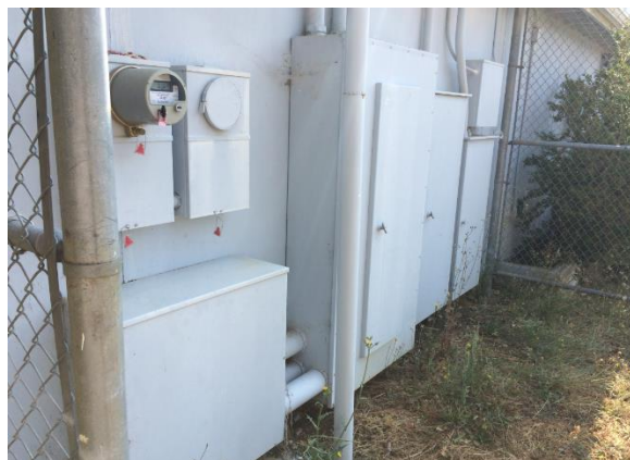
Figure 6: Service #2 277/480V Equipment at Building Exterior
