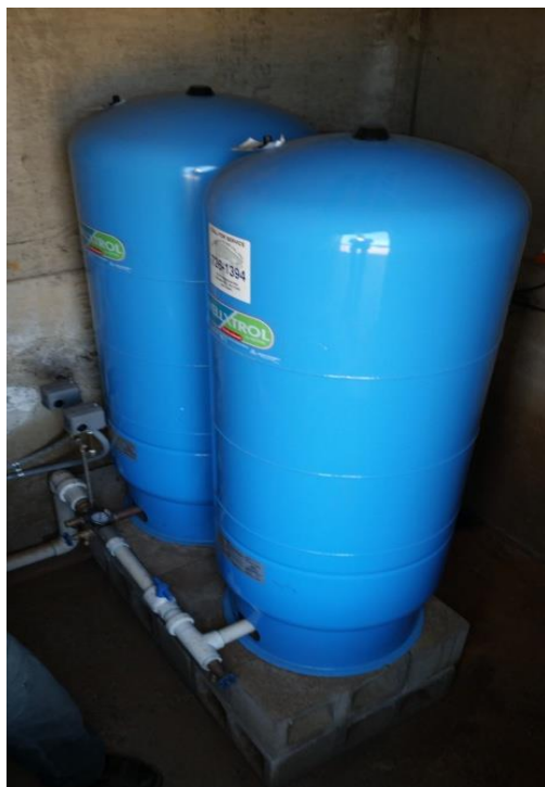
Figure 19: Pump House Pressure Tanks without Seismic Bracing
