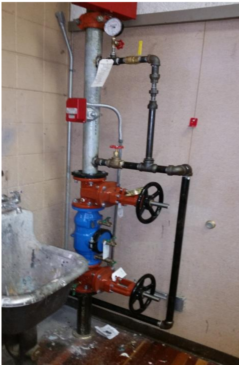
Figure 21: Fire Sprinkler Riser for Stage Area
