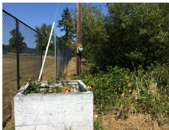
Figure 23: Existing 120/240V Metered Service at Pond
