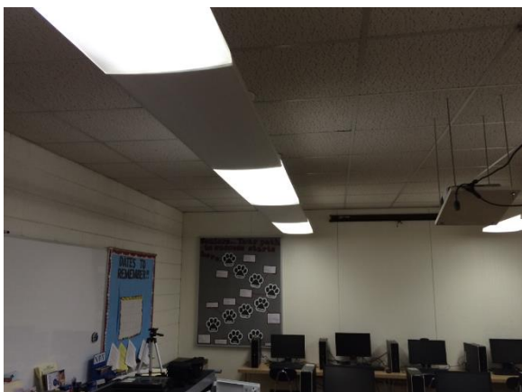
Figure 24: Linear Fluorescent Pendants at Computer Lab Classroom
