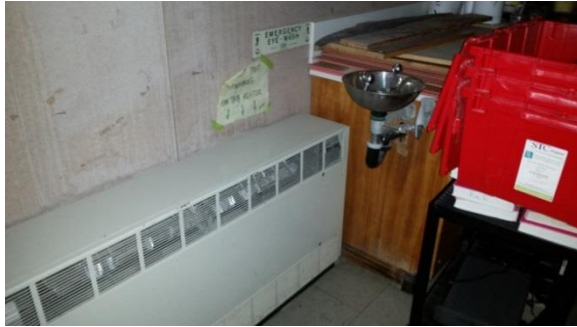
Figure 20: Science Room Emergency Eyewash Close to an Electric Unit Ventilator Console.
