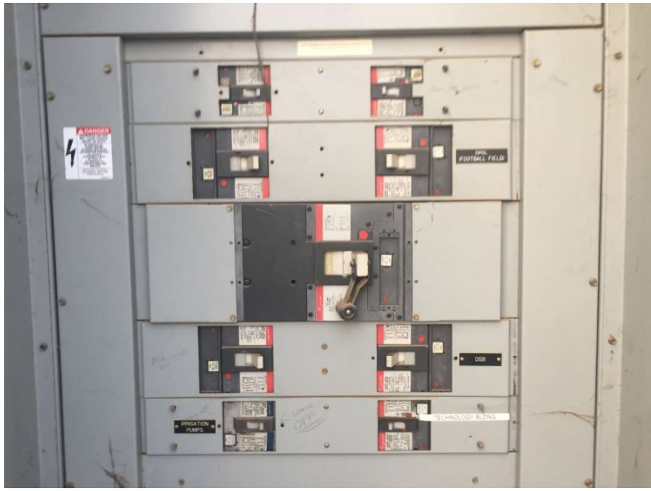
Picture 4: Circuit breakers to individual buildings
