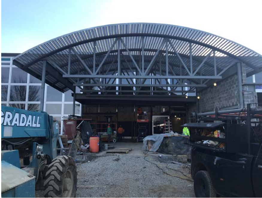
New main entrance to Auditorium and Administrative wing.
