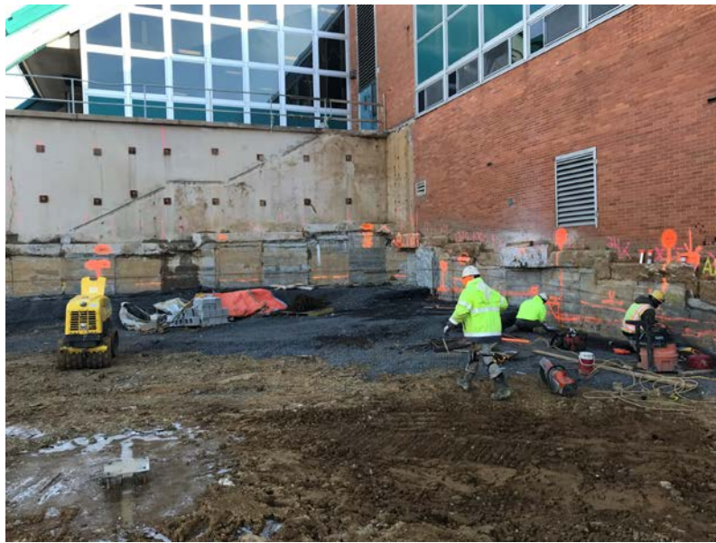
Excavation work for the Auxiliary Gymnasium.
