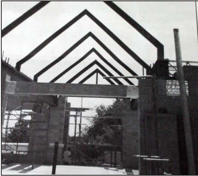
Construction on the PLES commons during 1992 renovation work
