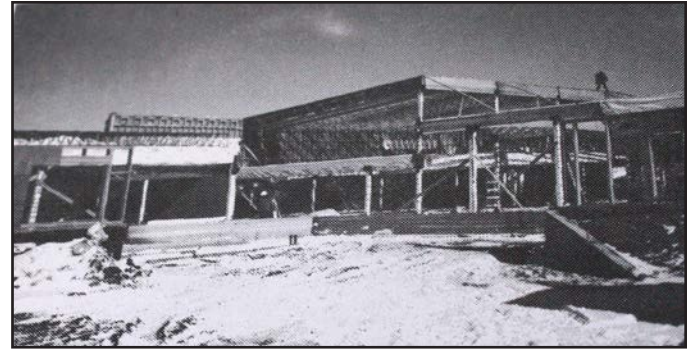
Kilmer Elementary under construction in 1988
