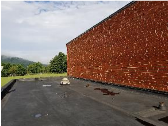
Photo #1 View of the roof over the locker room.
