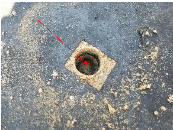
Photo #5 View of built-up roofing (HA-A) on the locker room roof.
