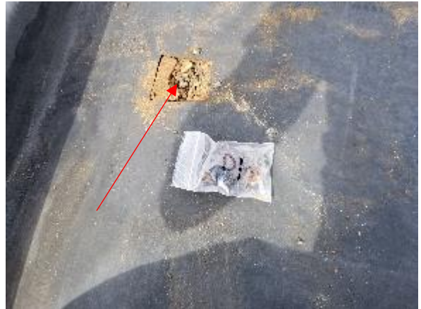
Photo #8 View of built-up roofing (HA-D, same as HA-F) on the eastern roof sections.
