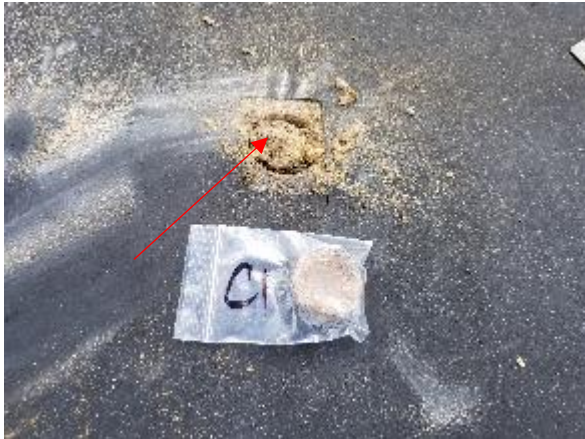
Photo #7 View of built-up roofing (HA-C, same as HA-E) on the eastern roof sections.
