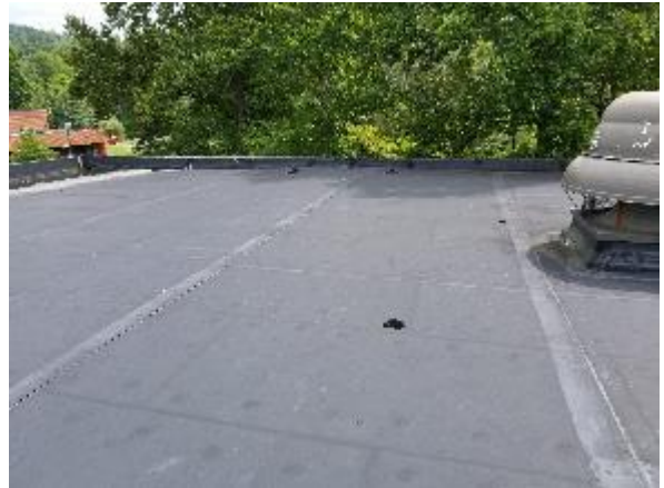
Photo #2 View of the roof over the high bay gym.
