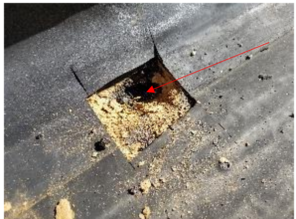
Photo #6 View of wall flashing (HA-B) on the locker room roof.
