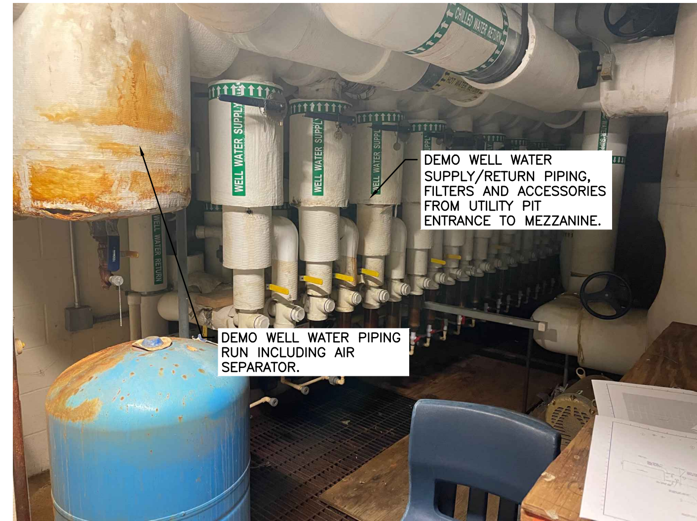
1 PHOTO 1: DEMO WELL PIPING/ACCESORIES MD-401 SCALE: NTS
