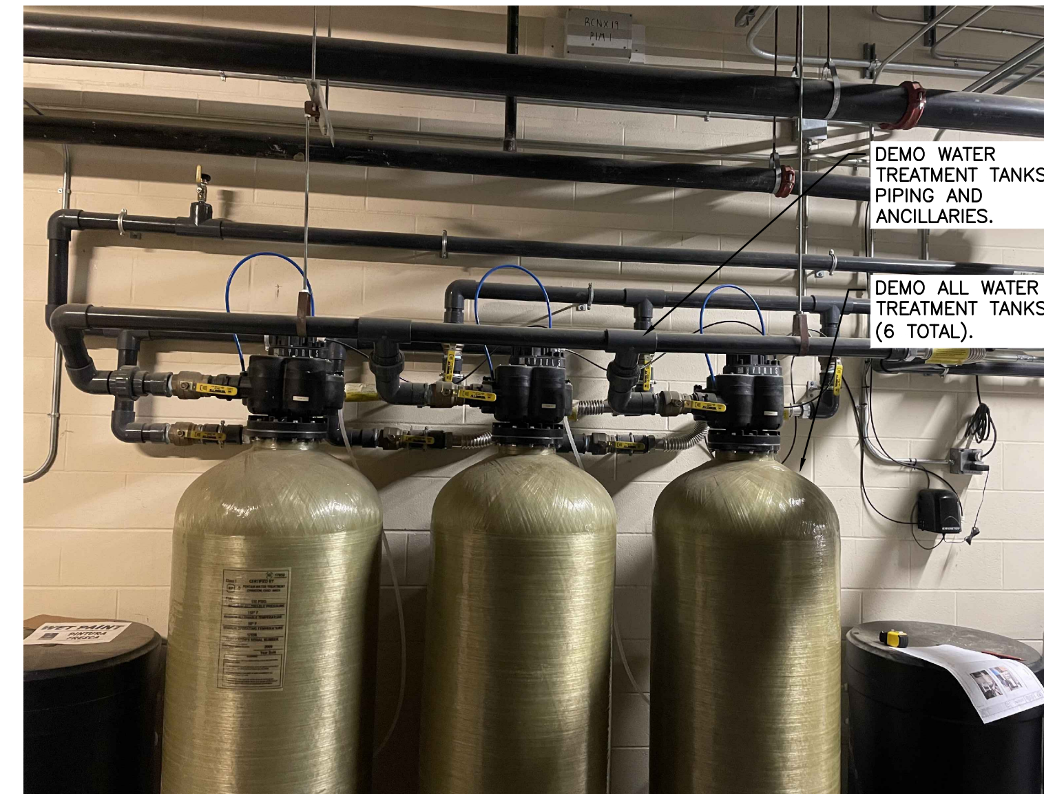
3 PHOTO 3: DEMO WATER TREATMENT TANKS AND PIPING MD-401 SCALE: NTS
