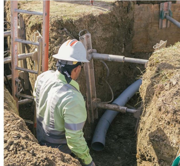
Julian Undergrounding Project
