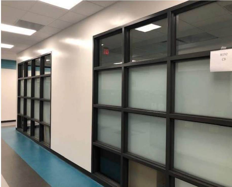
New Small Group Rooms are complete
