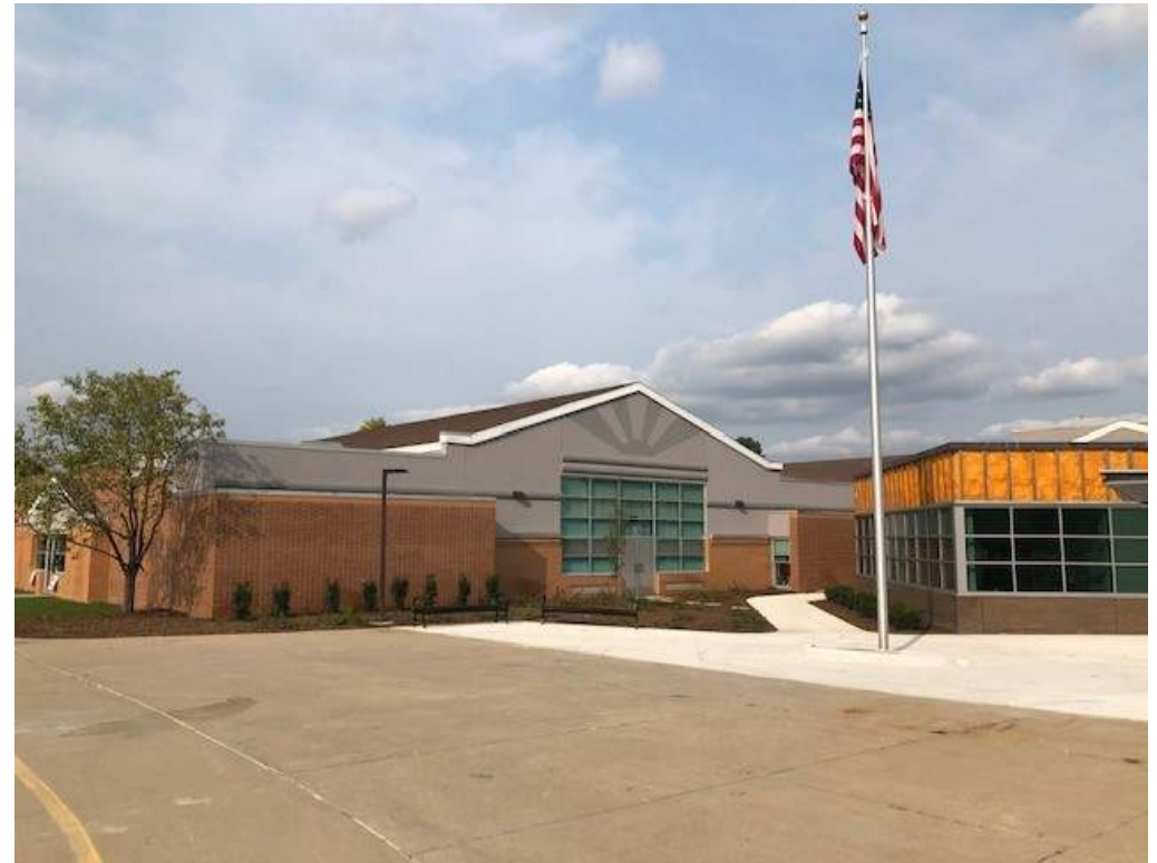
Repair and refinish of the Exterior Finish Insulation System around the entire school is complete.
