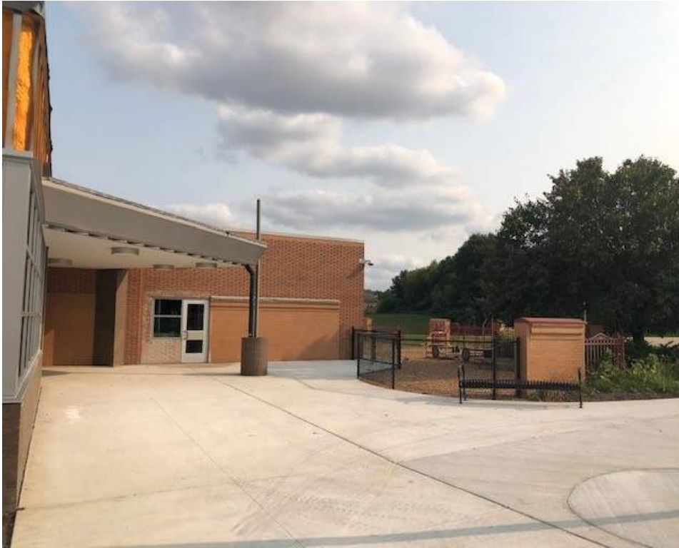
New vinyl clad fencing is installed to secure the playground area
