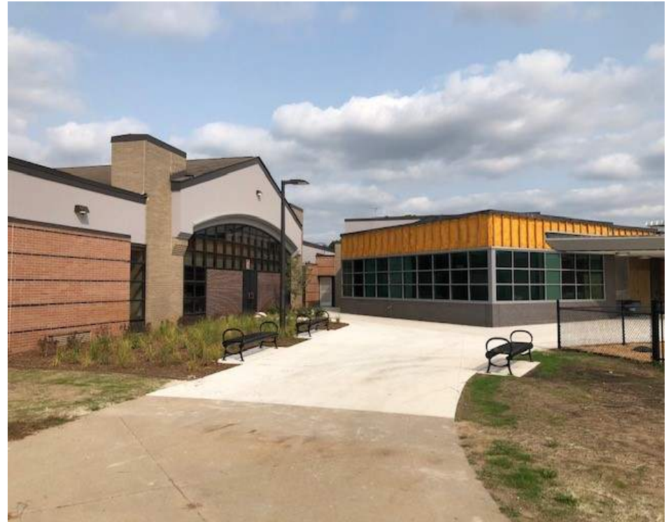
Landscaping is complete and benches have been set at the new Secured Entry Addition
