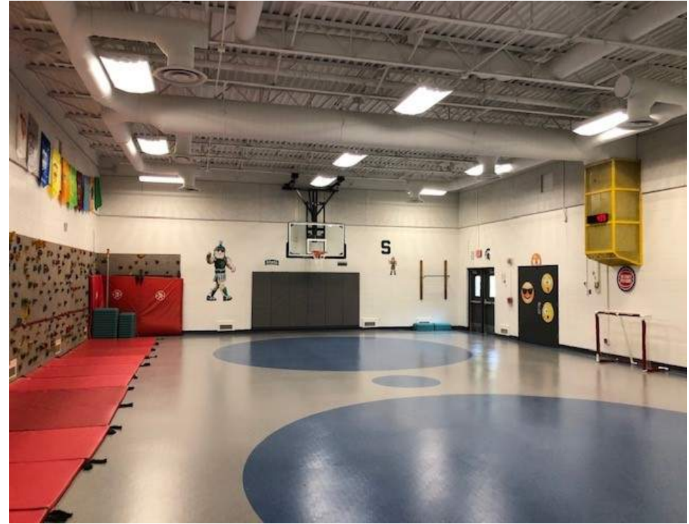
The existing gymnasium has been repainted, along with installation of new glass basketball backboards, new acoustical wall panels and pads and new rubber flooring and base
