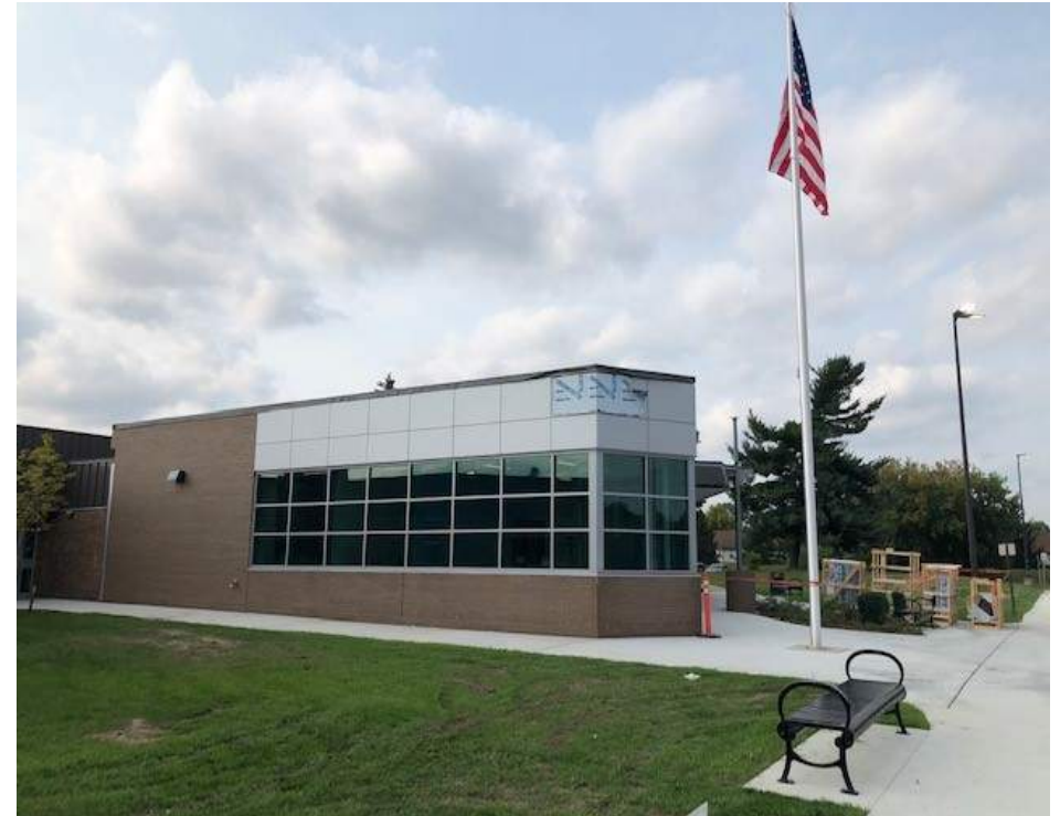
Metal Panels are being installed on Secured Entry
