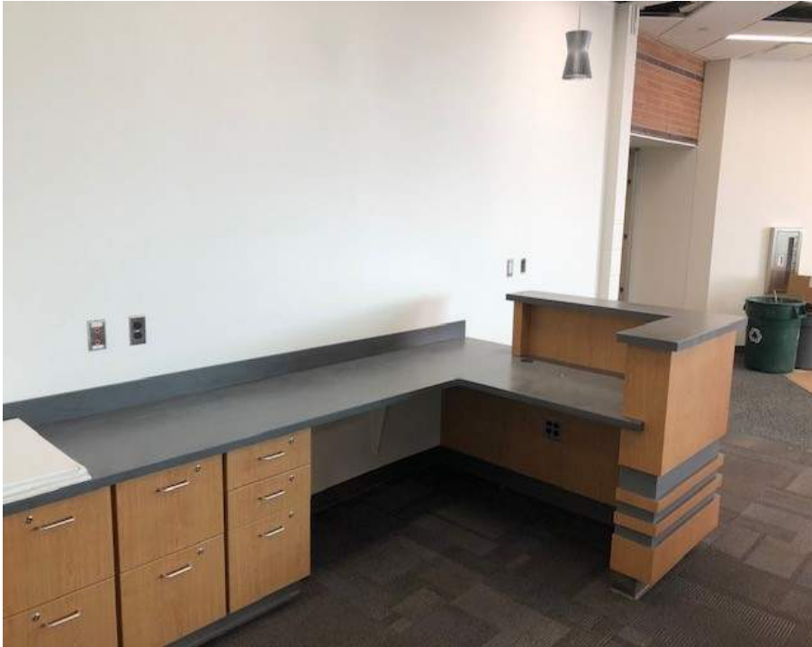
Reception Office millwork is installed in Secured Entry Addition
