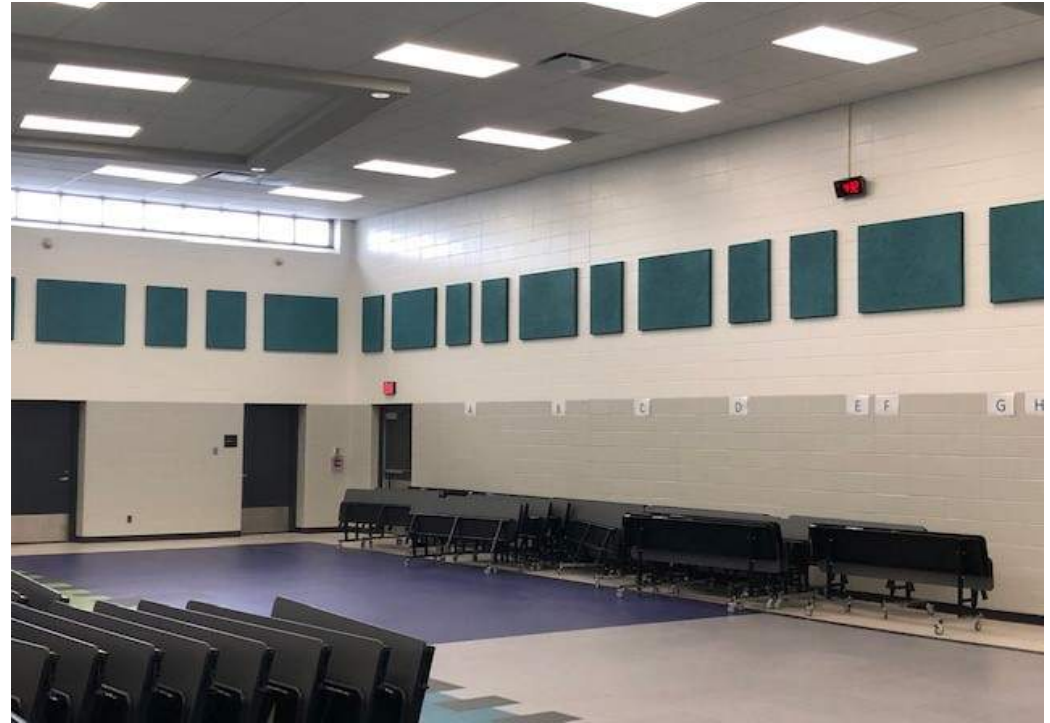
The existing Multipurpose Room has a new acoustical ceiling, new lighting, acoustical wall panels, painted walls and LVT flooring and base
