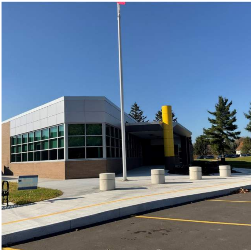
Concrete bollards have been installed
