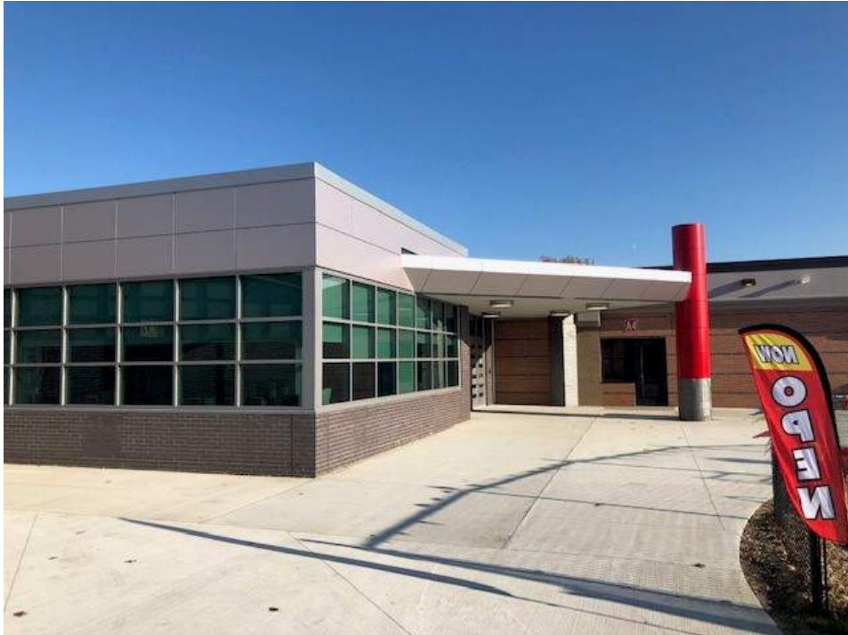
Metal panels and metal copings are complete
