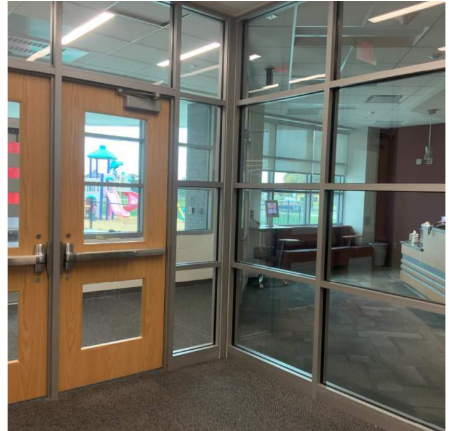
Secured entrance vestibule is complete
