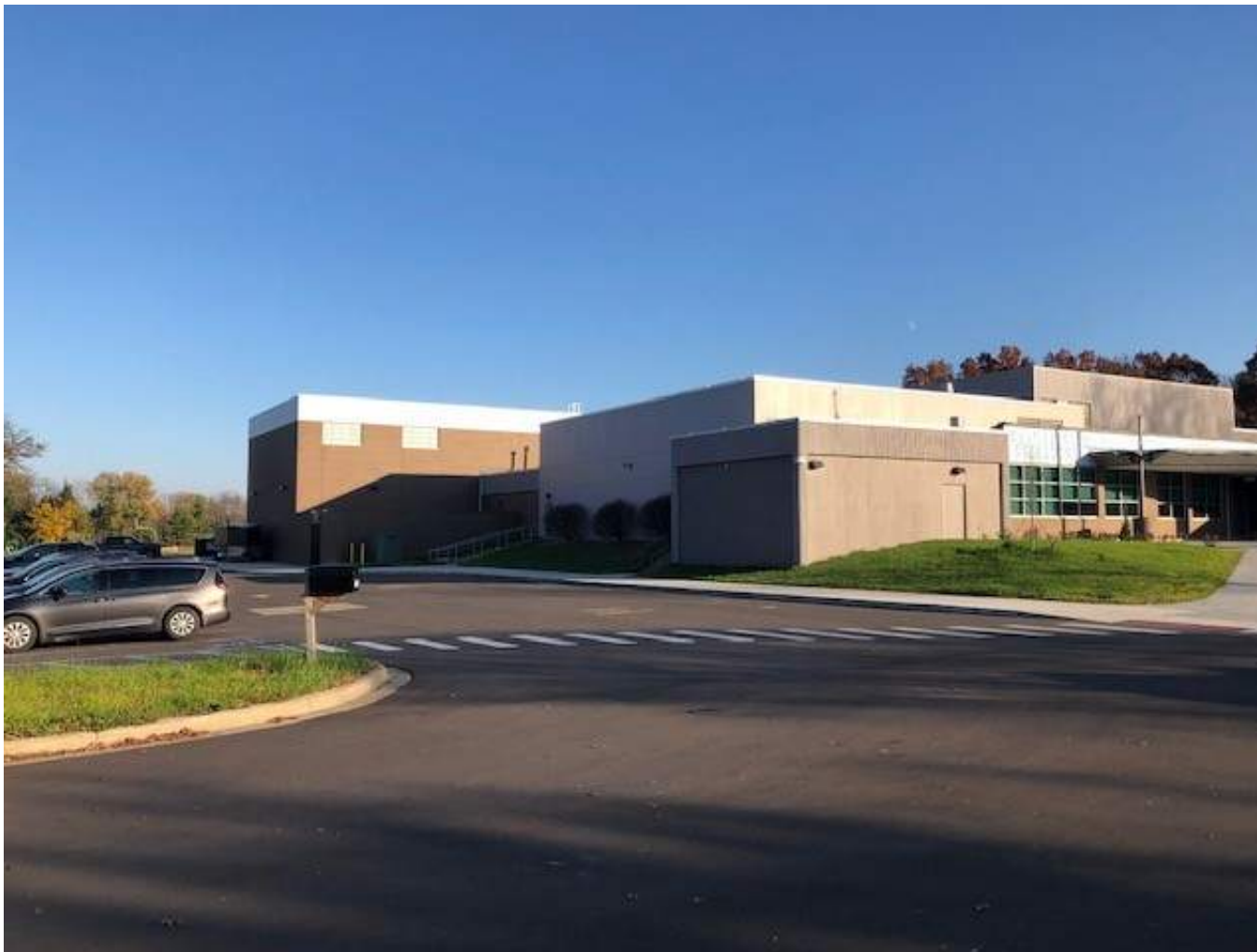
View of New Gymnasium / Classroom Addition and Secured Entry Addition
