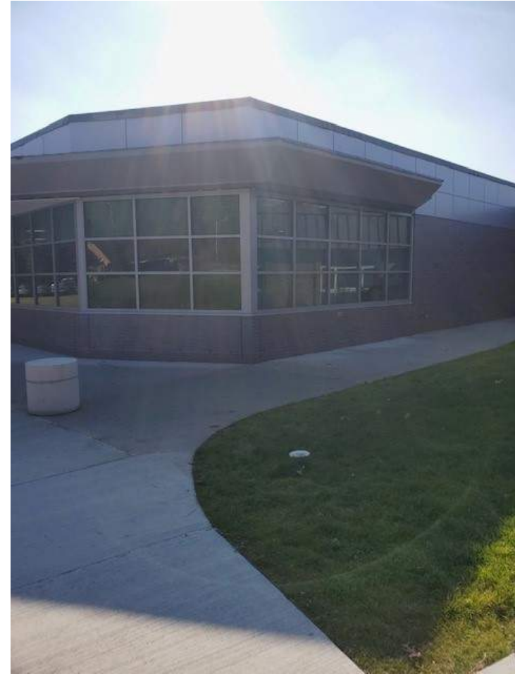
Metal Panel installation is underway
