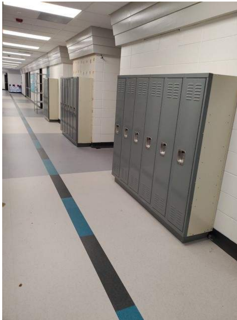
Installation of new lockers is underway
