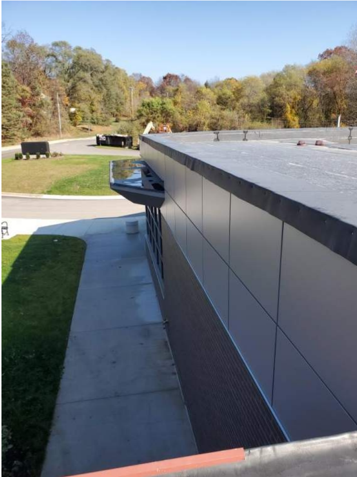
Metal Panel installation is underway
