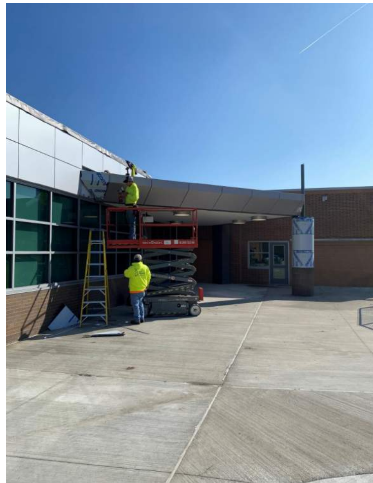
Metal panels at secured entry addition are being installed
