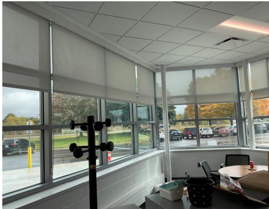
Roller shades have been installed
