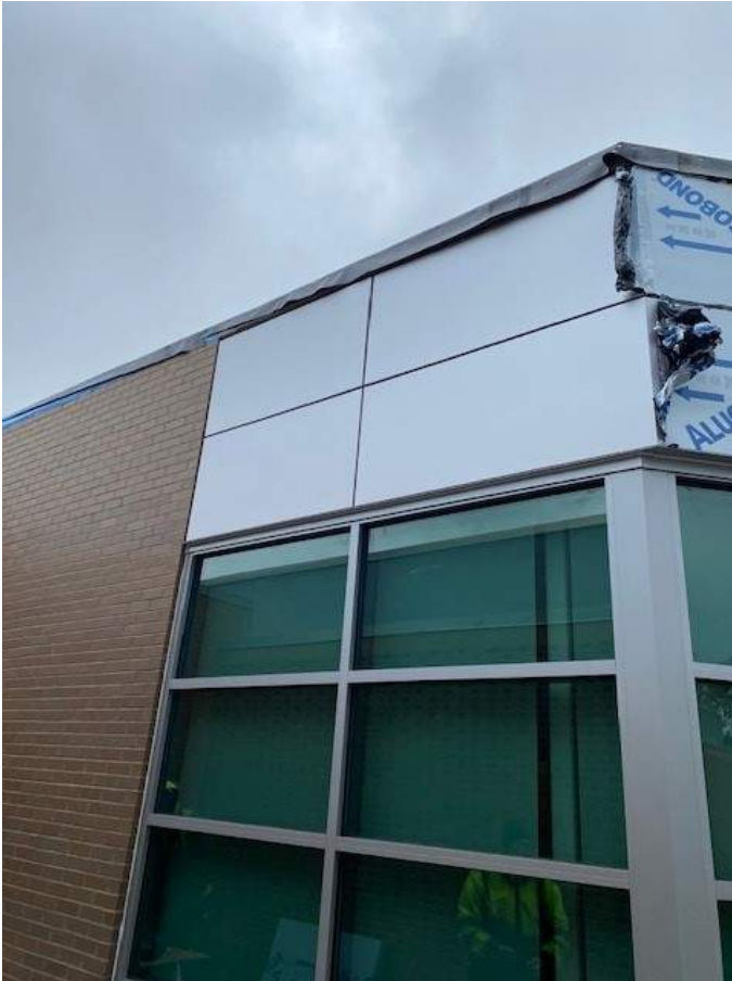
Metal panels are being installed at the secured entry addition.
