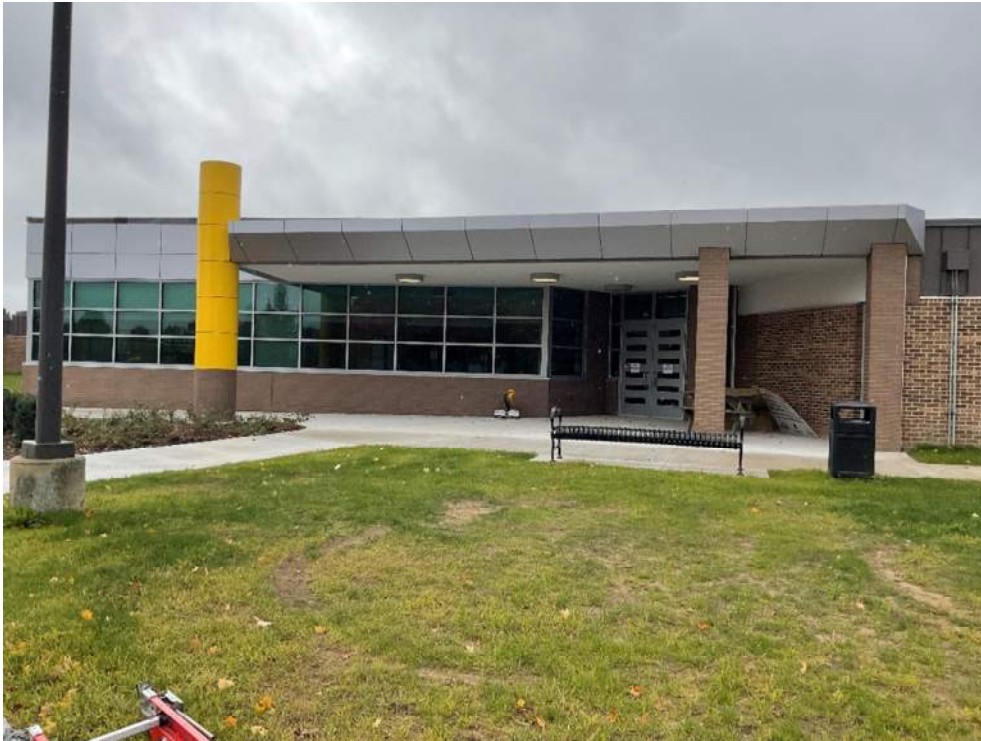
Completed secured entry metal panels.
