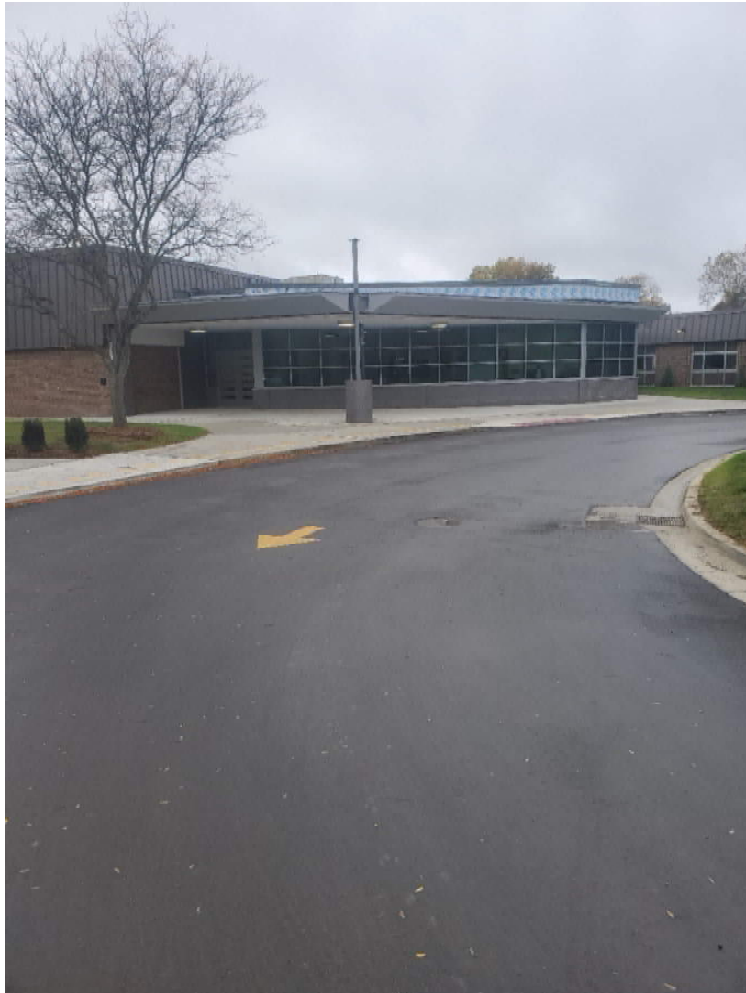
Ice & Water Shield has been installed at the metal panels.
