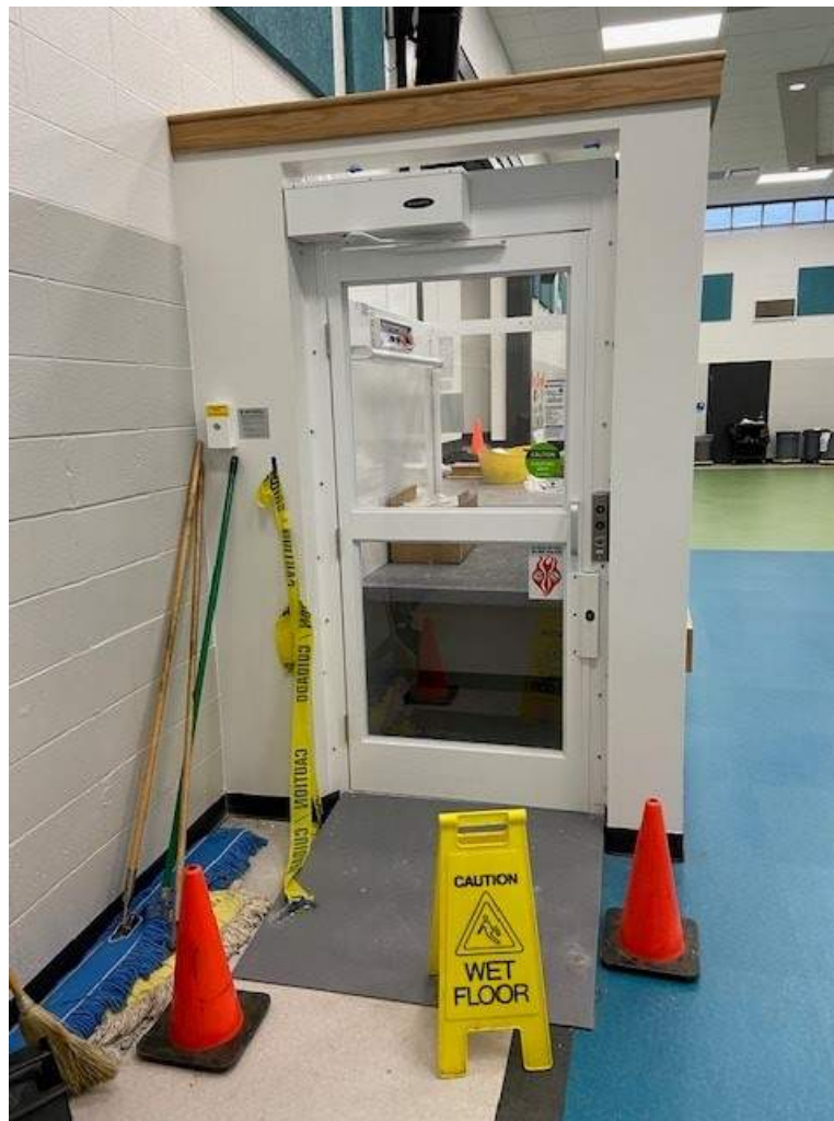
New wheelchair lift in the Multi-Purpose Room.
