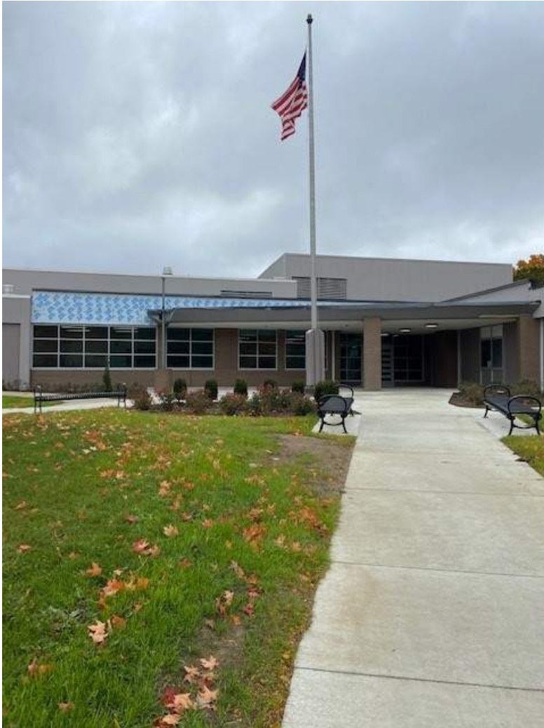
Ice & Water Shield installed at the metal panels.
