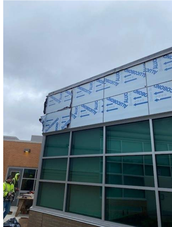
Metal panels are being installed at the secured entry addition.
