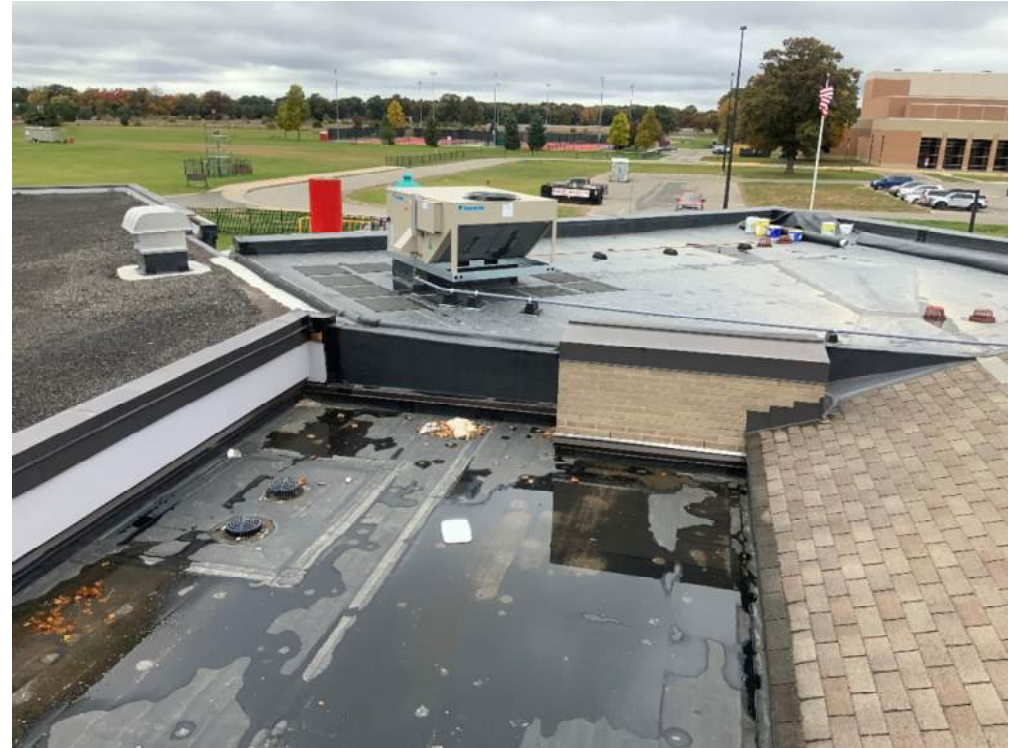
The rooftop unit (RTU) is set for the secured entry addition.
