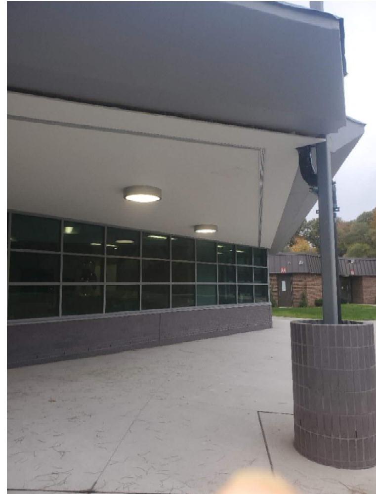
Vent strip has been installed at the secured entry addition canopy.
