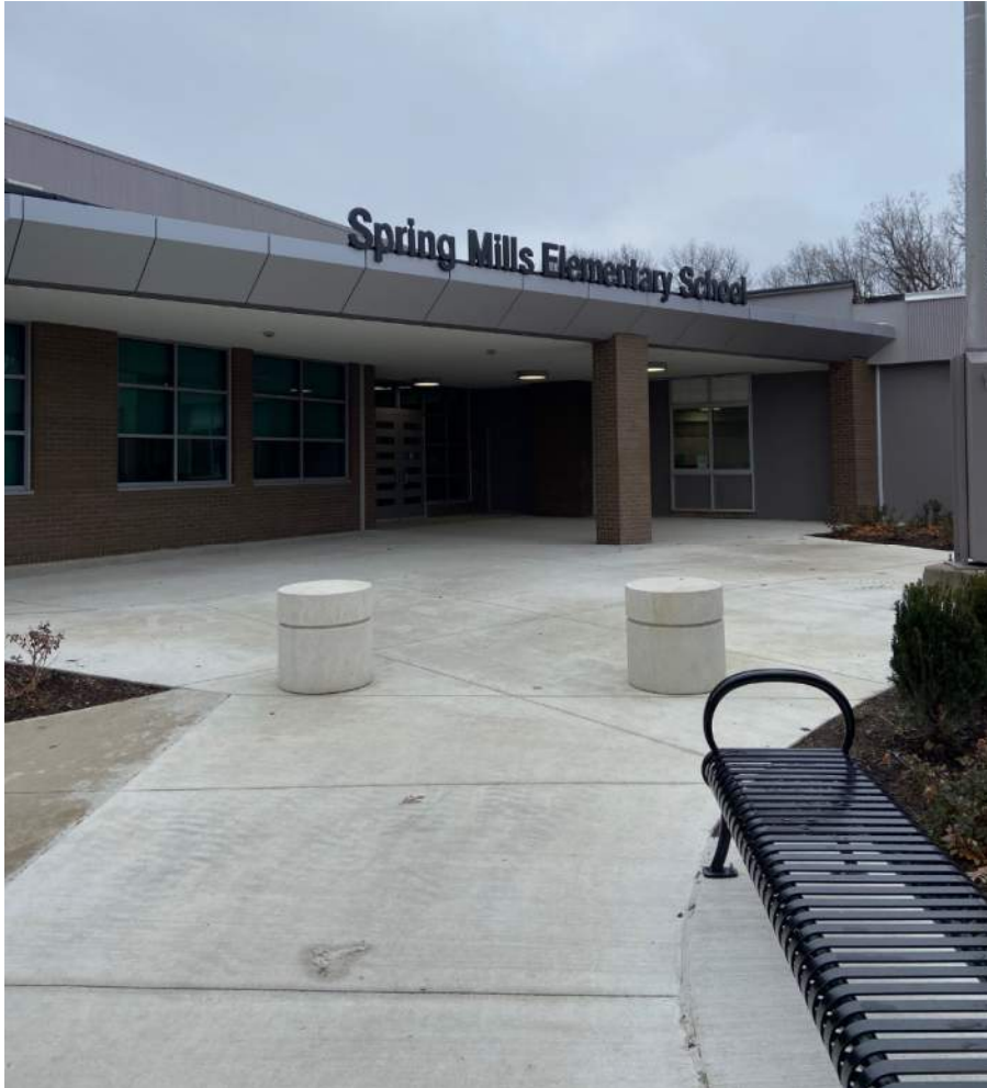
School Lettering and Metal Panels are complete
