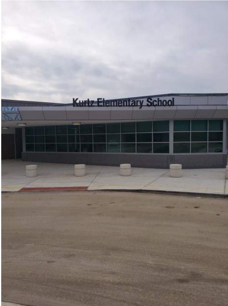
School Lettering is installed
