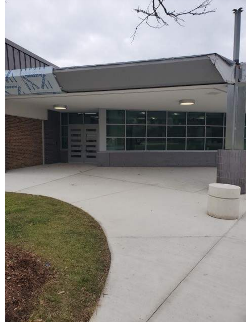
Metal panels installation is in progress
