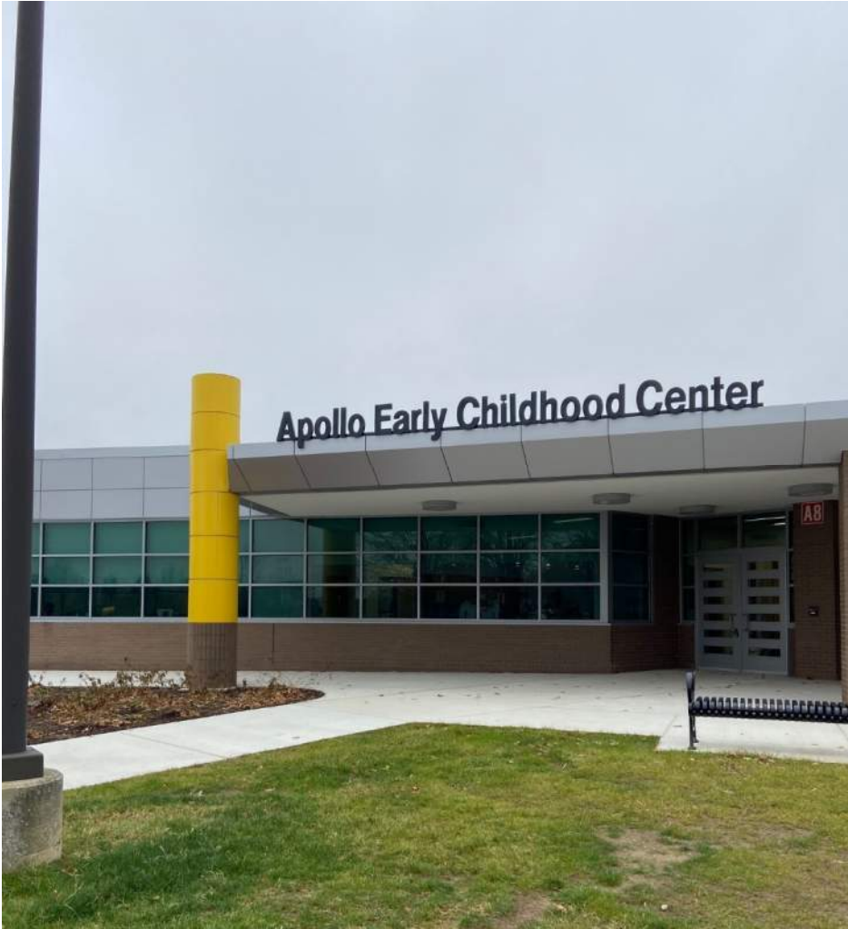
School Lettering & Metal Panels are complete
