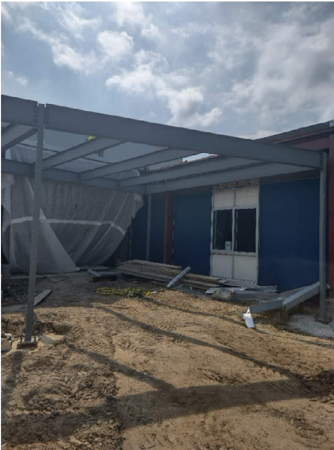
Canopy framing is erected for the new secured entry
