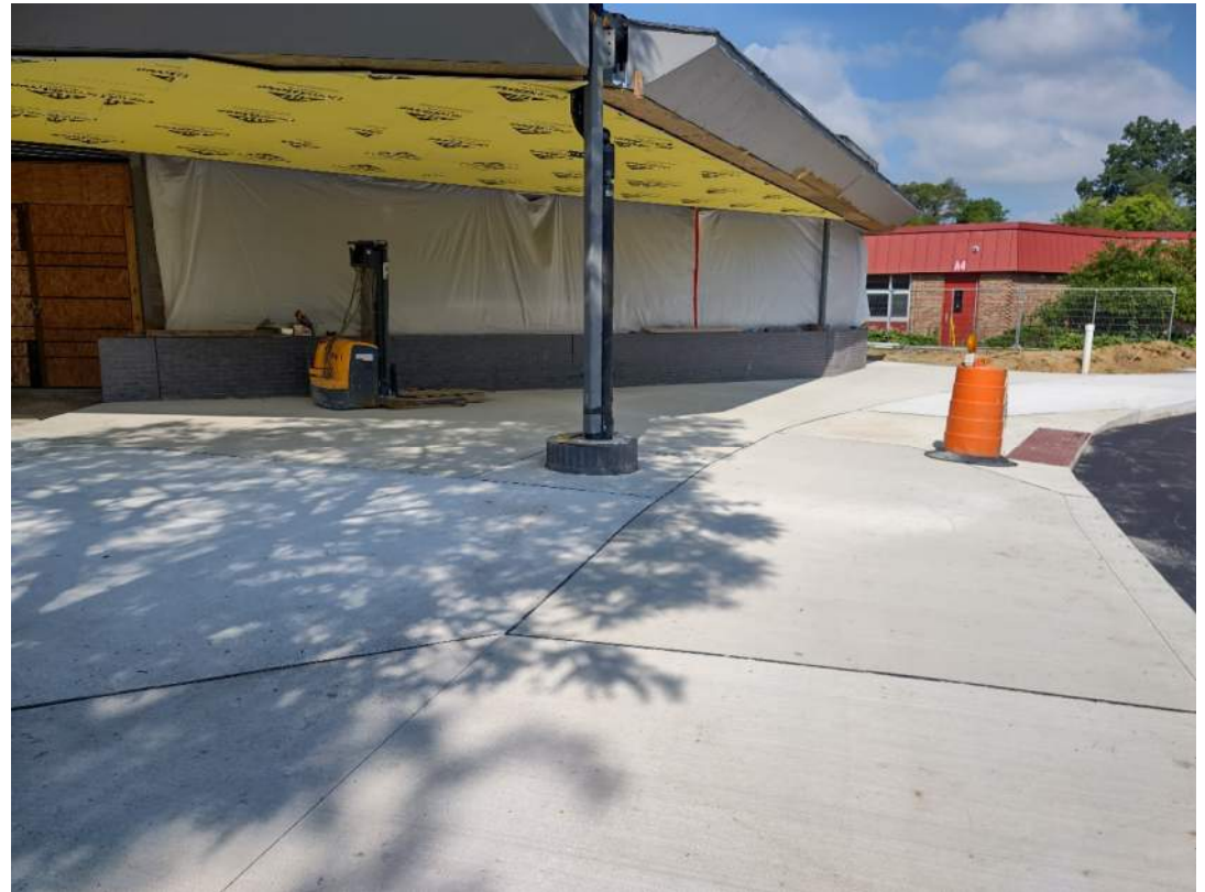
New sidewalk in front of the secured entry area.
