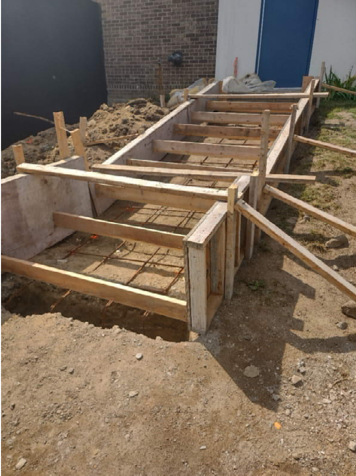
Formwork for the new steps going into the building.
