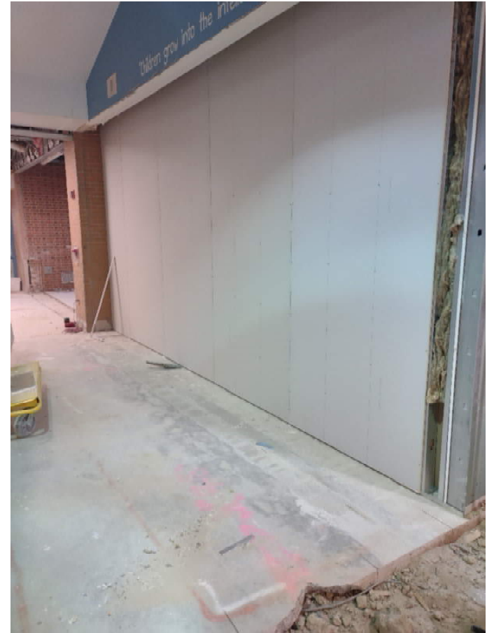
Drywall going up in the hall area of the secured entry.
