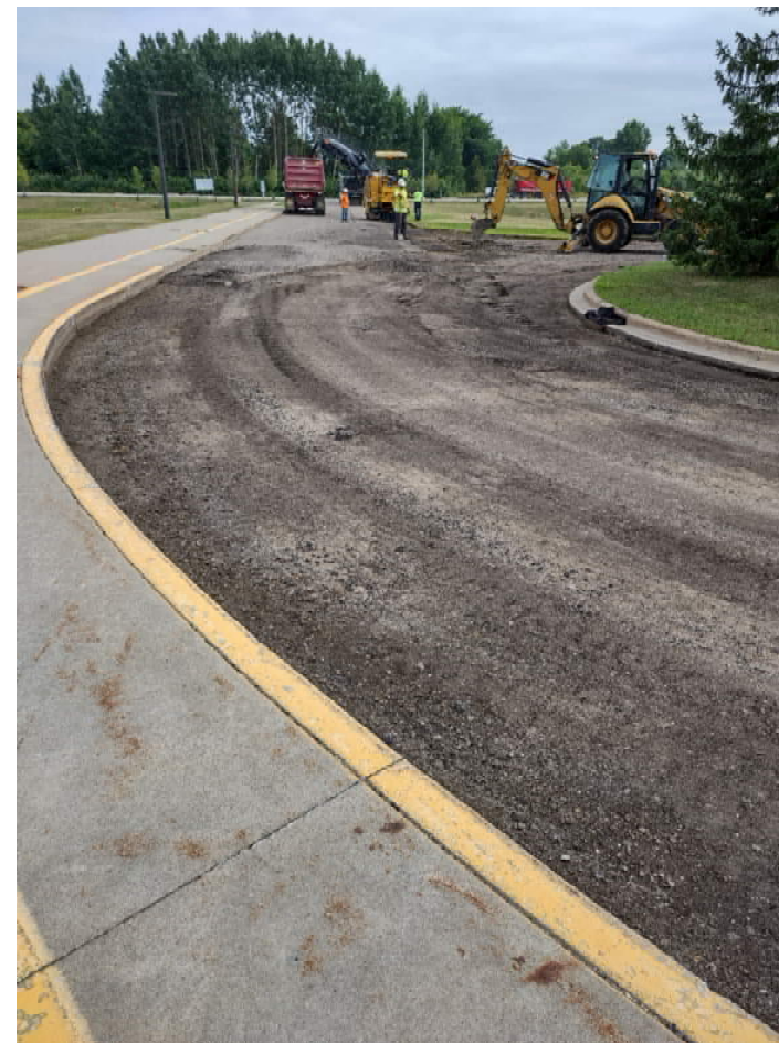
Pavement being removed for replacement on the drop-off. drop-off.
