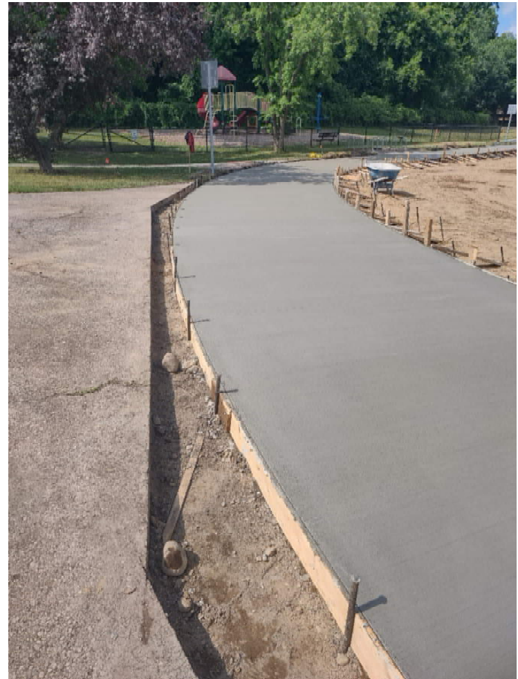
New sidewalk poured in front of the entry and drop-off area.
