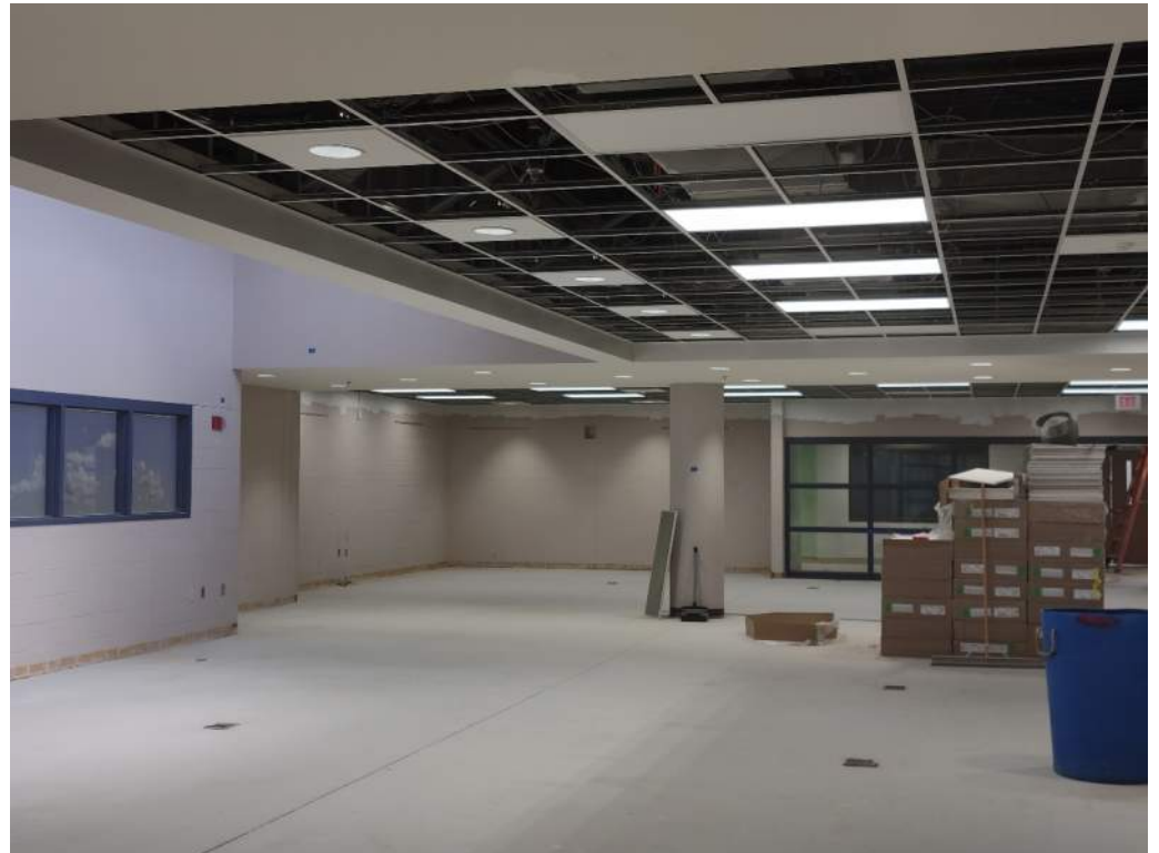
Ceiling grid and lights up in the media center.
