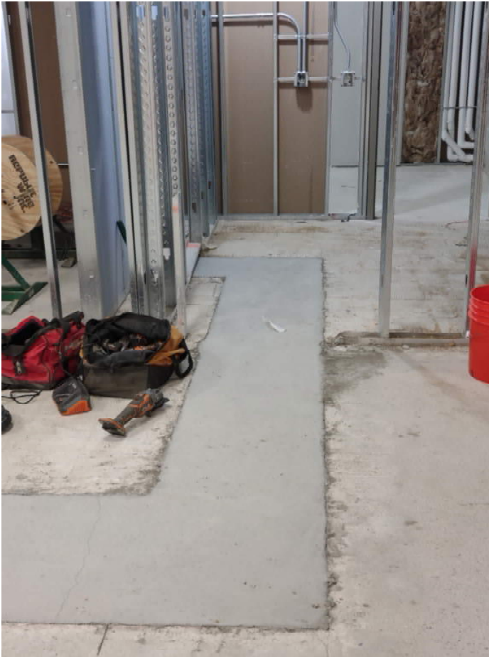
Underground complete going into the secured entry area, new concrete pored.
