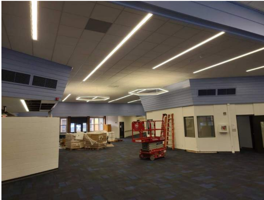
Media center ceiling, lights and flooring is complete
