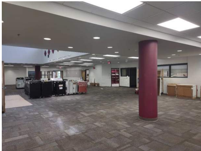
Media Center painting, flooring, and ceiling are completed
