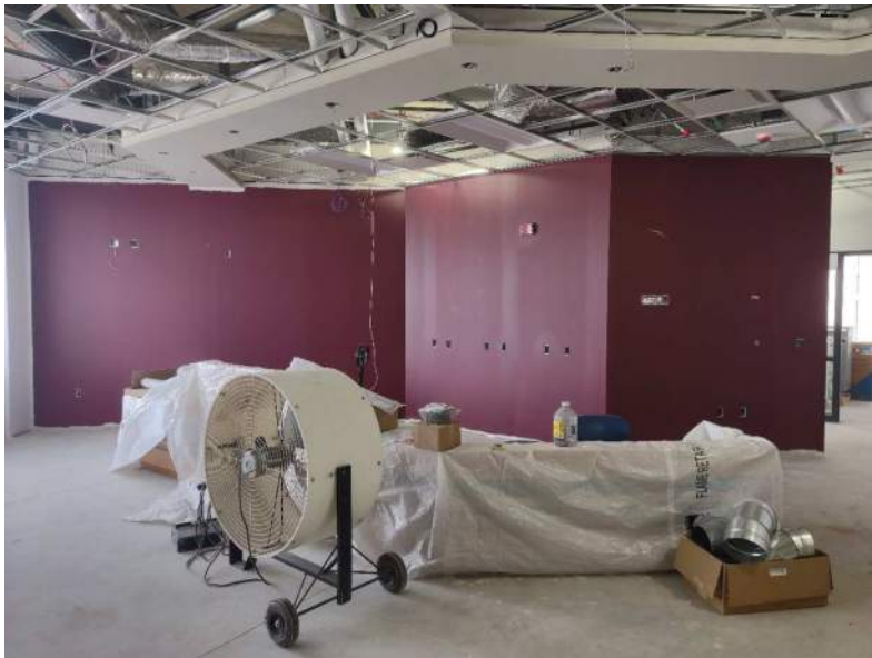
Secured entry addition is being painted and casework is being installed
