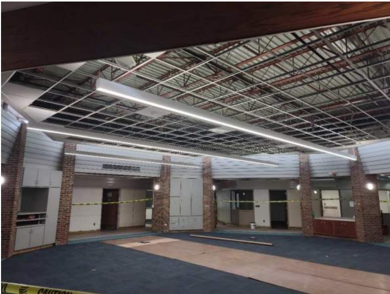
Resource Center carpeting and hanging lights have been installed
