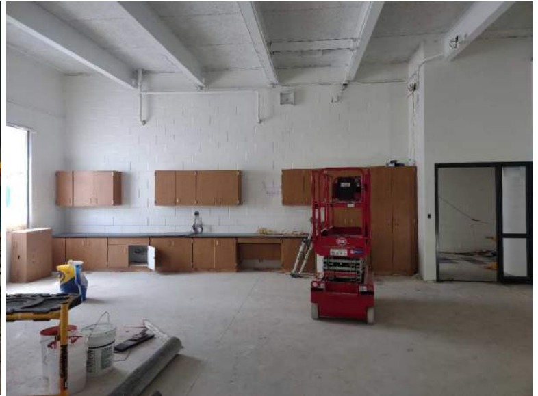
New casework is being installed throughout the school and Classroom Addition
