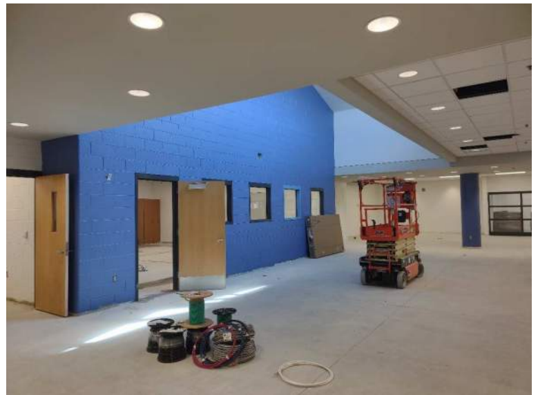
Media center has been painted. Full ceiling tiles are being installed
