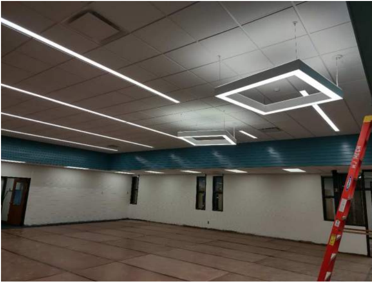
Media Center carpeting, lights and ceiling tiles are complete
