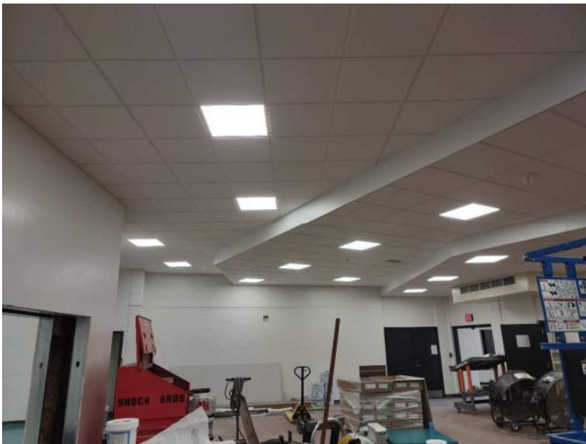
Motor Skills Room ceiling is complete
