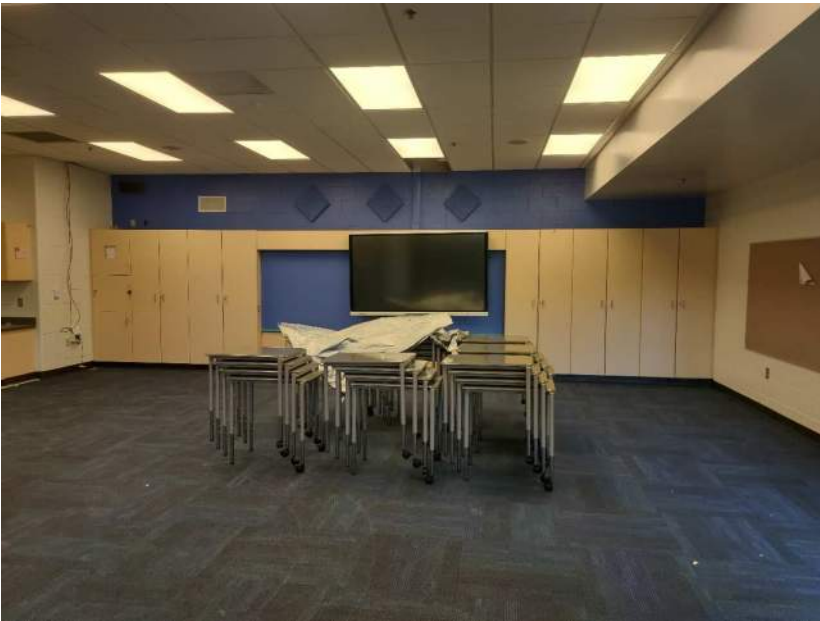
Classrooms are having Smart Boards installed and furniture is being delivered
