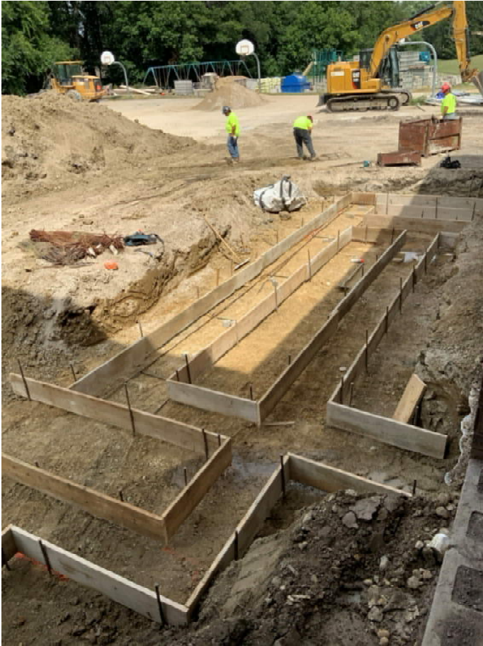
Ramp wall foundations for the Gymnasium and Classroom addition being formed
