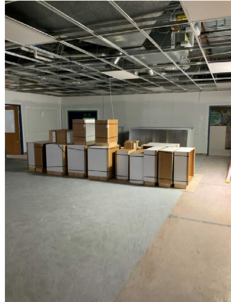
New ceiling grid and lights in the classroom area. Casework is ready to be installed.
