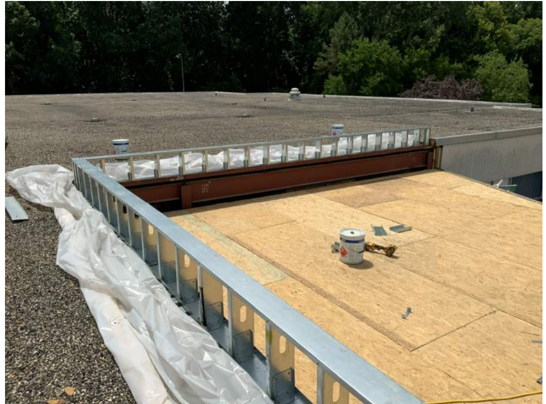
Parapet framing and tectum roof panels are in place for canopy at the new secured entrance addition
