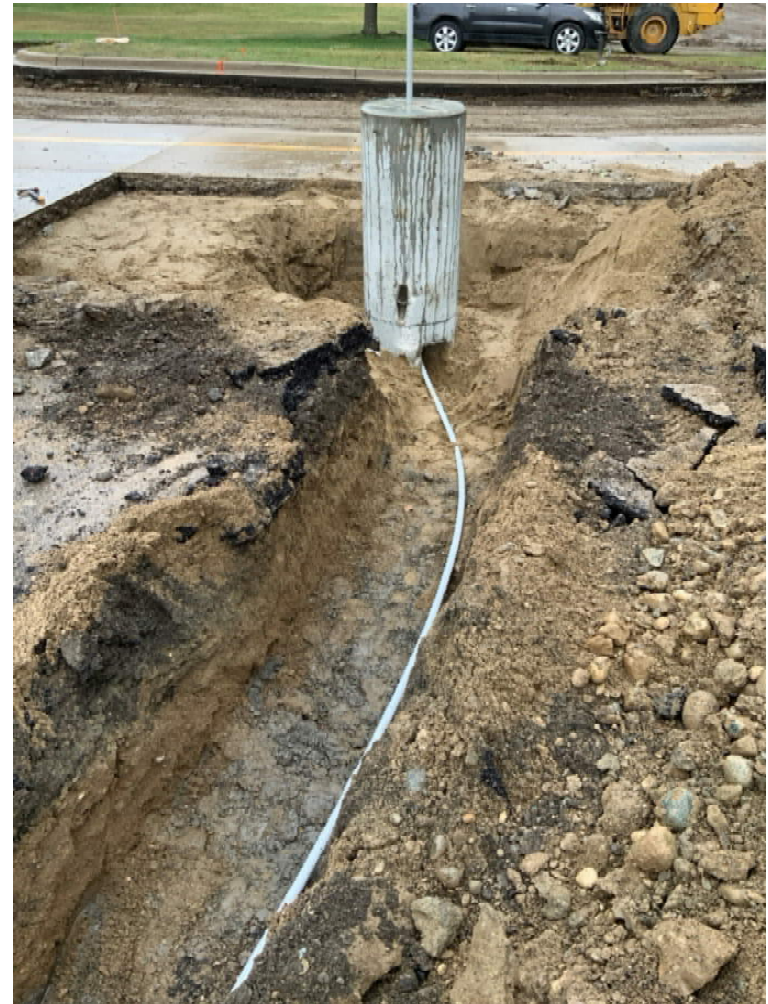
New light pole base and underground conduit for power cable
