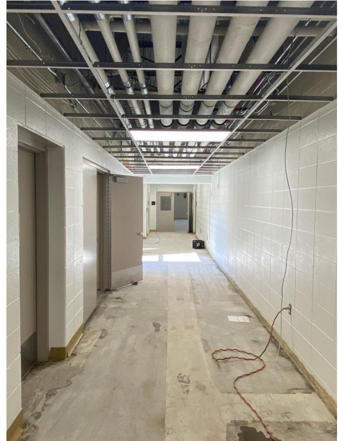
Flooring and ceilings removed in corridors
