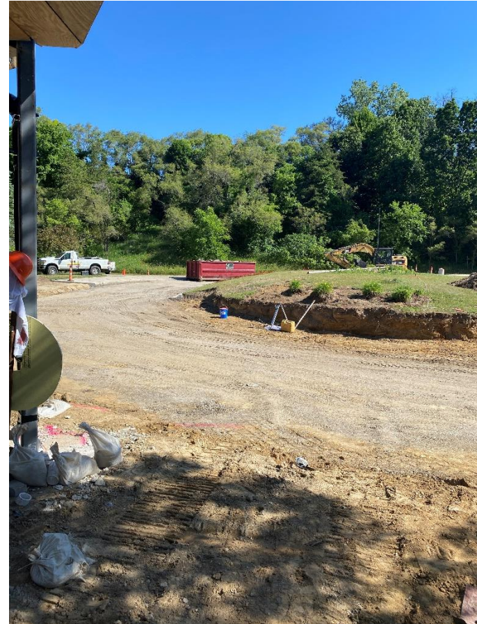
Existing asphalt removed and prepped for new base course.
