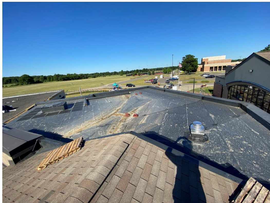
New roof on the secured entry
