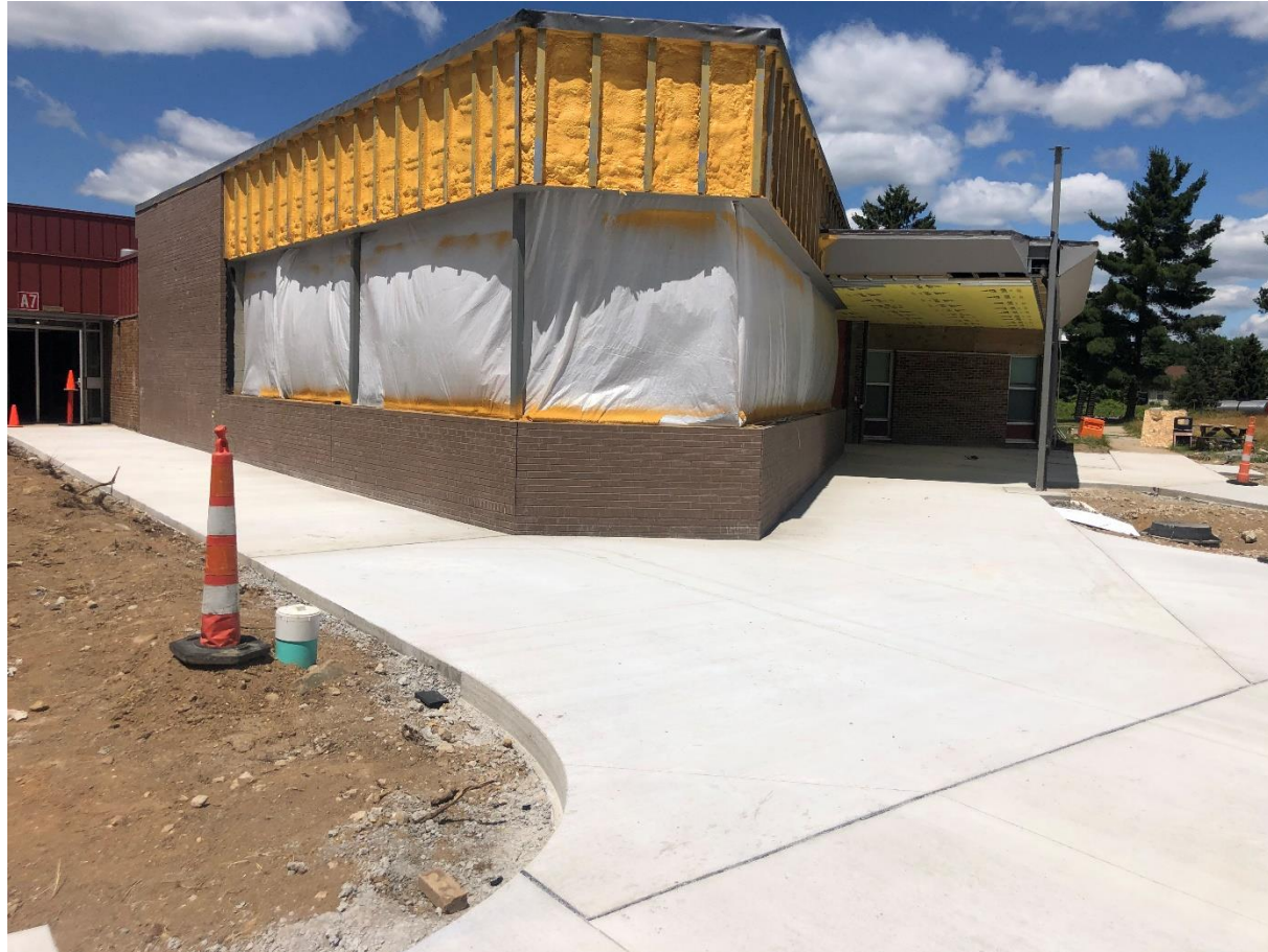
New sidewalks poured at secured entry
