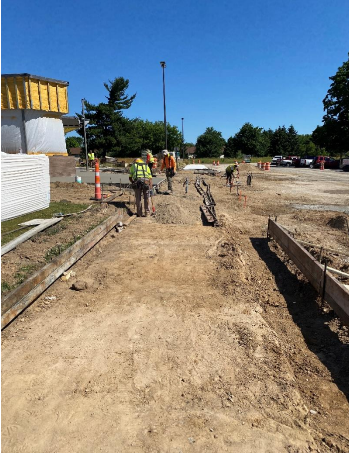
Secured entry sidewalks being formed.
