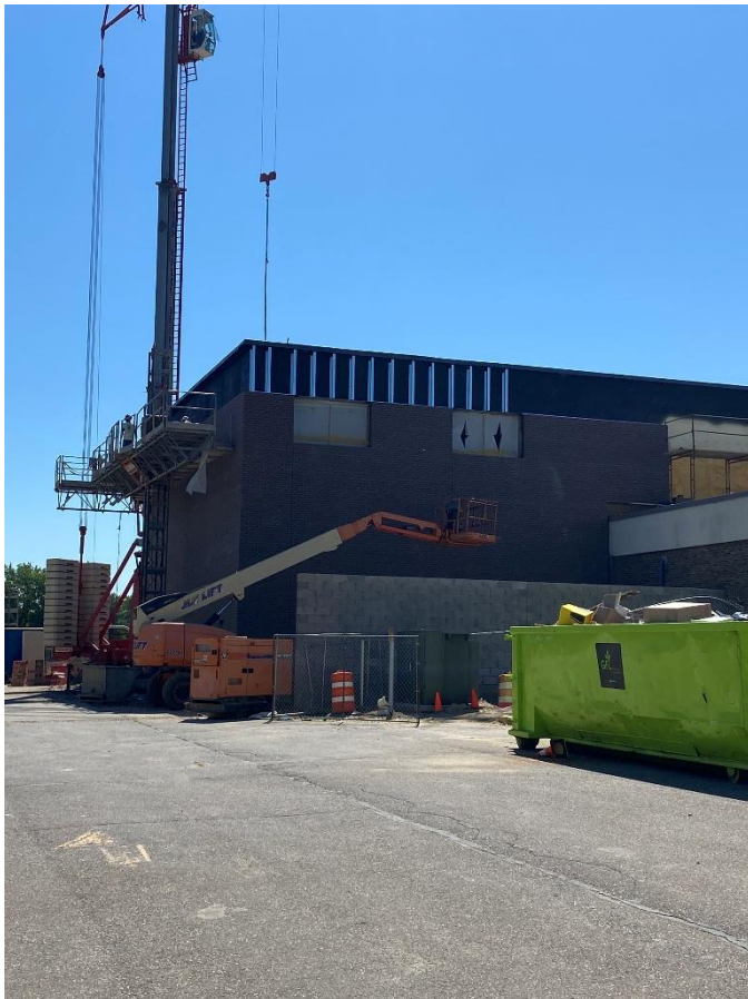
Gym addition masonry progressing and z-girts being installed.
