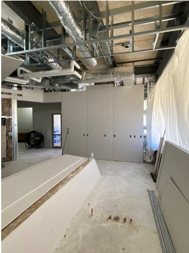
Drywall being hung in the new secured entry addition reception area.
