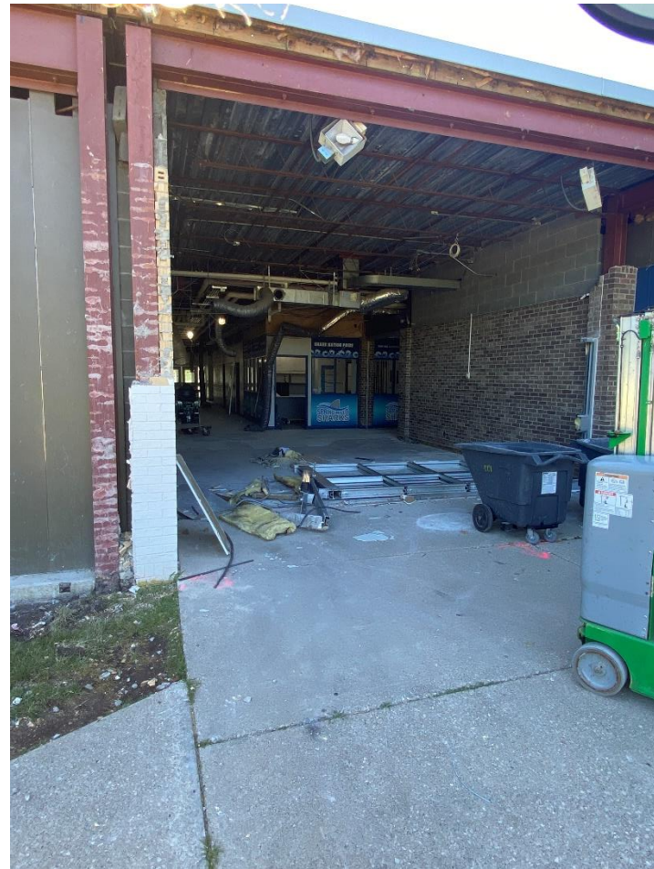
Old entry removed and prepping for new secured entry.
