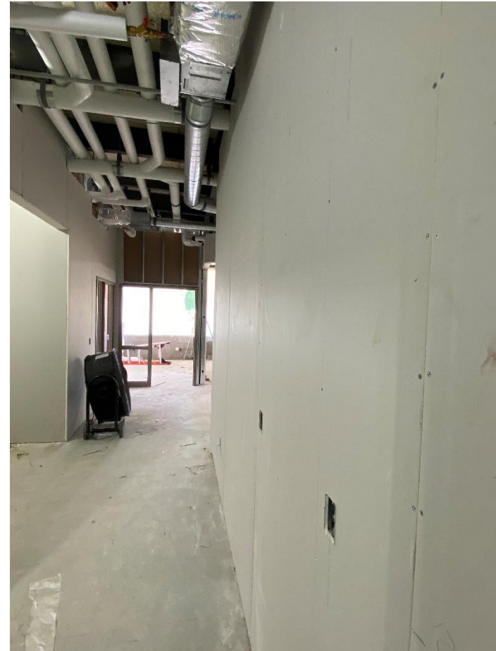
Drywall hung in new office area of secured entry addition
