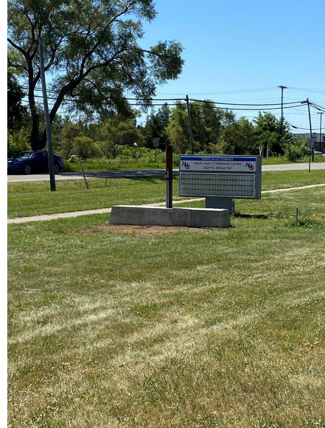
New sign foundation poured
