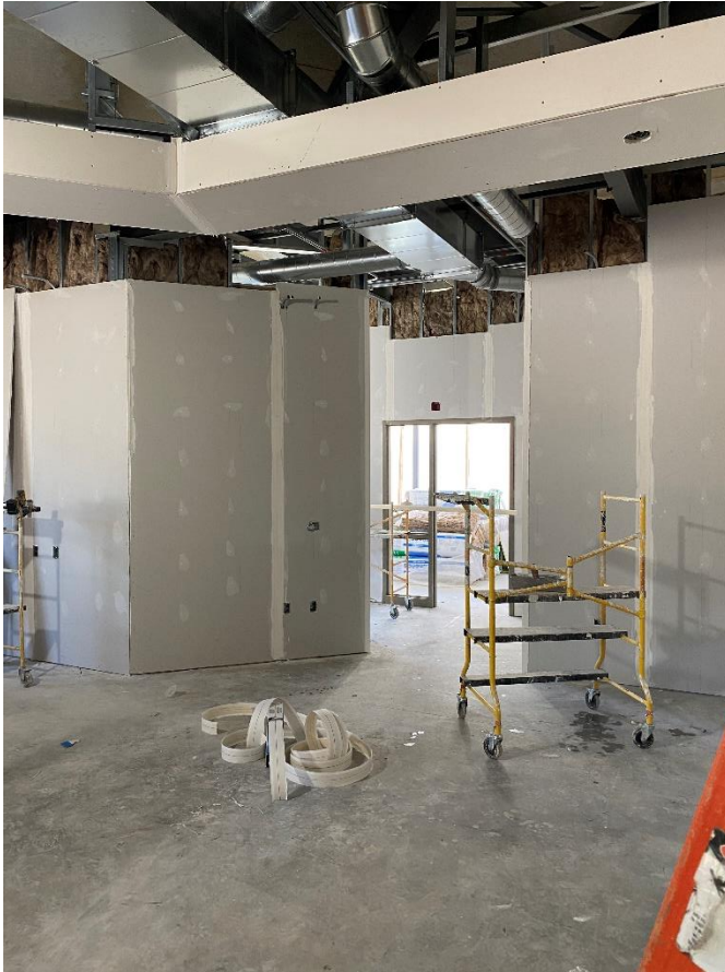
Drywall installation on going.
