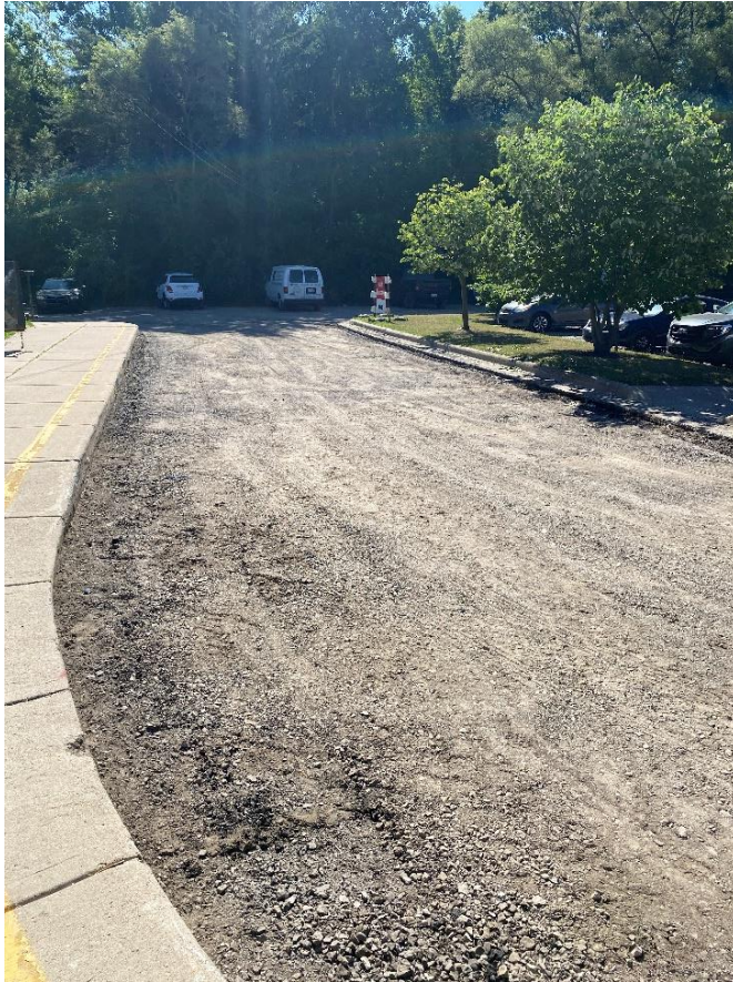
Existing asphalt removed and prepped for new base course.
