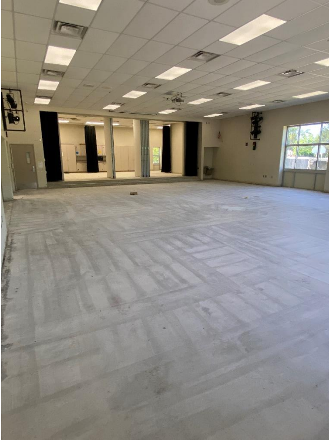
Old floors removed in the multipurpose room
