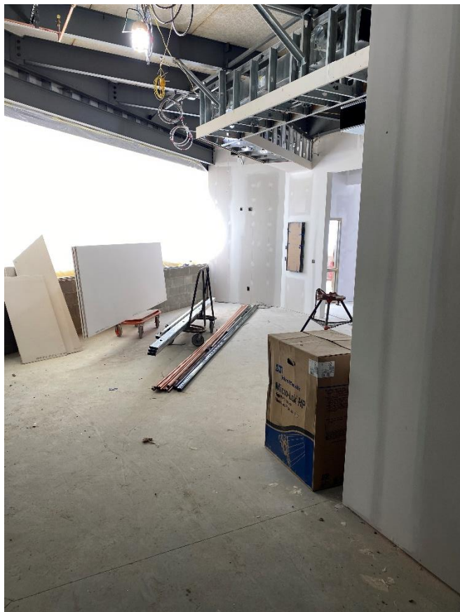
Drywall prep for paint on going at secured entry office area
