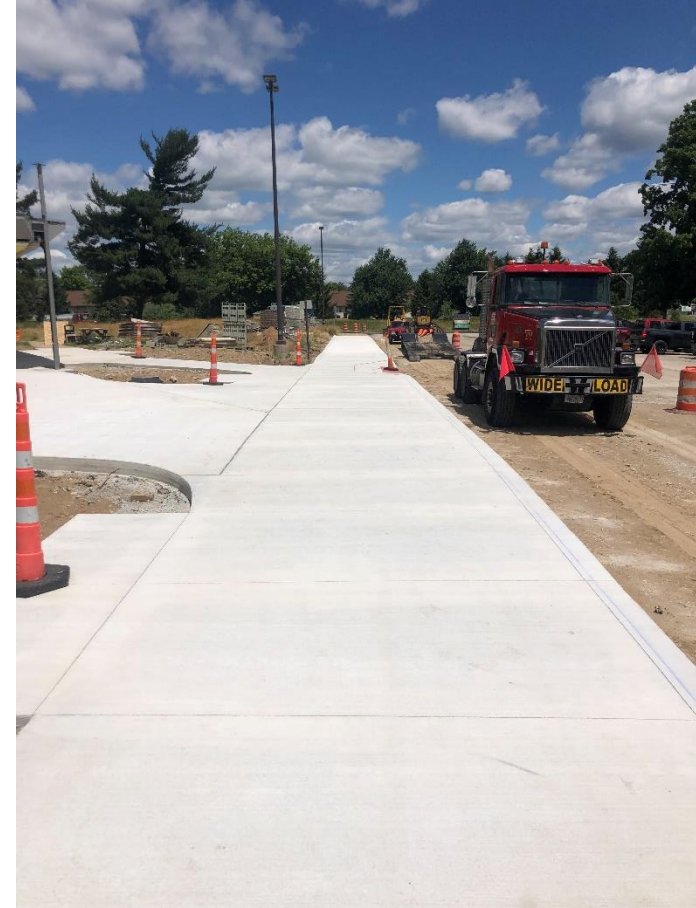
New sidewalks poured at secured entry
