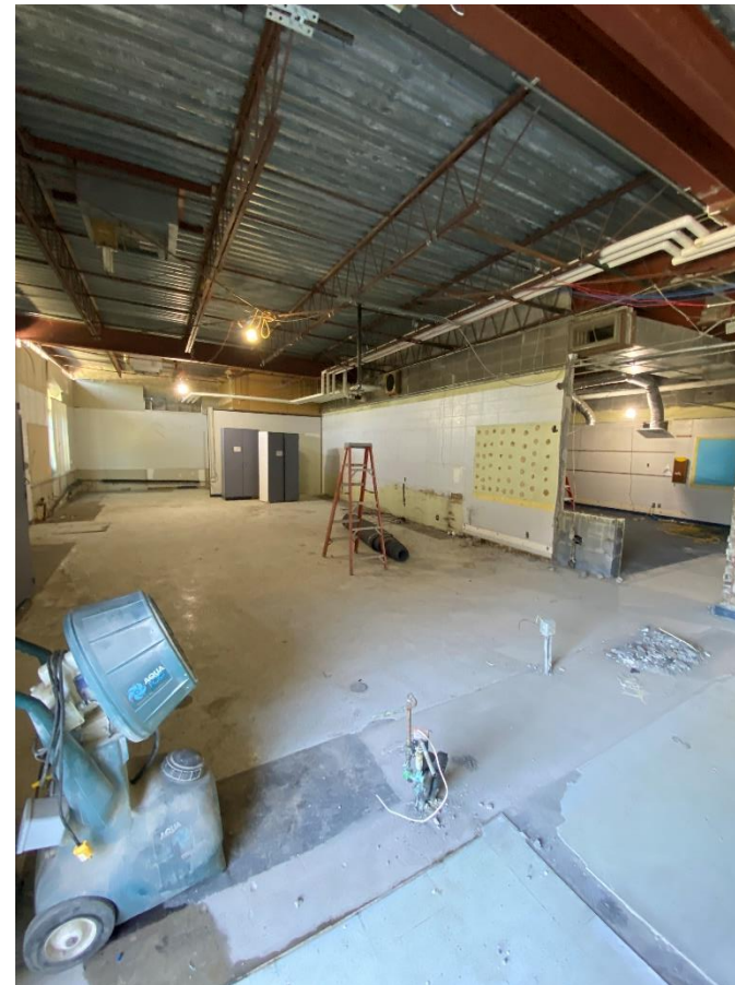
Demo on going in new secured entry area.
