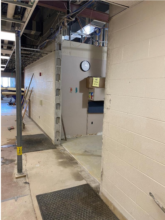
New opening in the masonry wall
