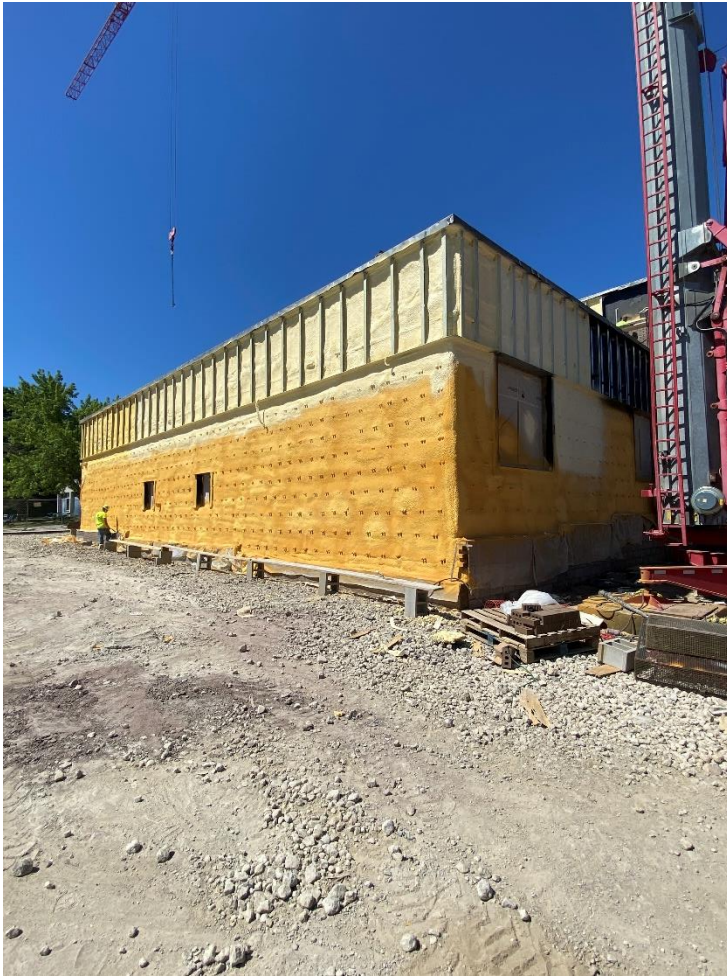
Spray foam completed on classrooms and brick starter courses being laid.
