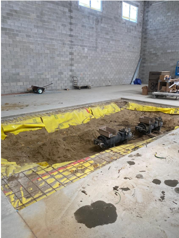
Old chiller dismantled and removed.
