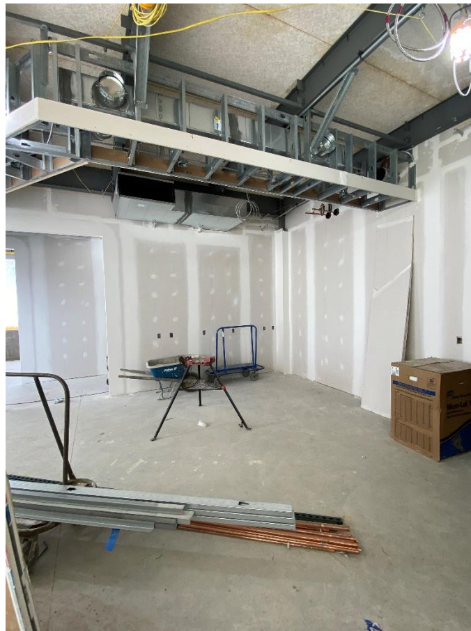
Drywall prep for paint on going at secured entry reception area.
