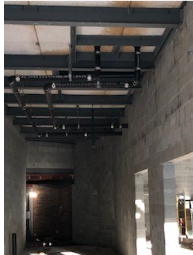
Roof sumps and piping being installed
