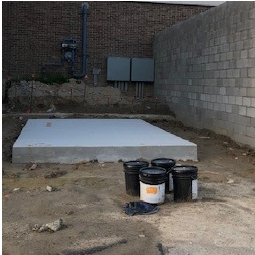
New equipment pad for new chiller poured
