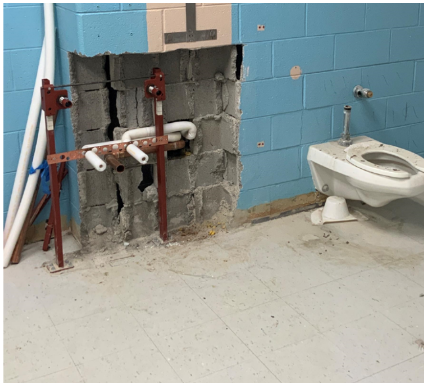
Interior toilet room new sink carrier and rough plumbing installed
