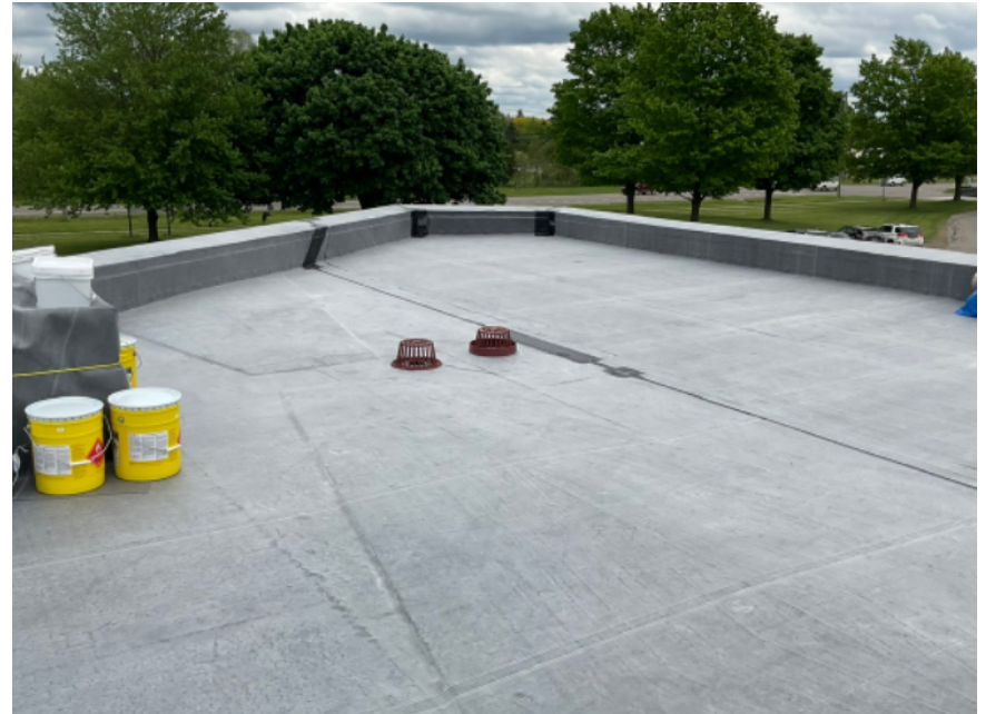
EPDM roofing installed on secured entry addition.
