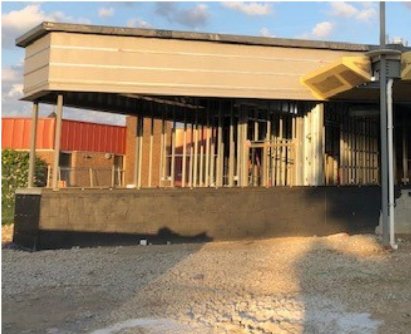
Installation of damp proofing prepped for spray foam insulation.
