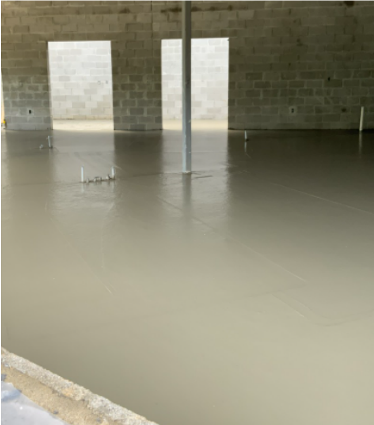
Slab on grade poured at secured entry addition
