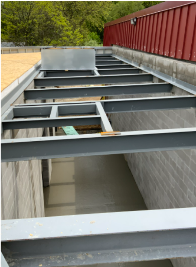
Curb for new RTU is Set and concrete in corridor poured
