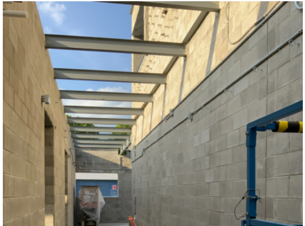
Above ceiling electrical rough in is on-going.
