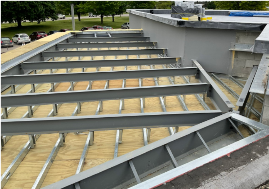
Canopy Roof prepped and ready for Tectum Deck.
