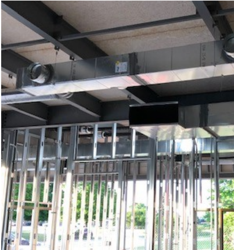
HVAC duct work being installed
