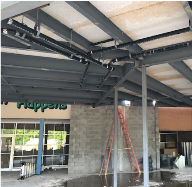
Roof sumps and piping being installed
