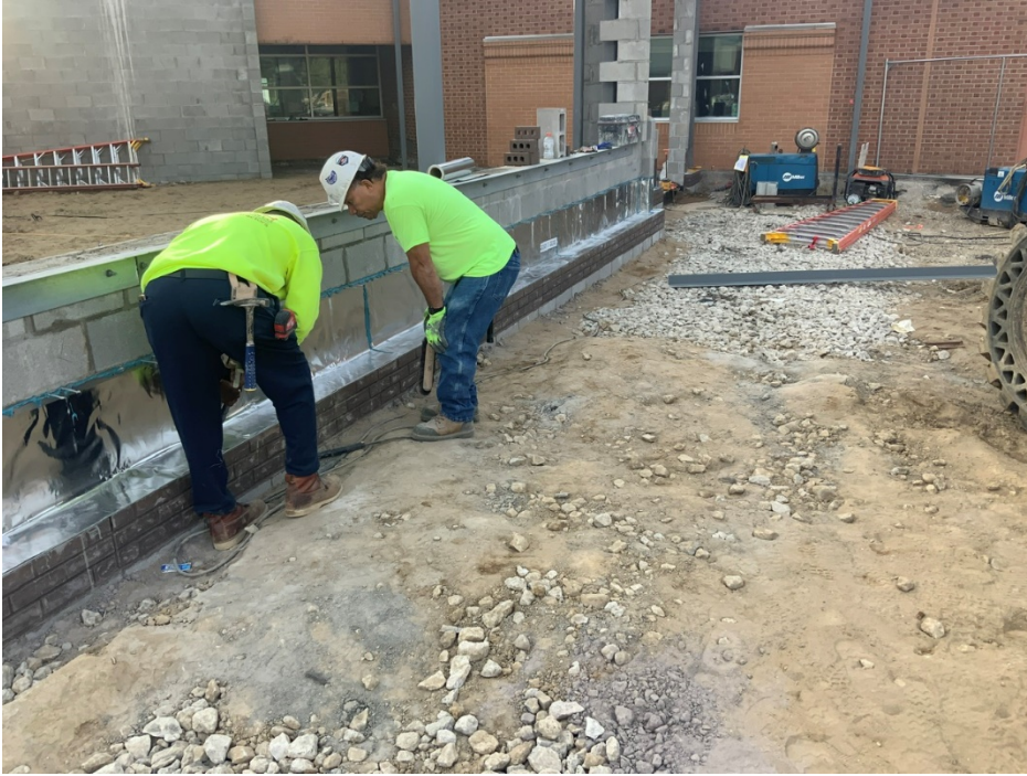
Masonry thru-wall flashing being installed
