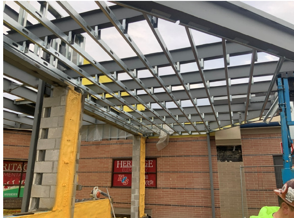
Cold formed metal framing for canopy soffit is complete
