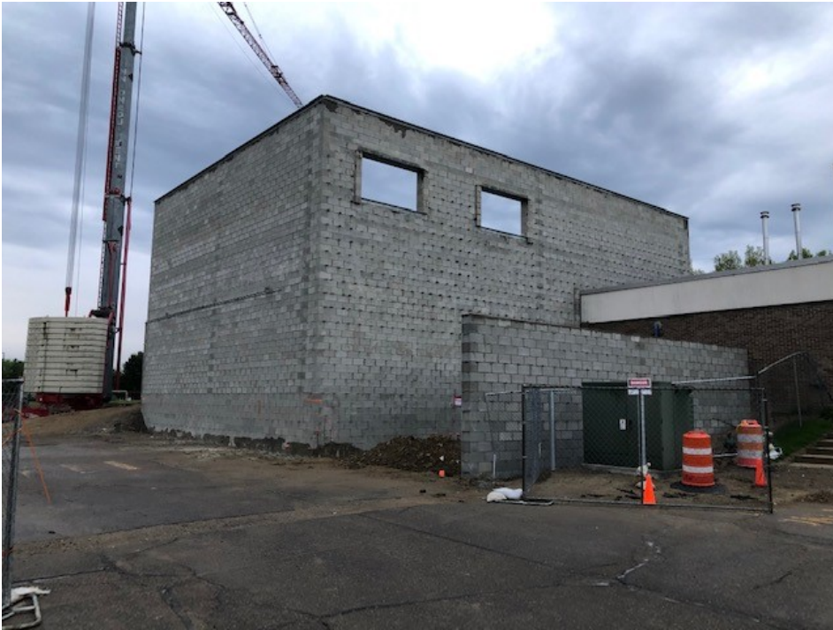
North and west CMU walls for the new gymnasium is complete.
