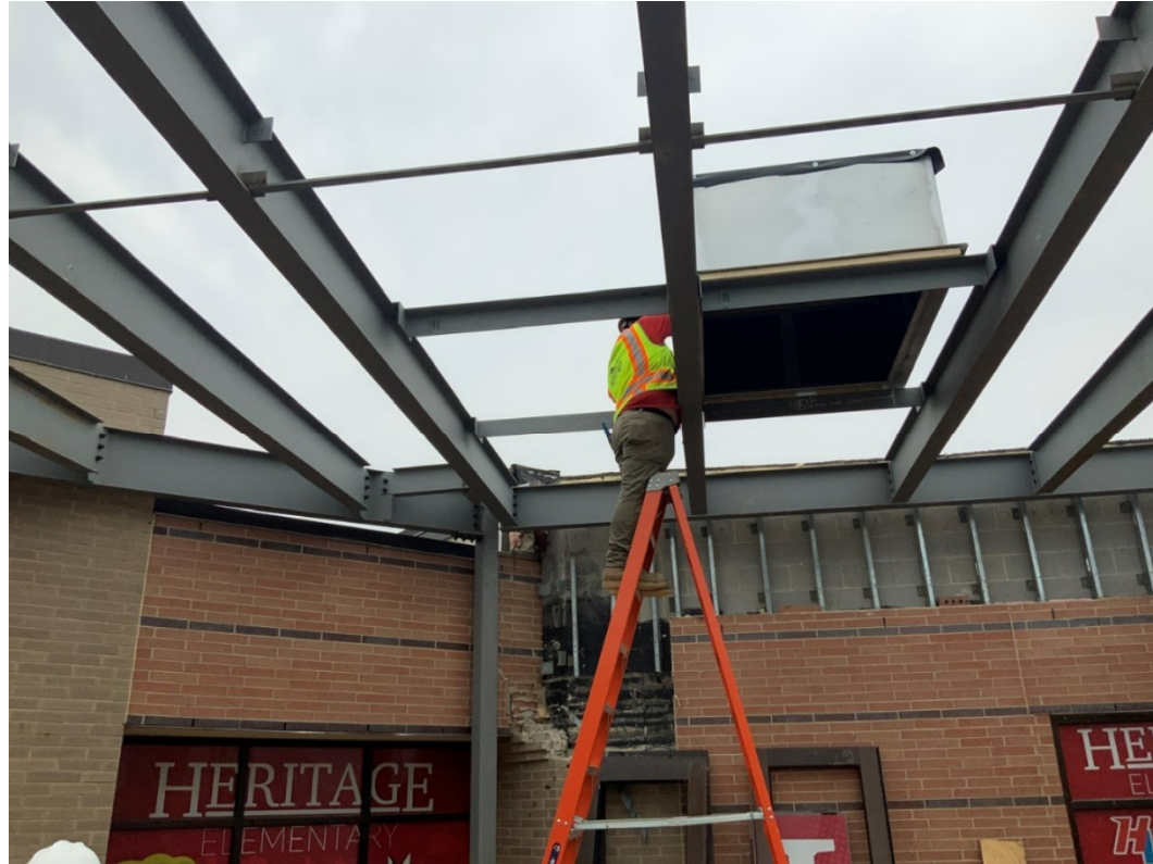
Curb for new rooftop air handling unit is set
