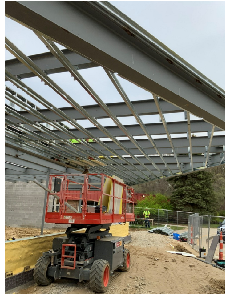
Cold formed metal framing has been installed for entrance canopy
