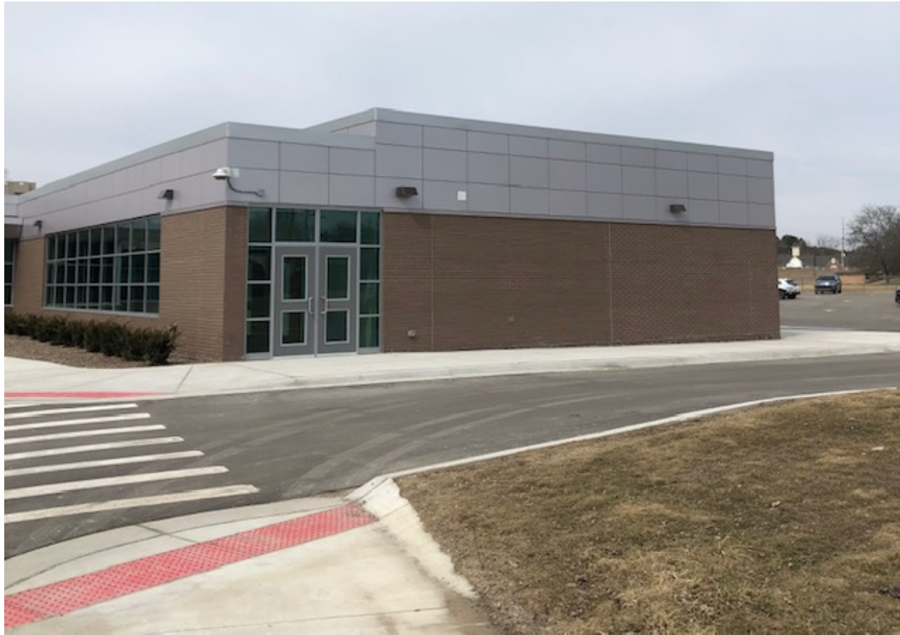
Completed Installation of Metal Panels, Flashings, Spire Cap and Scupper
