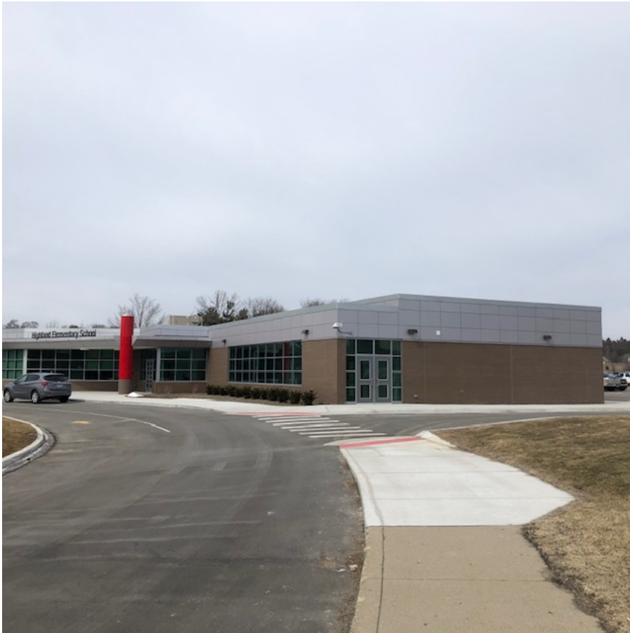
Completed Installation of Metal Panels, Flashings, Spire Cap and Scupper
