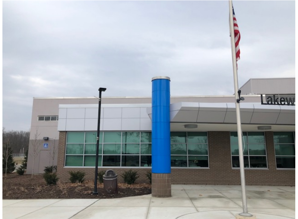
Completed Installation of Metal Panels, Flashings, Spire Cap and Scupper
