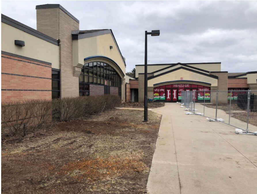
Secured Entry Addition – Trees Removed Adjacent to Existing Main Entrance
