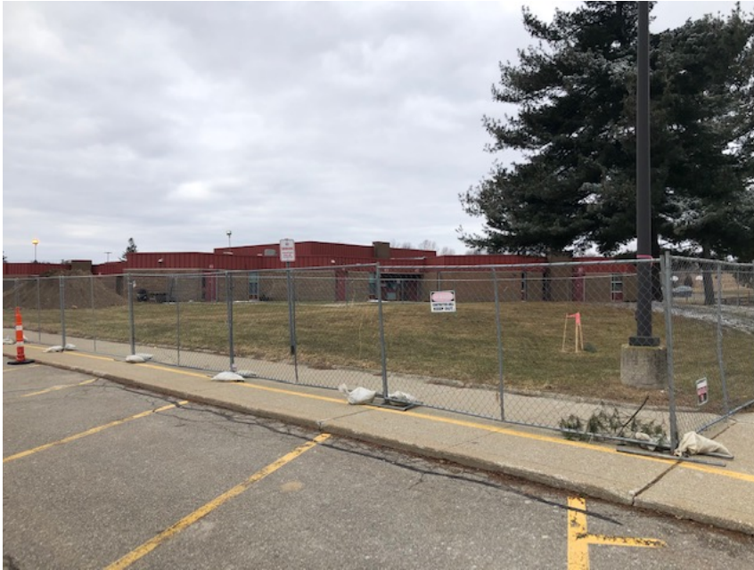
Secured Entry Addition – Temporary Fencing Around Staging Area
