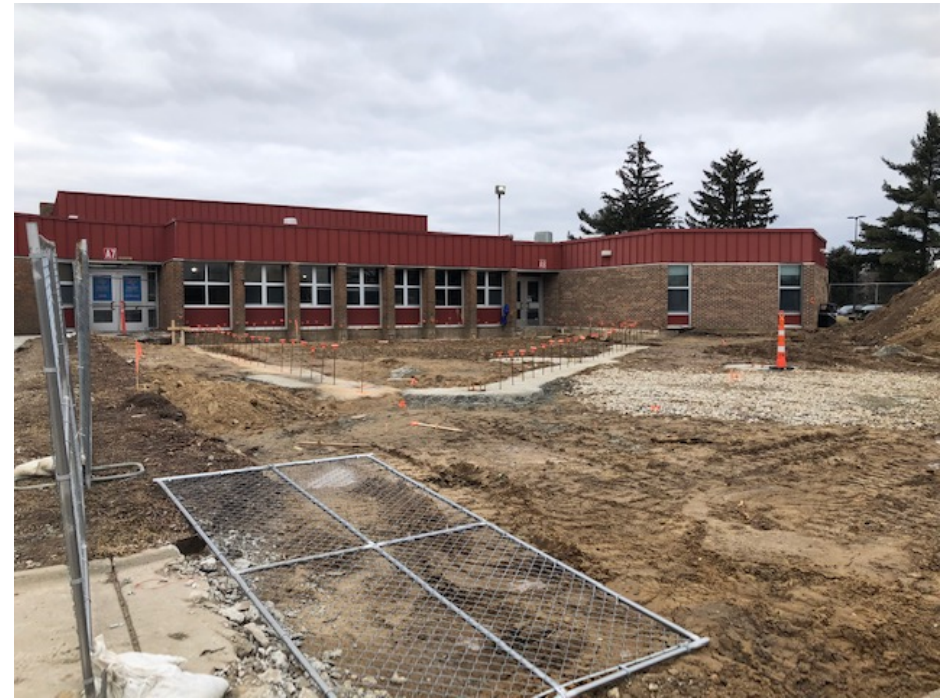
Secured Entry Addition – Site Clearing Complete
