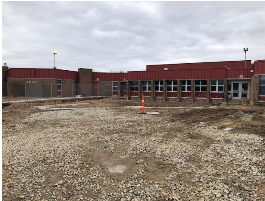
Secured Entry Addition – Foundations Complete
