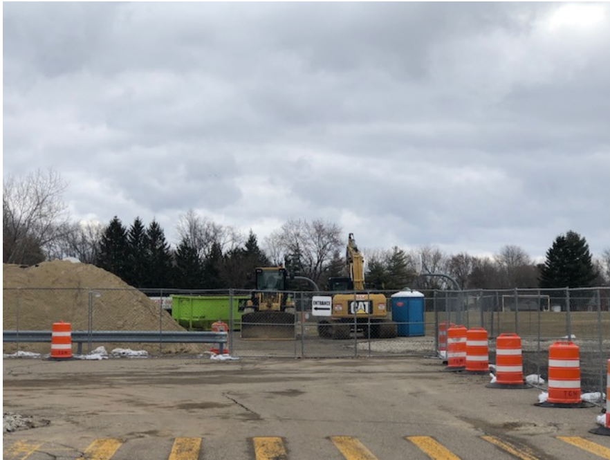
Gymnasium & Classroom Addition – Temporary Fencing to Secure Material and Equipment Staging Area is in Place and Sand Material Has Been Delivered
