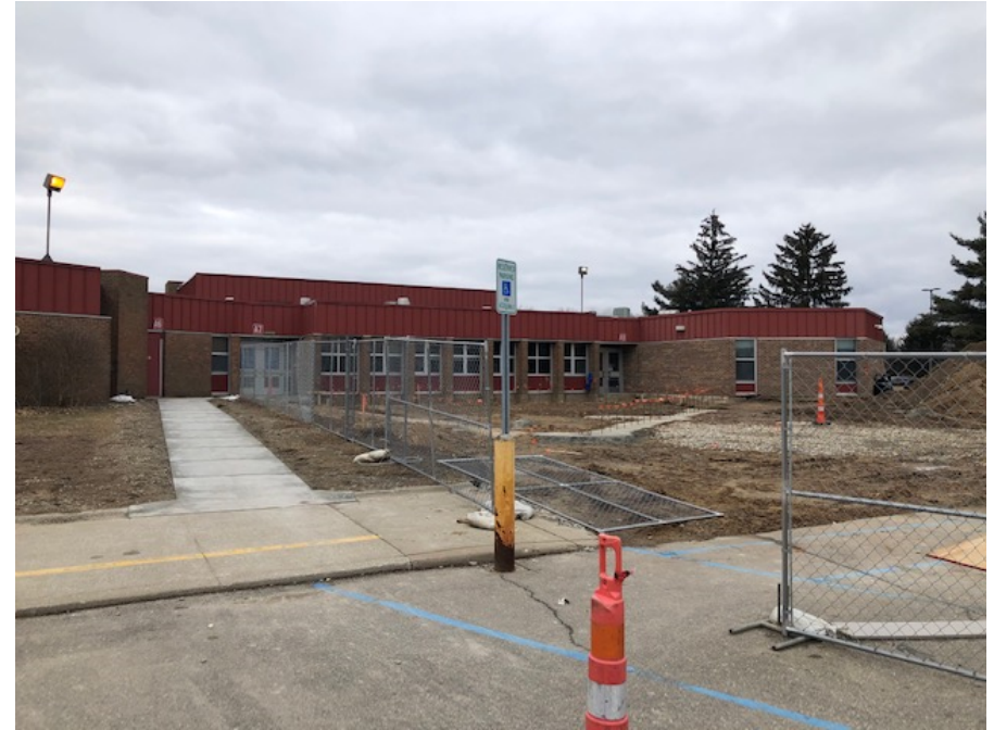
Secured Entry Addition – Temporary Sidewalk in Place for Emergency Egress
