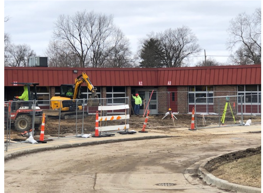
Secured Entry Addition – Site Clearing is Complete, and Foundations are Underway
