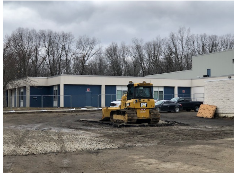
Gymnasium & Classroom Addition – Building Pad After Site Clearing
