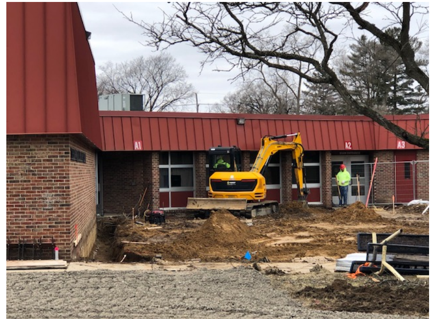
Secured Entry Addition – Excavation for Foundations is Underway
