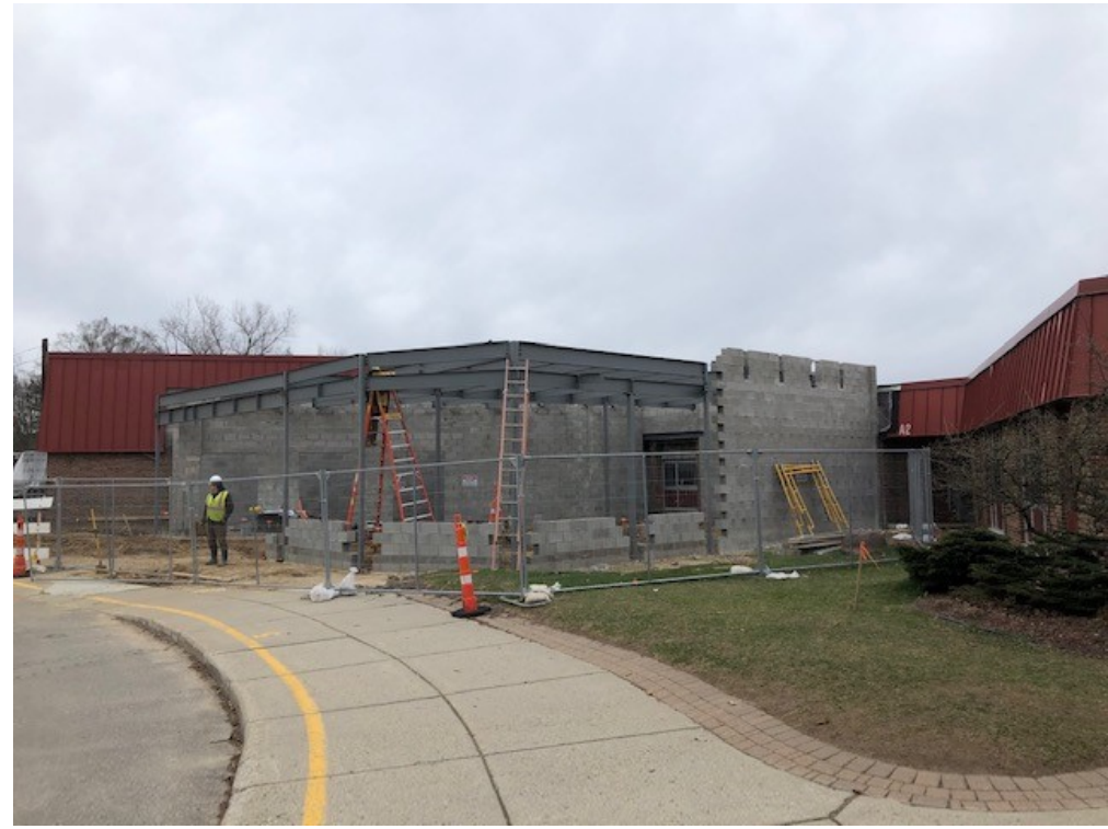
Steel erection is nearly complete for Secured Entry Addition
