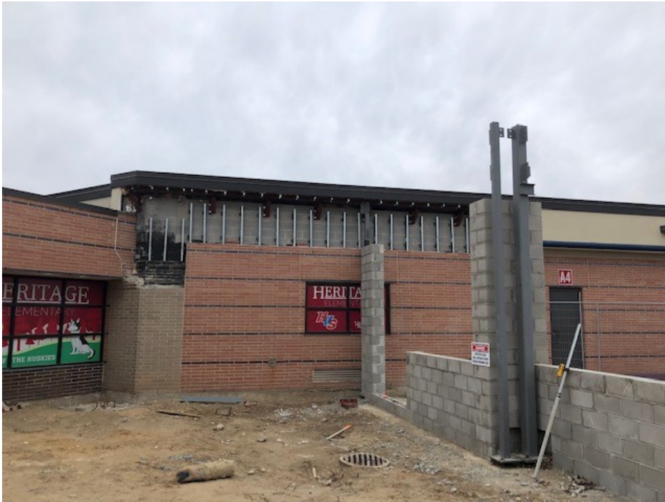
Masonry walls are partially complete and steel erection has started.
