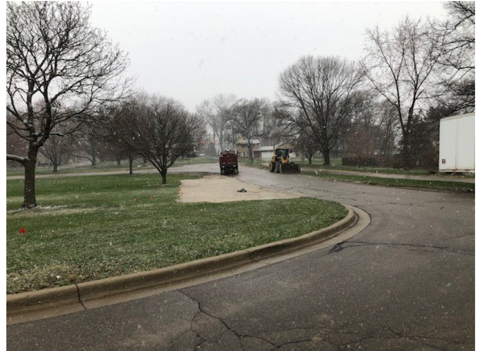
Temporary parking spaces added on north side of drop off loop for staff
