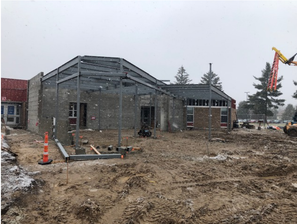
Steel erection is underway
