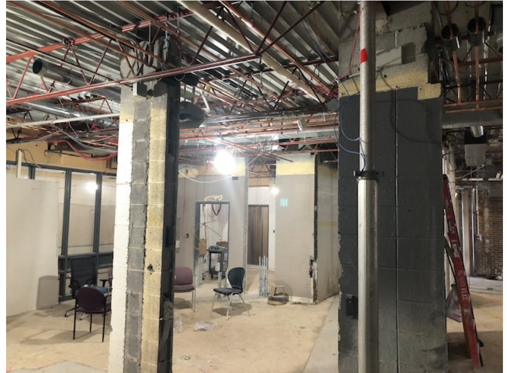
Interior renovations adjacent to the secured entrance addition are underway
