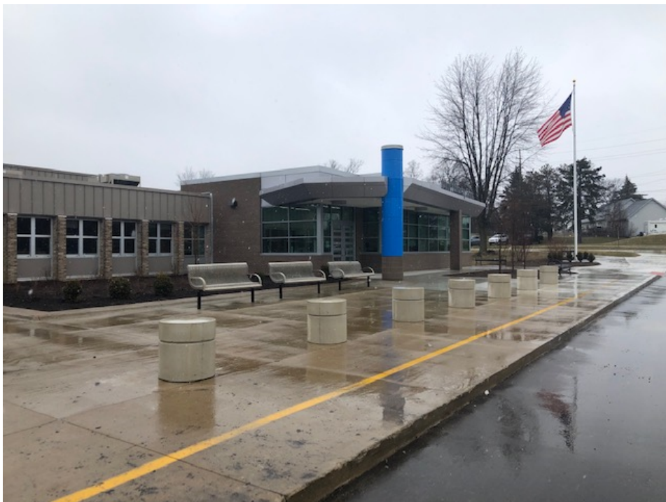
Bollards and Benches are installed
