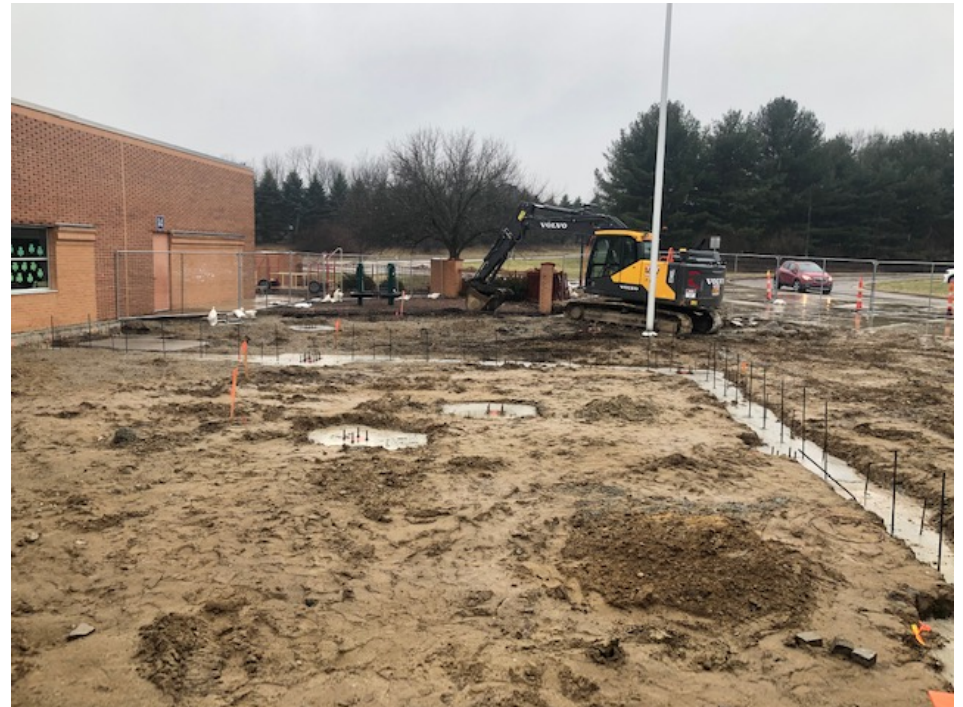
Foundations are complete for secured entrance addition
