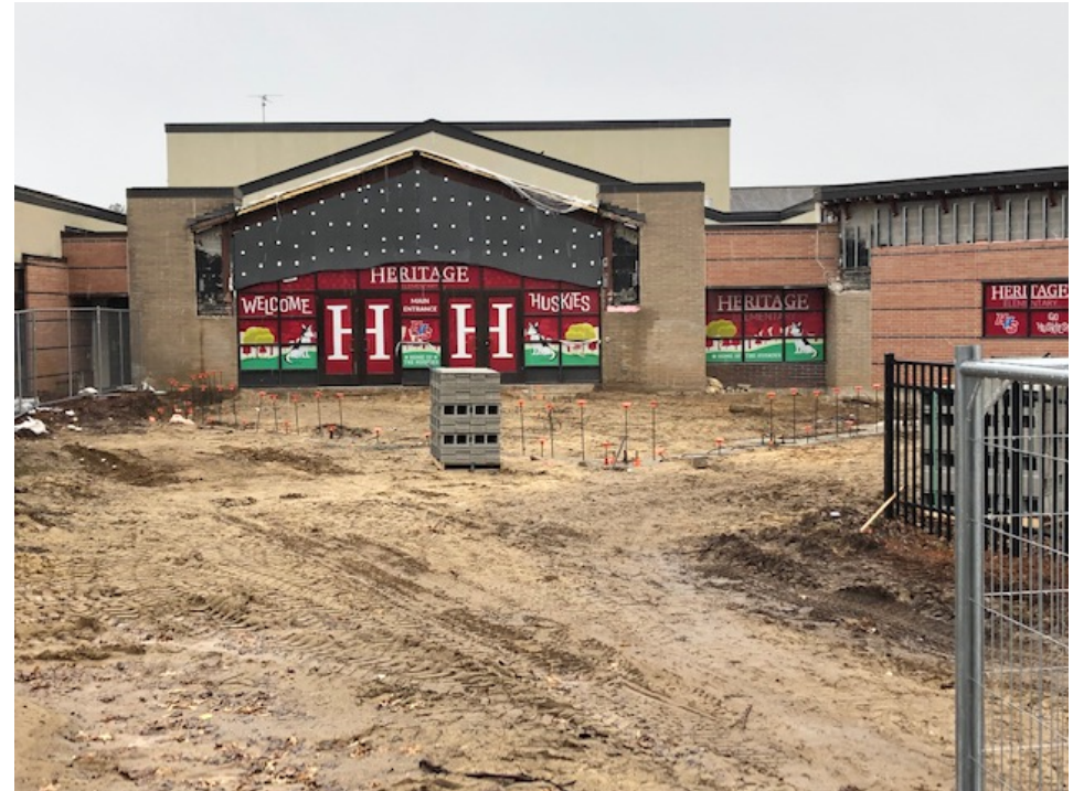
Foundations are complete for secured entrance addition
