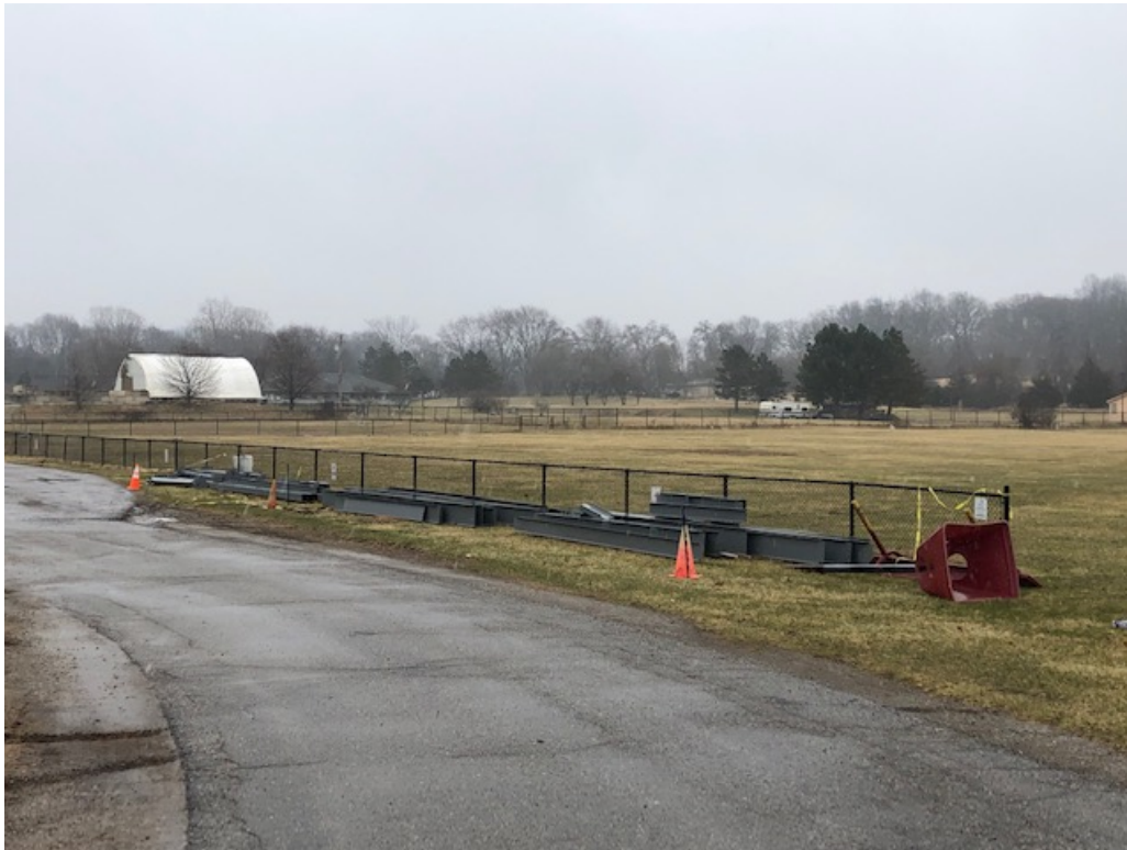
Structural Steel has been delivered
