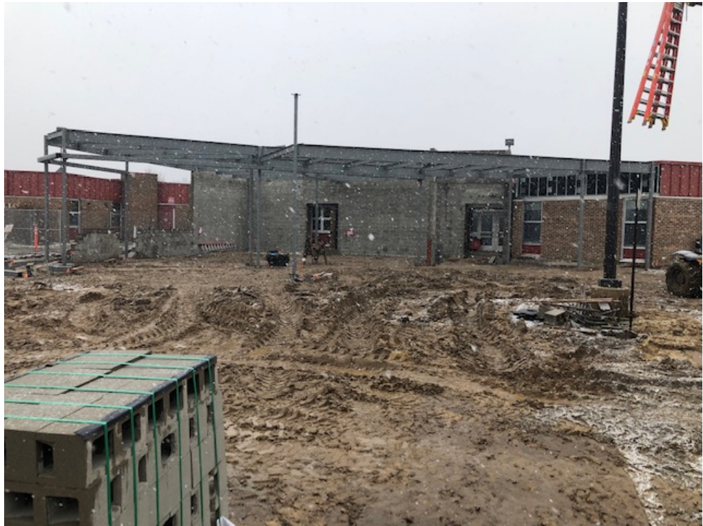
Steel erection is underway
