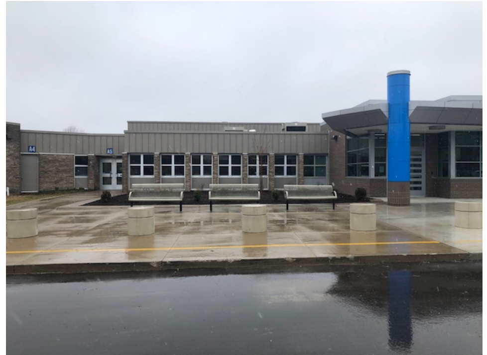
Bollards and Benches are installed
