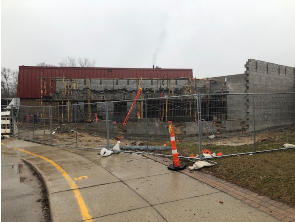
Masonry is underway for secured entrance addition
