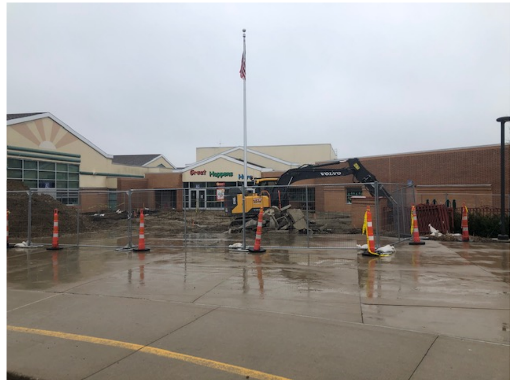
Foundations are complete for secured entrance addition
