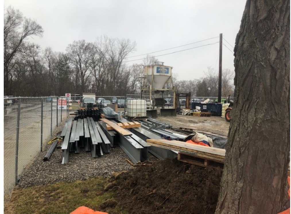
Structural Steel has been delivered
