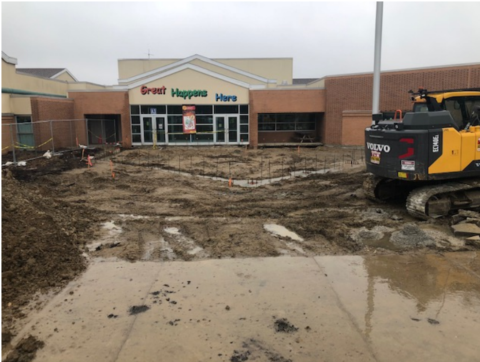
Foundations are complete for secured entrance addition
