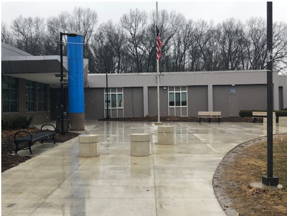
Bollards and Benches are installed
