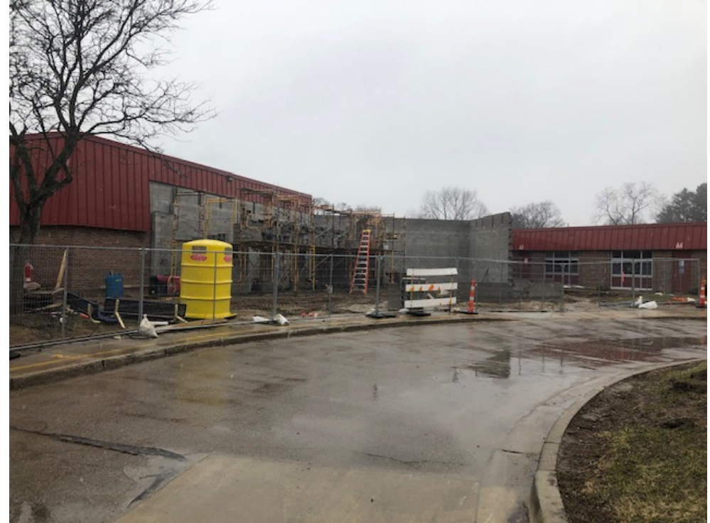
Masonry is underway for secured entrance addition
