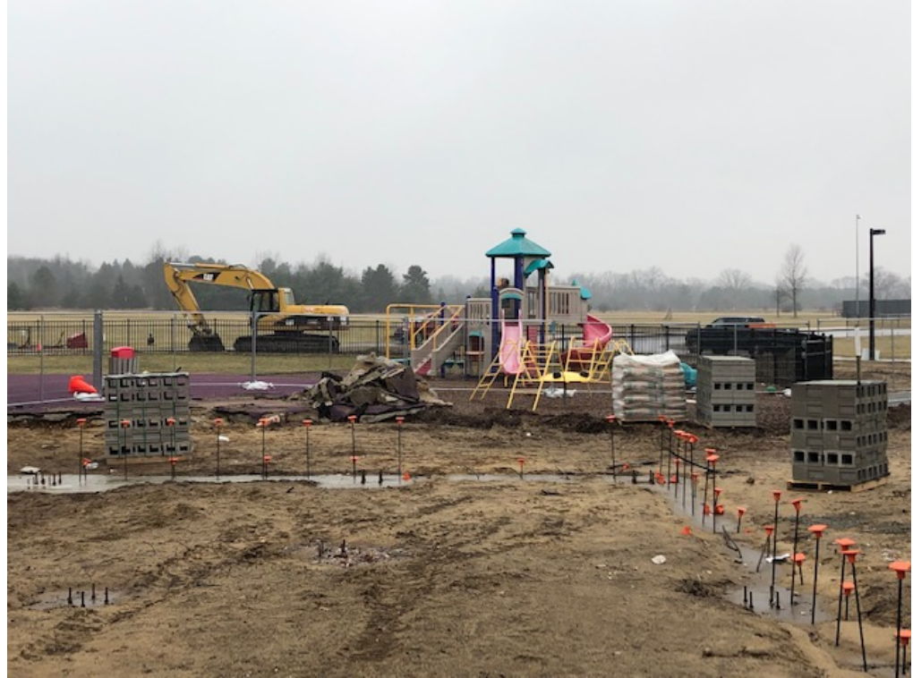
Foundations are complete for secured entrance addition
