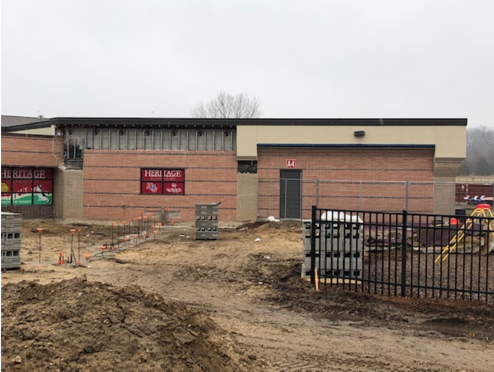
Foundations are complete for secured entrance addition
