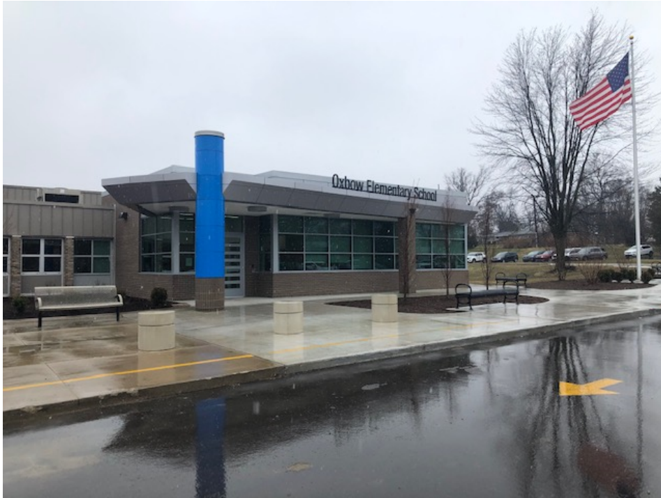
Bollards and Benches are installed
