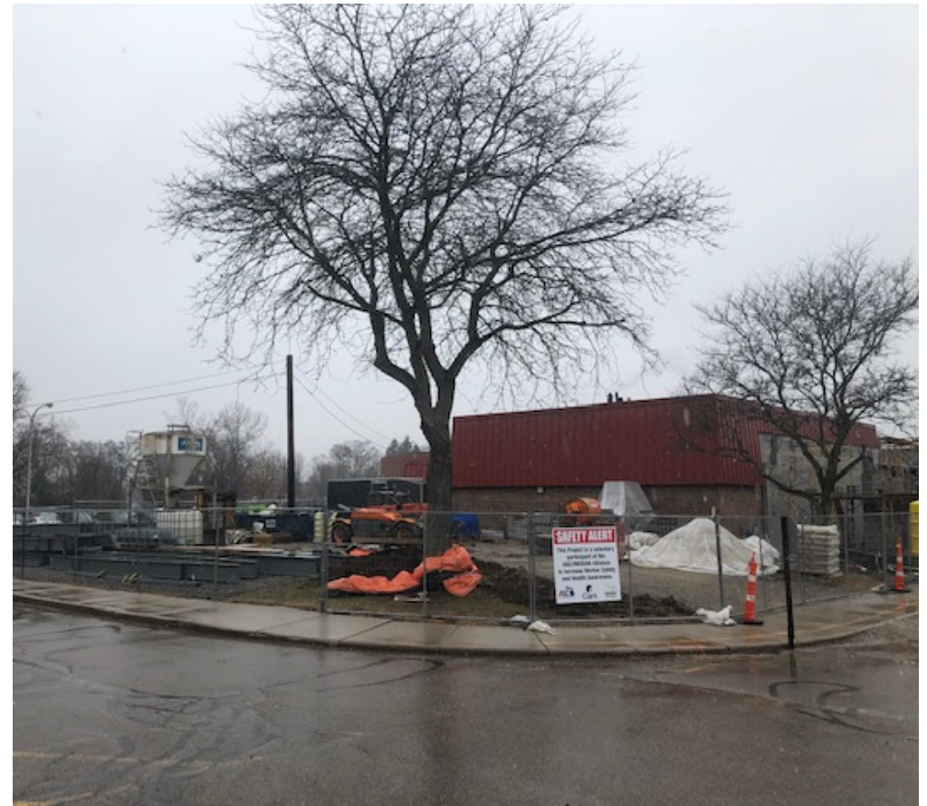
Structural Steel has been delivered
