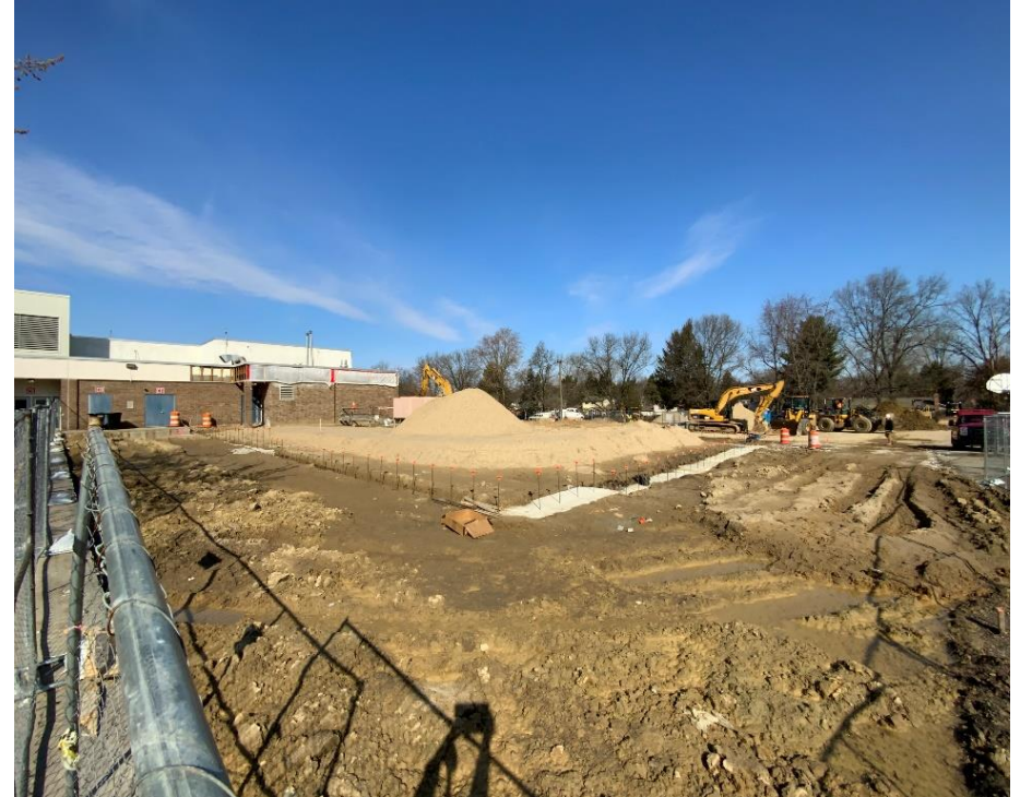
Gymnasium & Classroom Addition – Building Pad After Site Clearing
