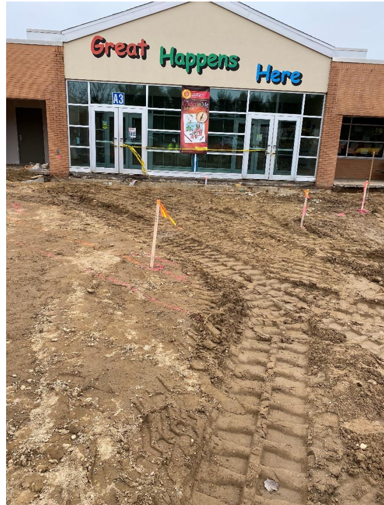
Secured Entry Addition – Site demolition is complete, foundations are staked.
