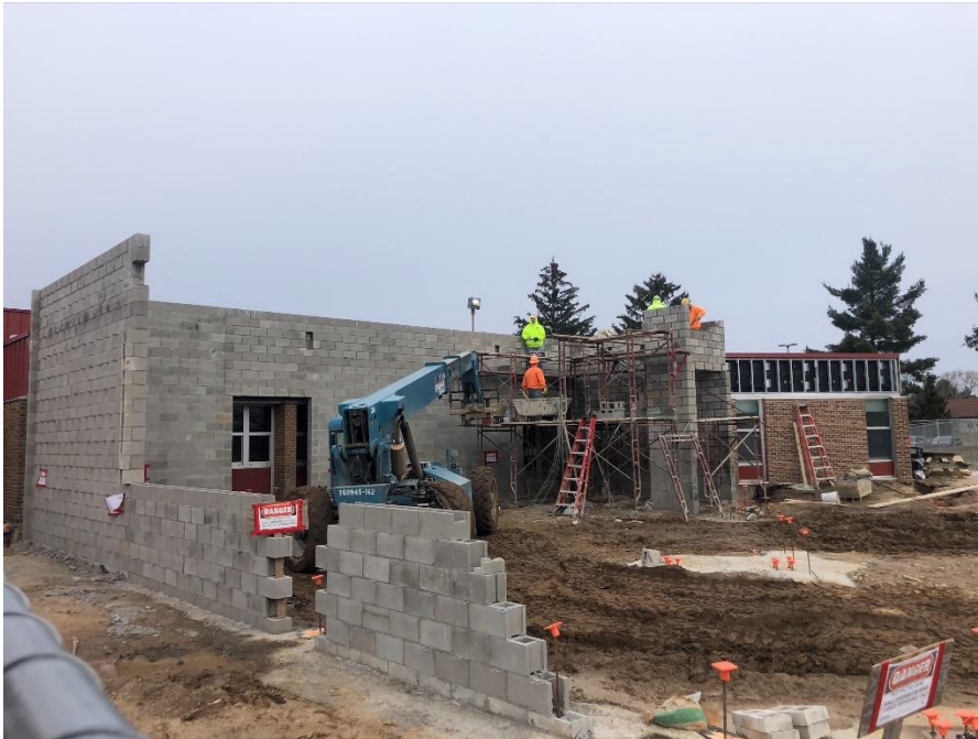
Secured Entry Addition – Masonry walls are underway.
