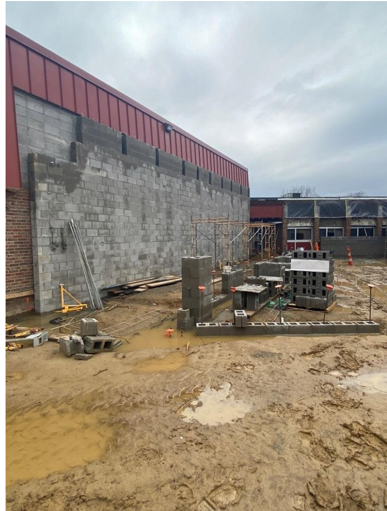
Secured Entry Addition – Masonry walls are ongoing.
