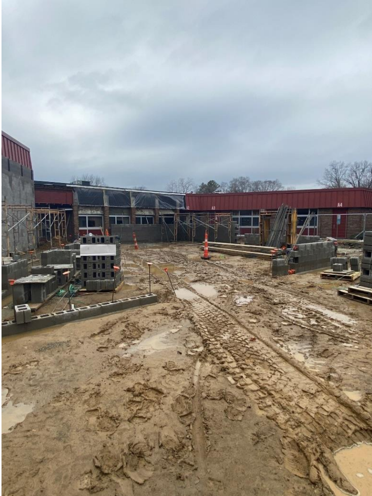
Secured Entry Addition – Masonry walls are ongoing.
