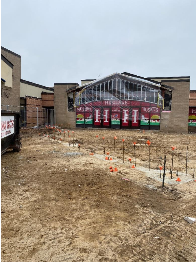
Secured Entry Addition – Foundations are poured, existing exterior removed.
