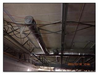
**Figure (10)** – HVAC duct above Room 4 covered with polyethylene sheeting.
