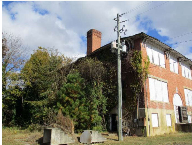
3. View of power pole and transformers on west side of main school building.
