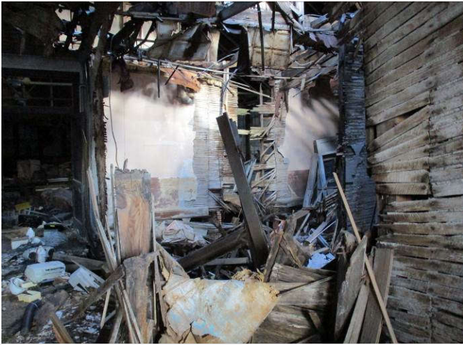
13. View inside the administration building.
