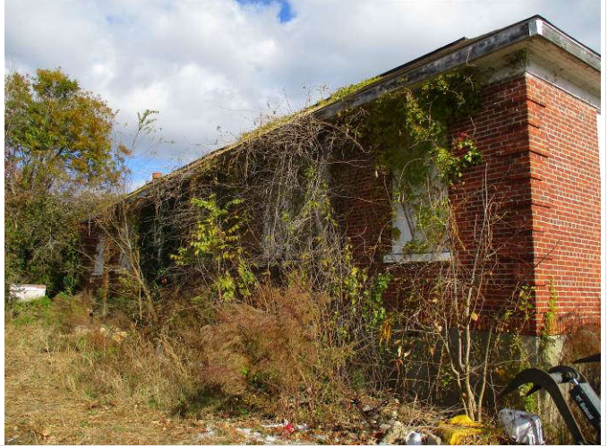
8. View west side of administration building.
