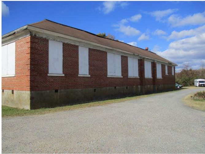
9. View east side of administration building.
