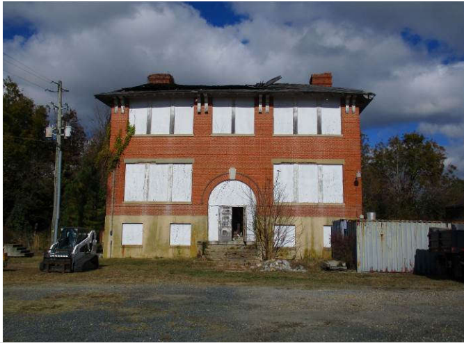
1. View south side of main school building.
