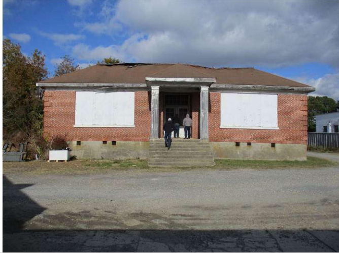
7. View south side of administration building.
