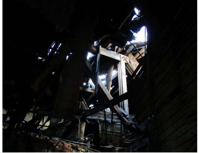
14. View inside the administration building.
