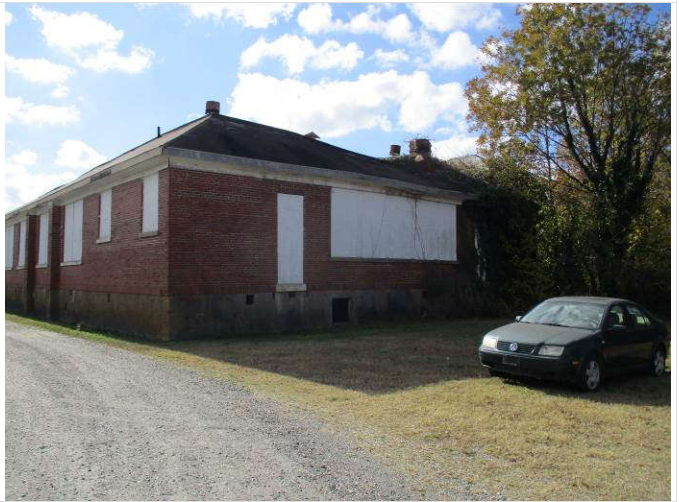
10. View north side of administration building.
