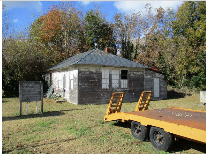
15. View of the dining room/kitchen building.
