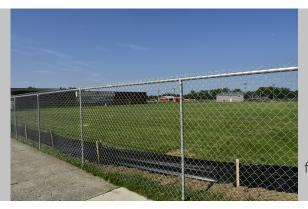
The black silt fencing around the perimeter helps to contain dust, debris, and sediment.
