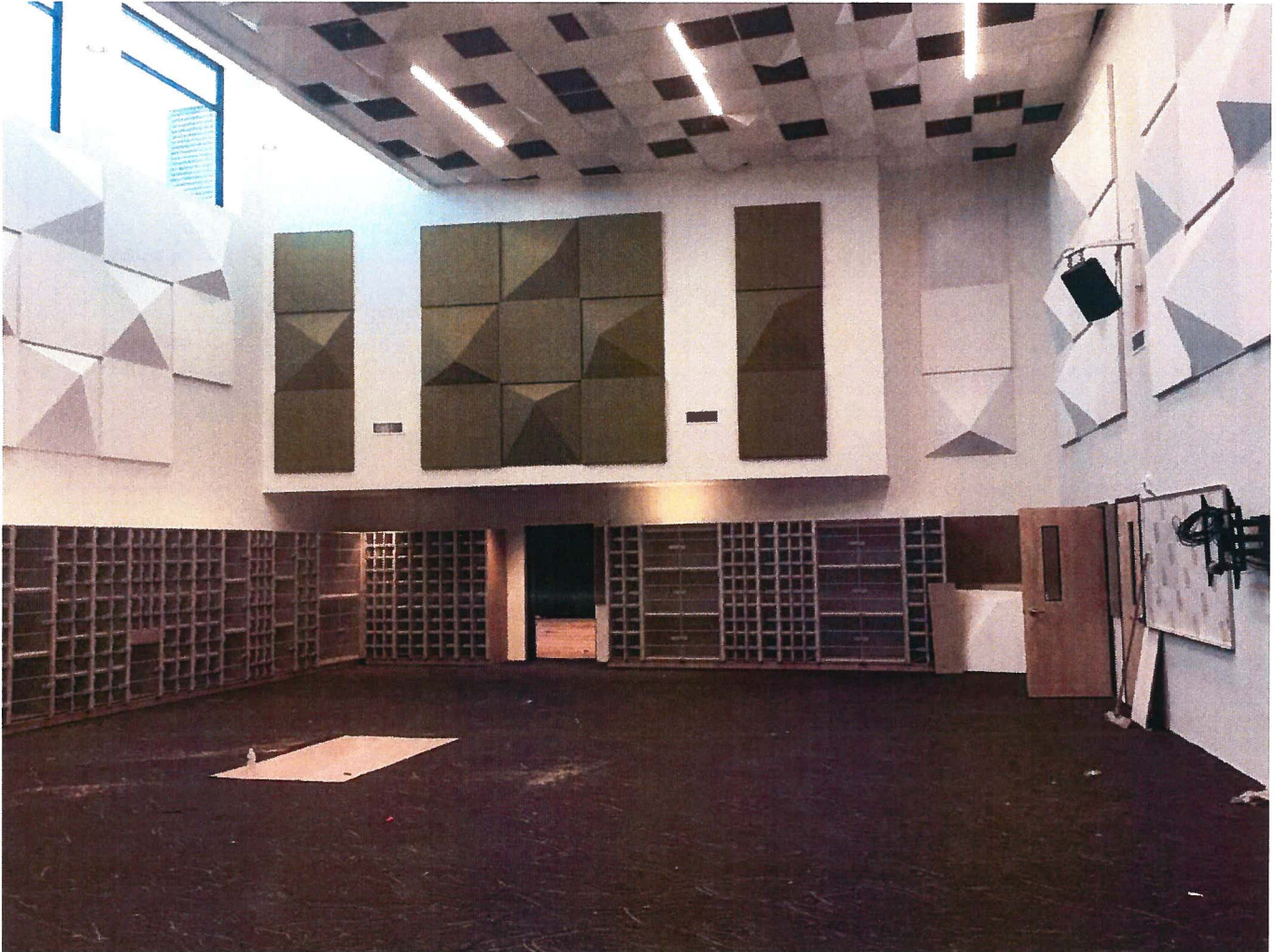
SRIS / VRMS – Band Room – All acoustical panels installed and instrument casework recently finished.
