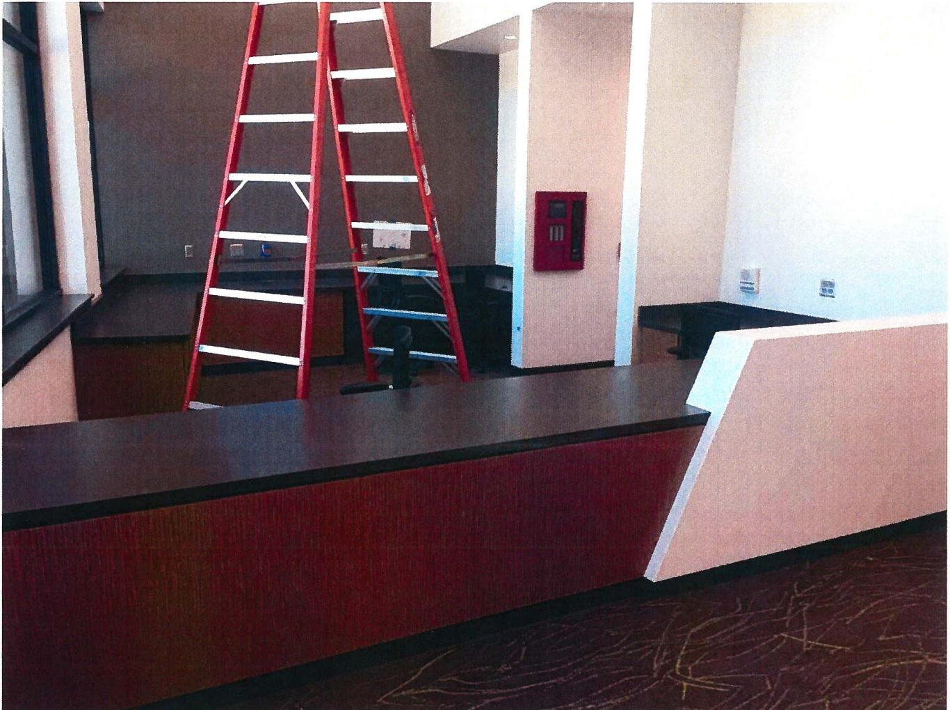
SRIS / VRMS – Front Office – casework installed and most furniture distributed.
