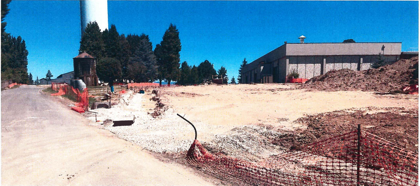
HIGH SCHOOL – Bus lane sub-grade being prepped
