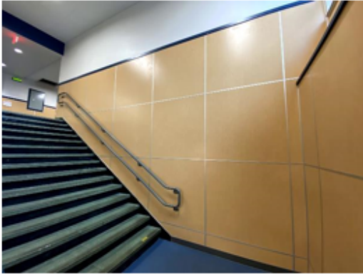
Stair wainscot installation complete
