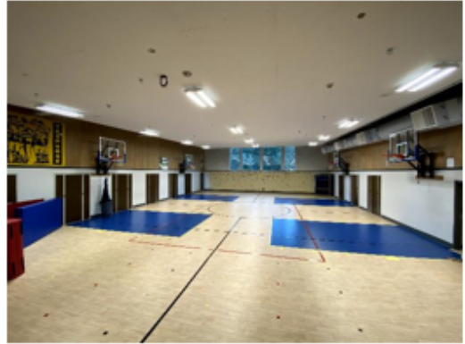
Gymnasium - new floor, new ceiling
