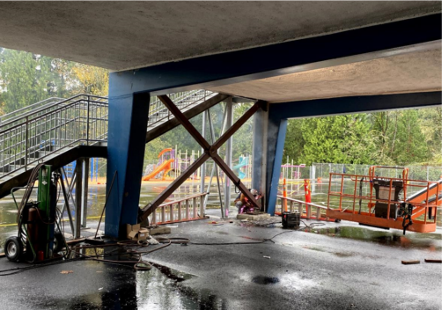
Seismic brace installation under gymnasium
