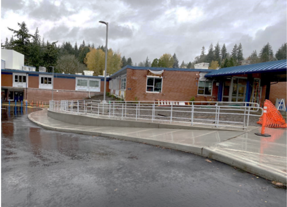
Handrail/Guardrail installation at ADA ramp underway
