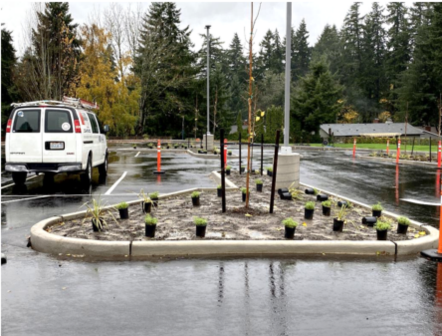
Landscape planting ongoing
