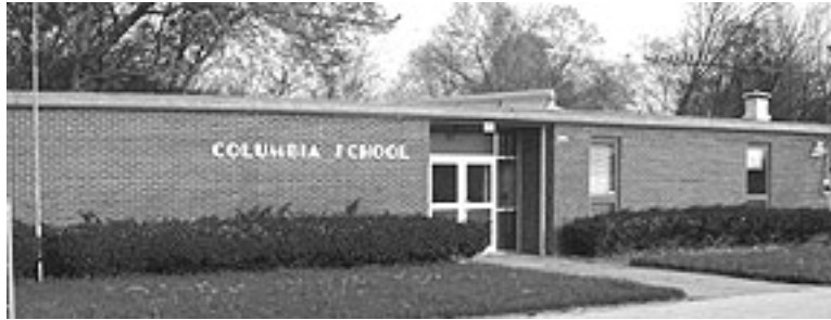
Columbia School on Spring Creek Road; currently unoccupied.
