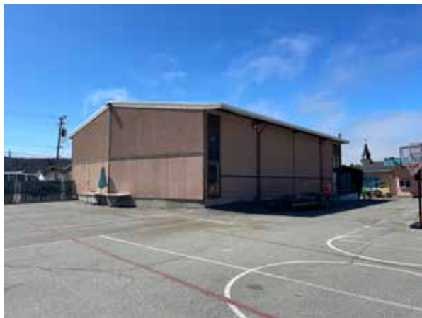
Paint building exteriors
