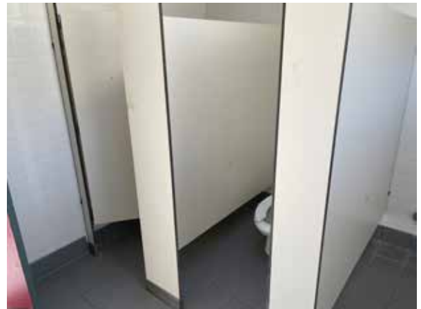
Remodel restroom building for ADA
