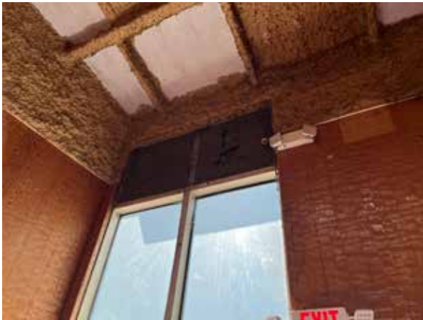
Resurface multipurpose interior
