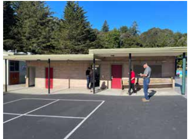
Remodel restroom building for ADA
