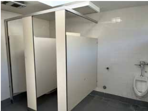
Remodel restroom building for ADA
