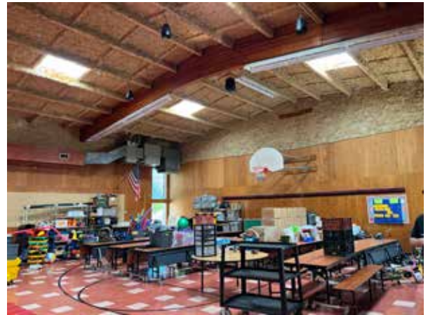
Resurface multipurpose interior
