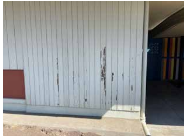
Paint building exteriors
