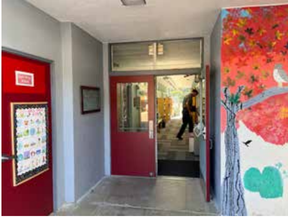
Replace doors and hardware
