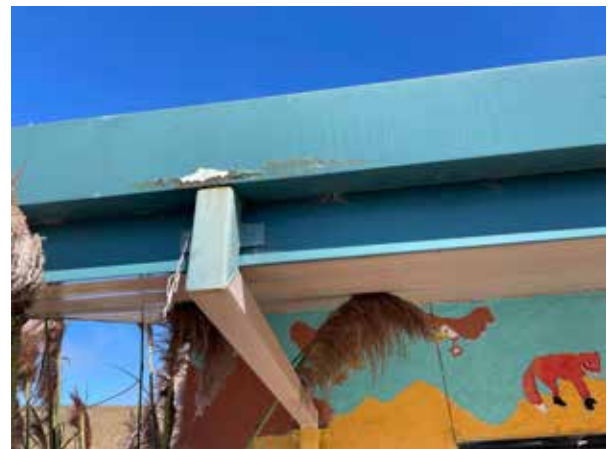
Paint building exteriors
