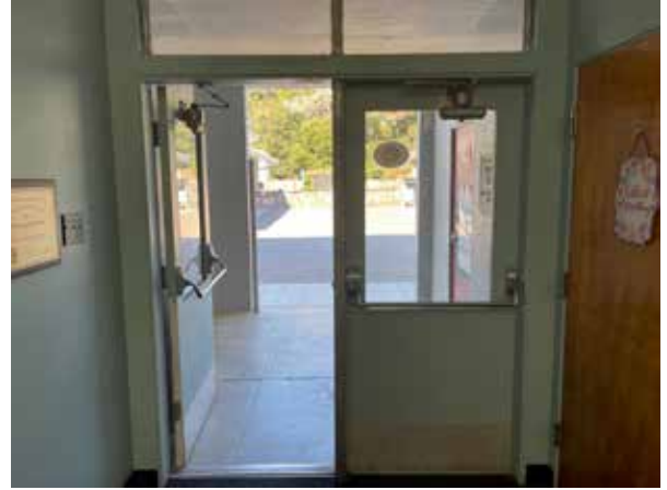
Replace doors and hardware
