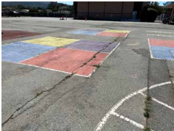
Repave asphalt flatwork
