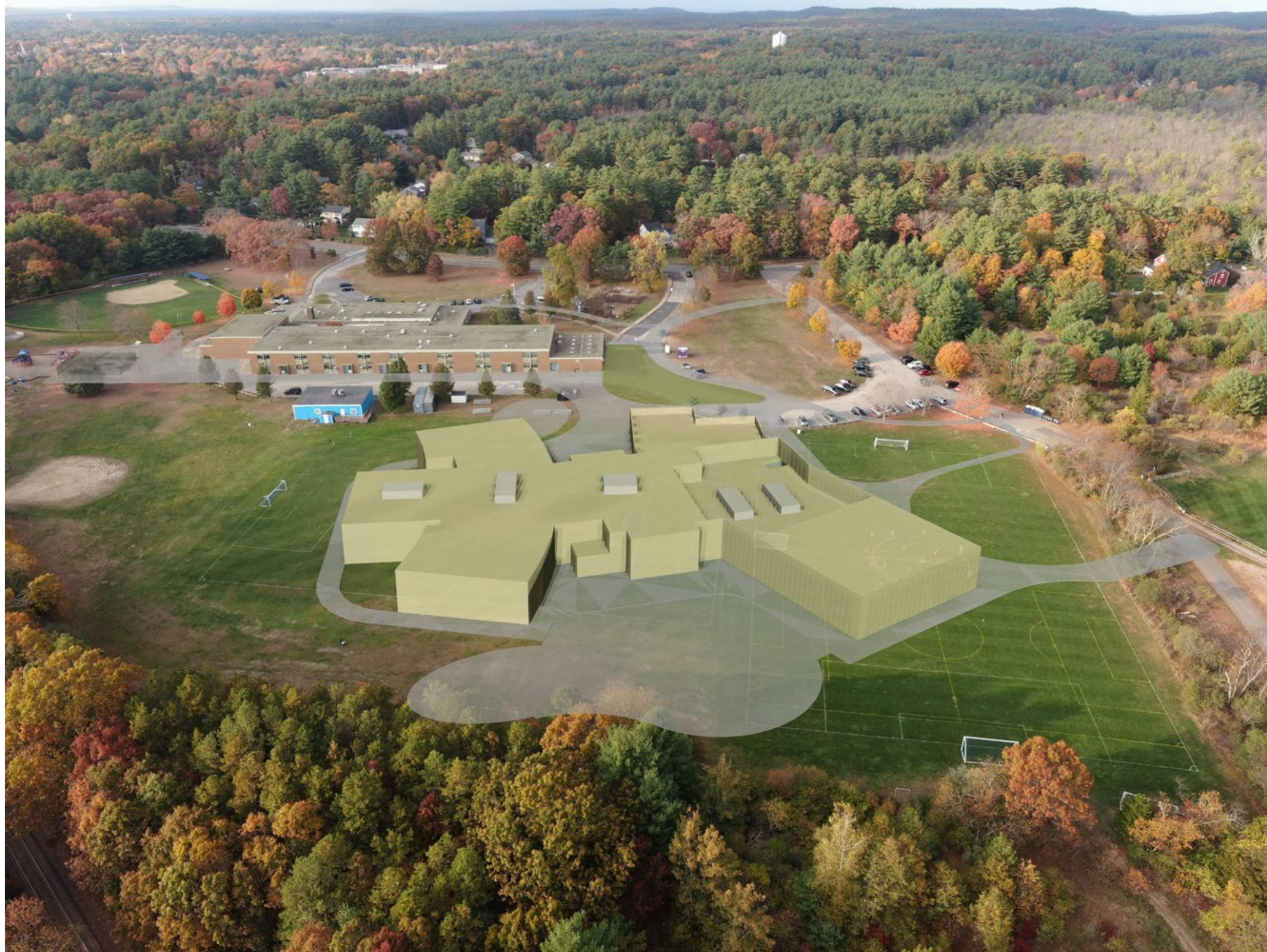
VIEW LOOKING NORTH
